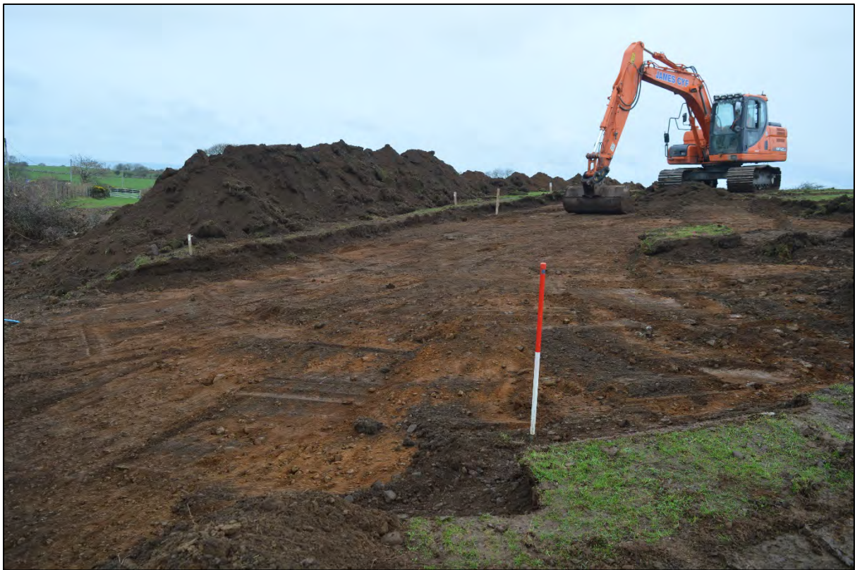
Plate 1. Stripping of topsoil for access road, 1m scale
