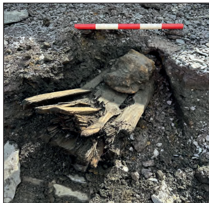
Rail sleeper with chair, looking south. 0.5m scale.
