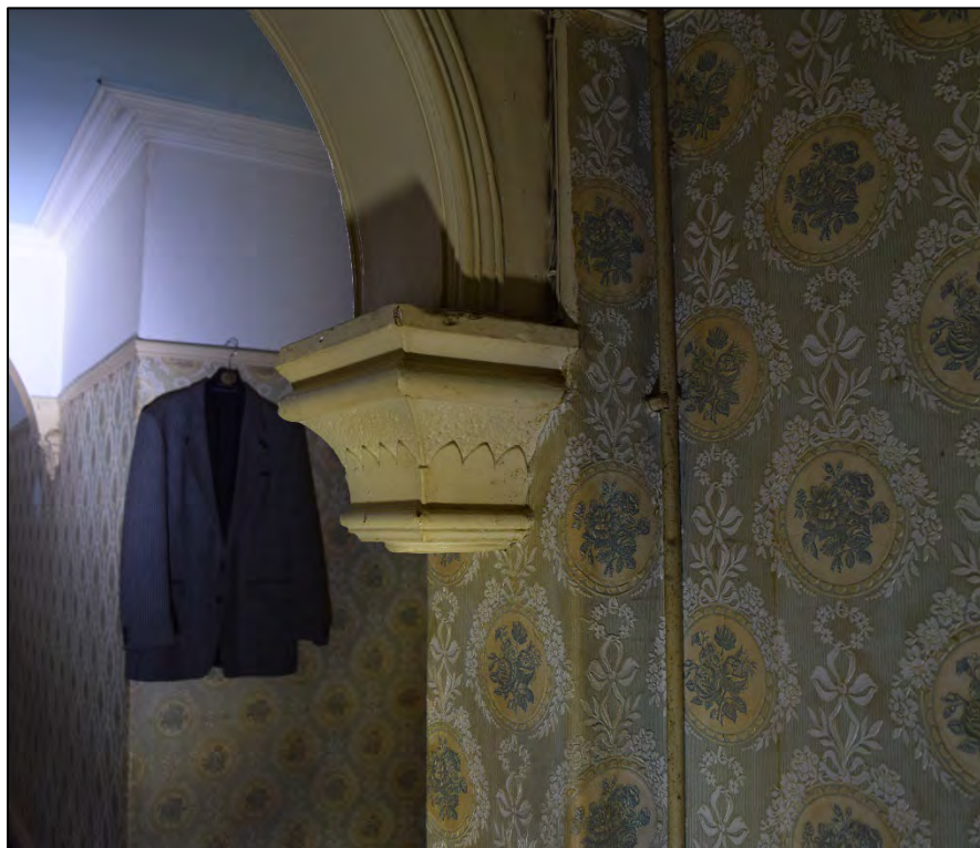
Plate 37. Corbel supporting trefoil-headed arch in hallway, Room 4, looking south-east.
