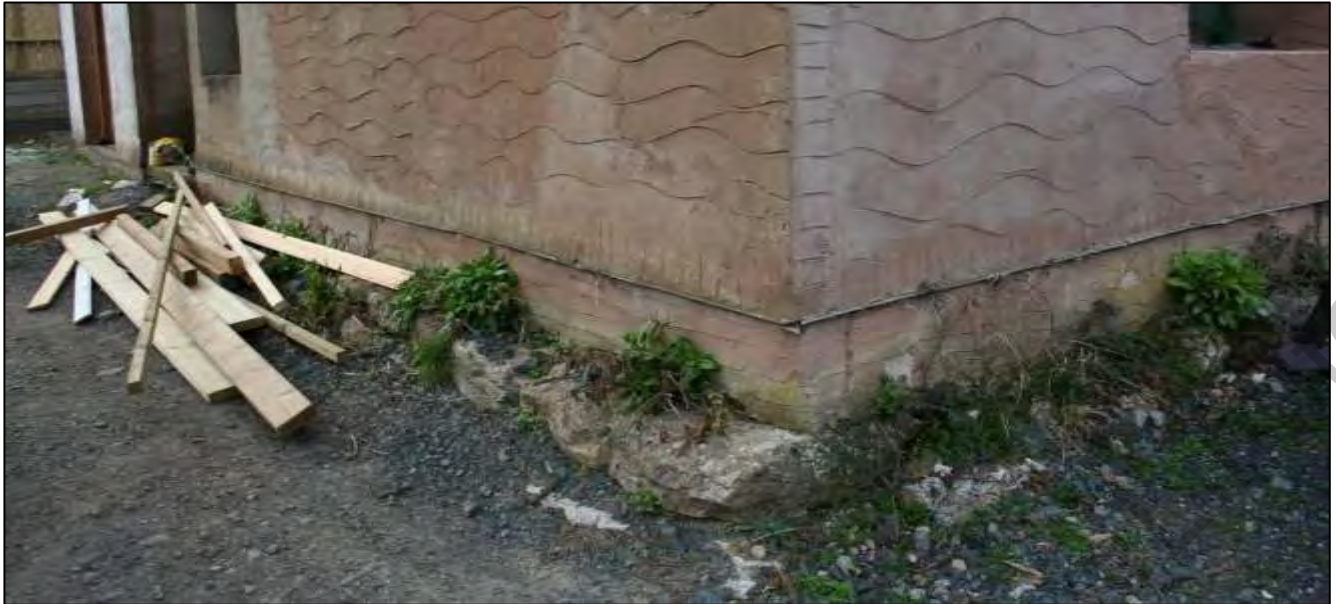
Plate 17. Exposed rubble stone foundations in south-east corner of original range, view north-west.
