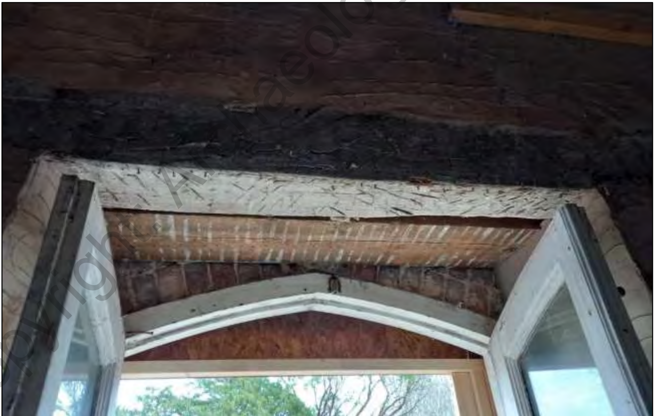
Plate 26. Lintels over front door, Room 1. View east.
