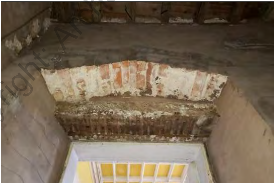
Plate 36. Brick arch and wooden lintel over door from Room 1 to Room 4, view north.
