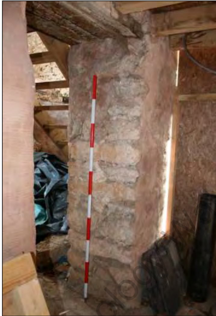
Plate 47. Doorway from Room 7 to Room 3, cut through original farmhouse wall. View south-east. Scale 2m.
