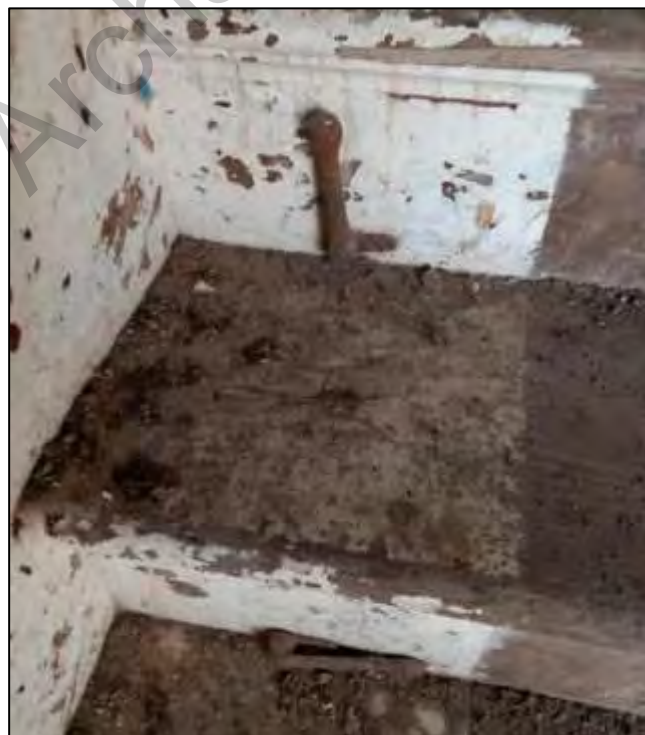
Plate 33. Detail of stair clips on risers, Room 1.
