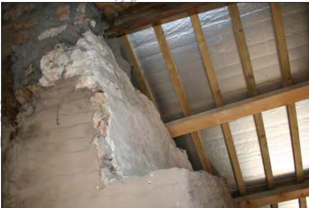
Plate 30. Surviving lime plaster to very top of chimney breast in Room 1, view east.
