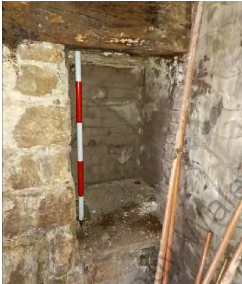
Plate 41. Alcove, possibly a former oven, to right of fireplace in Room 2. Scale 1m.
