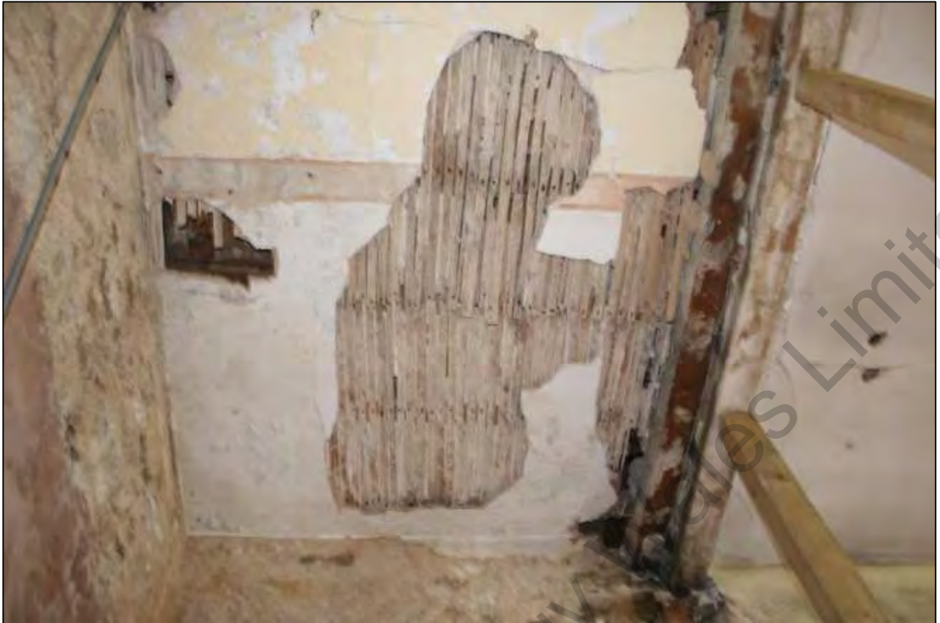
Plate 59. Ceiling at north end of Room 5 showing exposed lathes.
