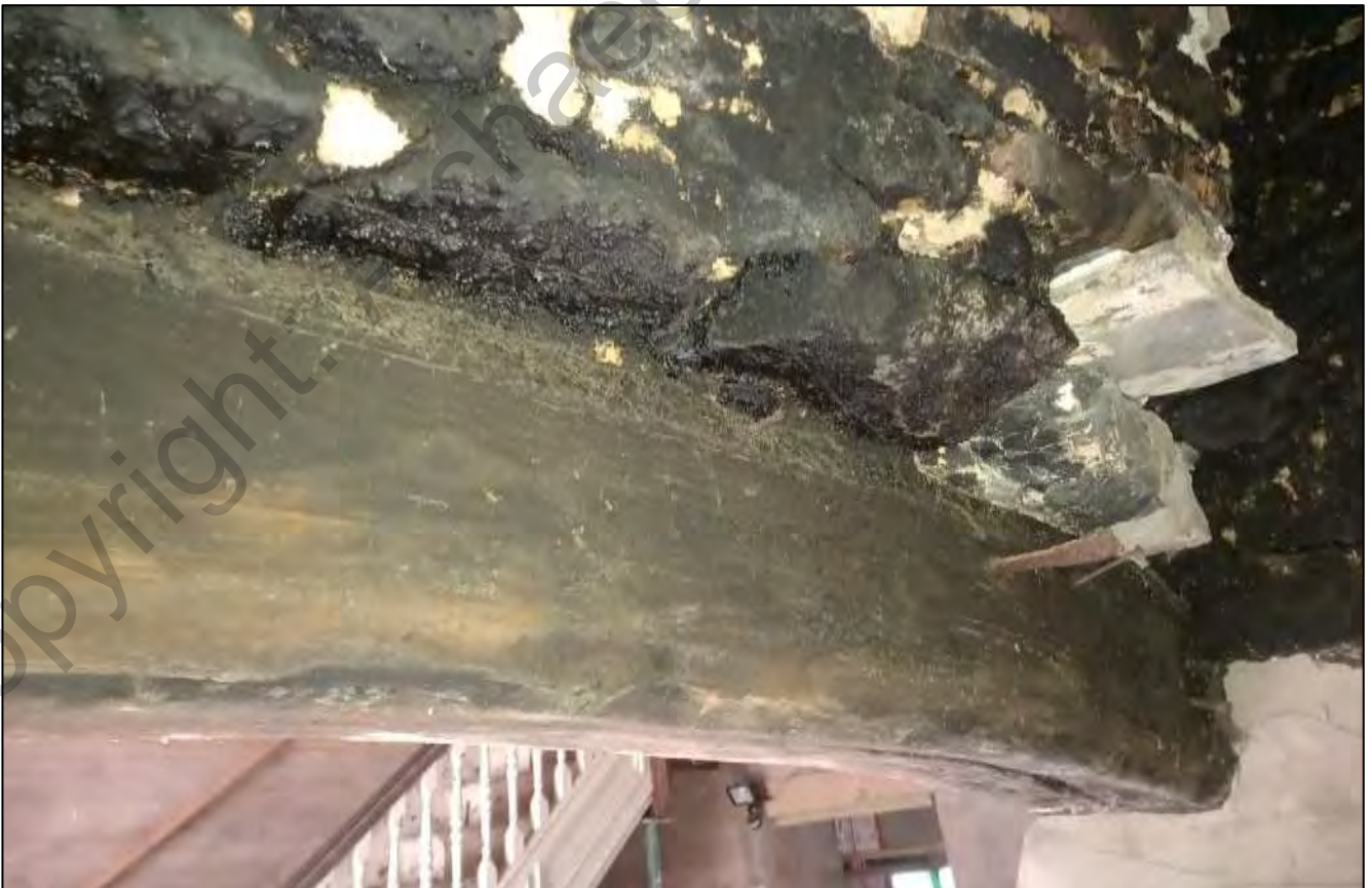
Plate 28. Interior of fireplace lintel with iron nails, view west.
