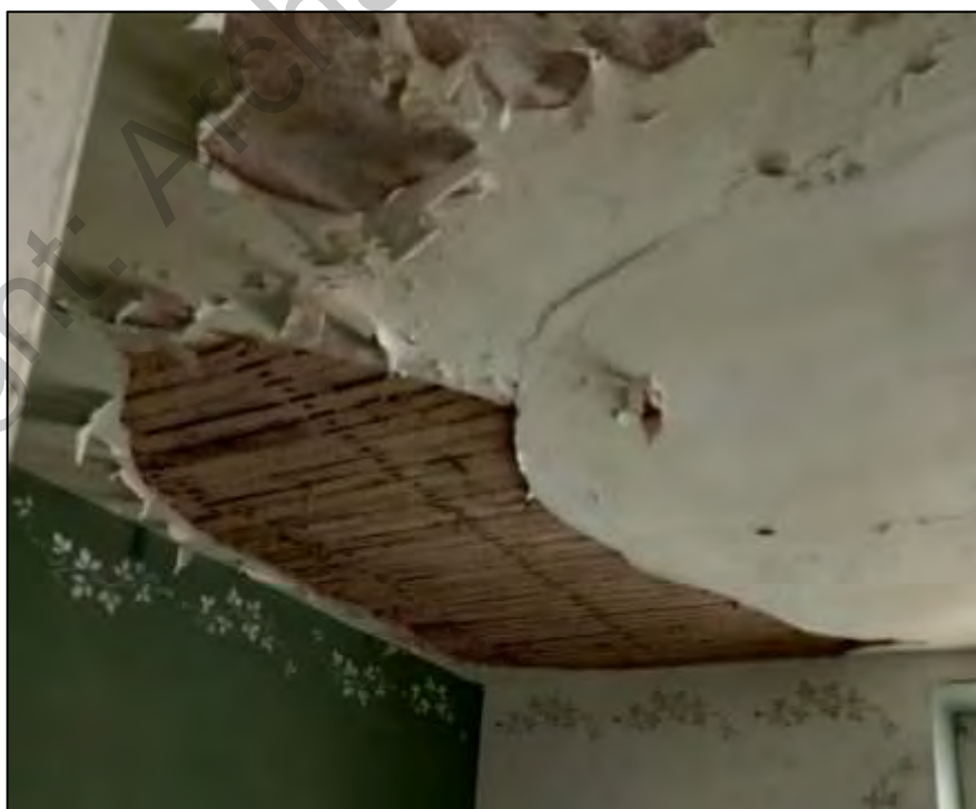
Plate 106. West end of ceiling of Room 17 with exposed lathes, view north-west.
