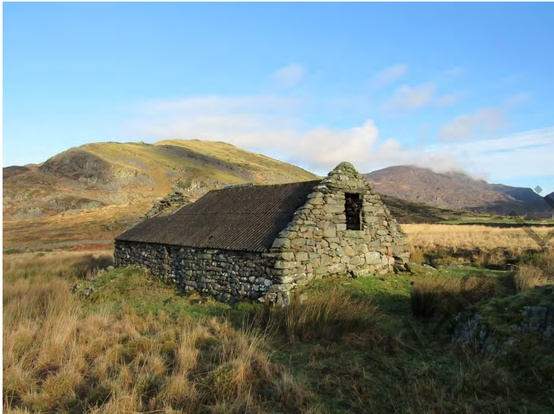
Photo 21: View of barn HW03, with blocked doorway visible in the side wall, and missing roof sections to the north. View northeast. 1m scale.
