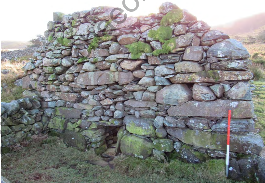
Photo 16: External face of northern gable wall of Cow Barn HW02. The central blocked doorway and sheep access visible. View south. 1m scale.
