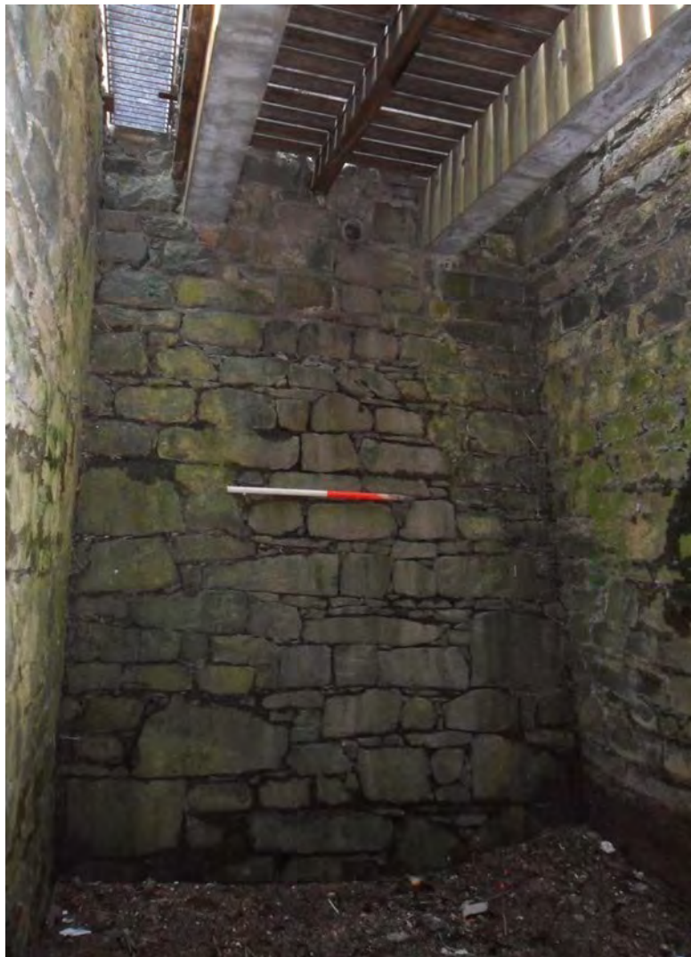
East facing elevation image of drawbridge pit
