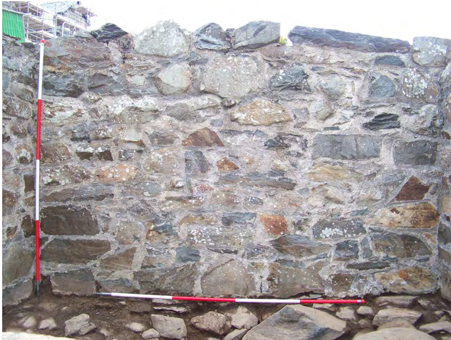
Foundation 3: Full elevation of north facing wall of pier base
