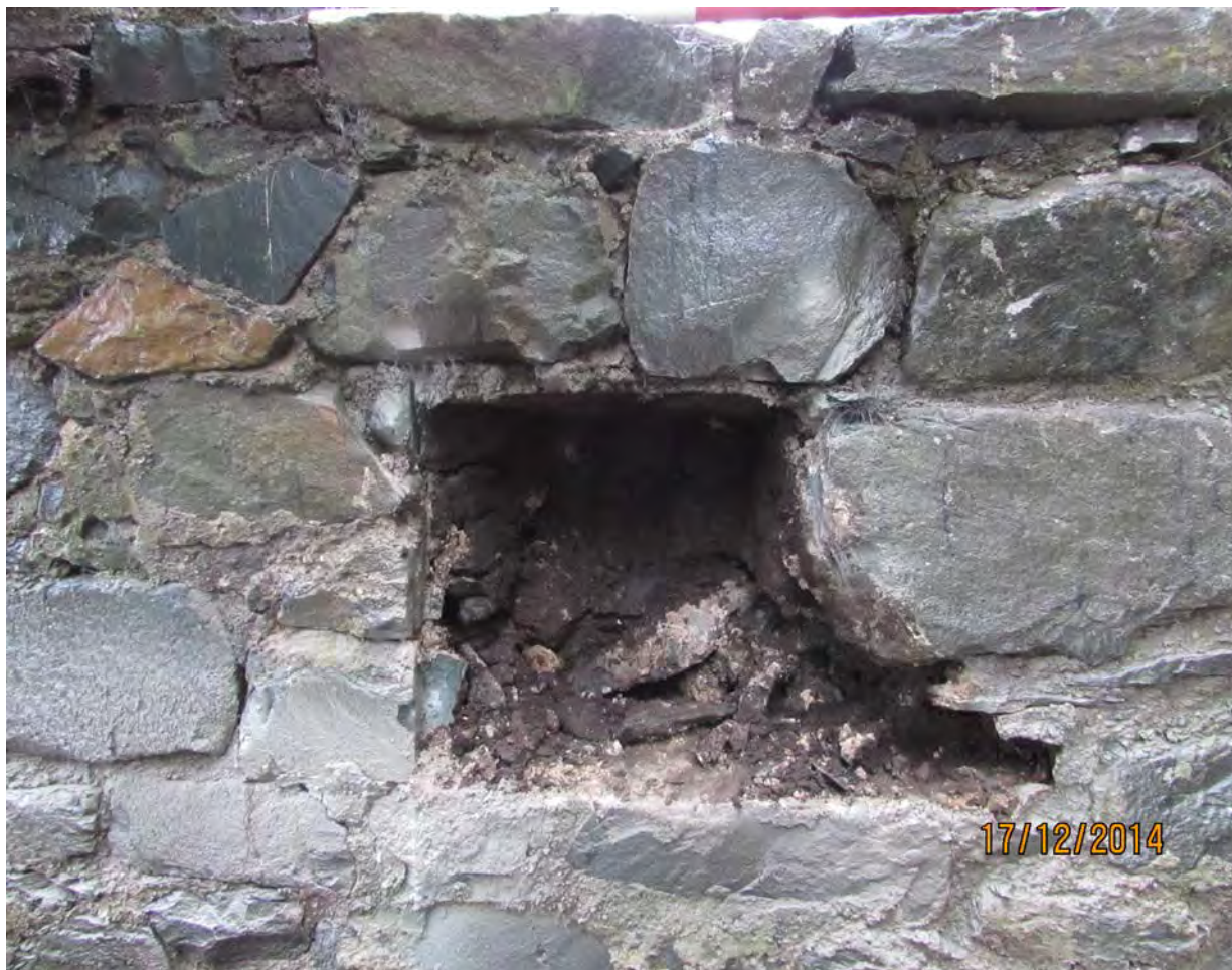
Removal of stone in upper Drawbridge pit north facing wall for new bridge socket - see fig.6 for location (looking south)
