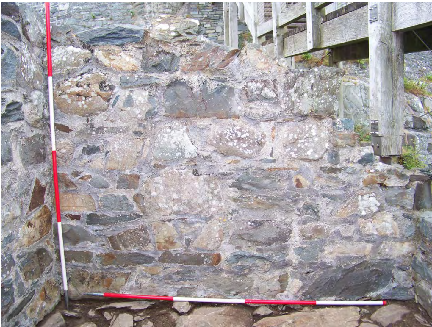
Foundation 3: Full elevation of east facing wall of pier base
