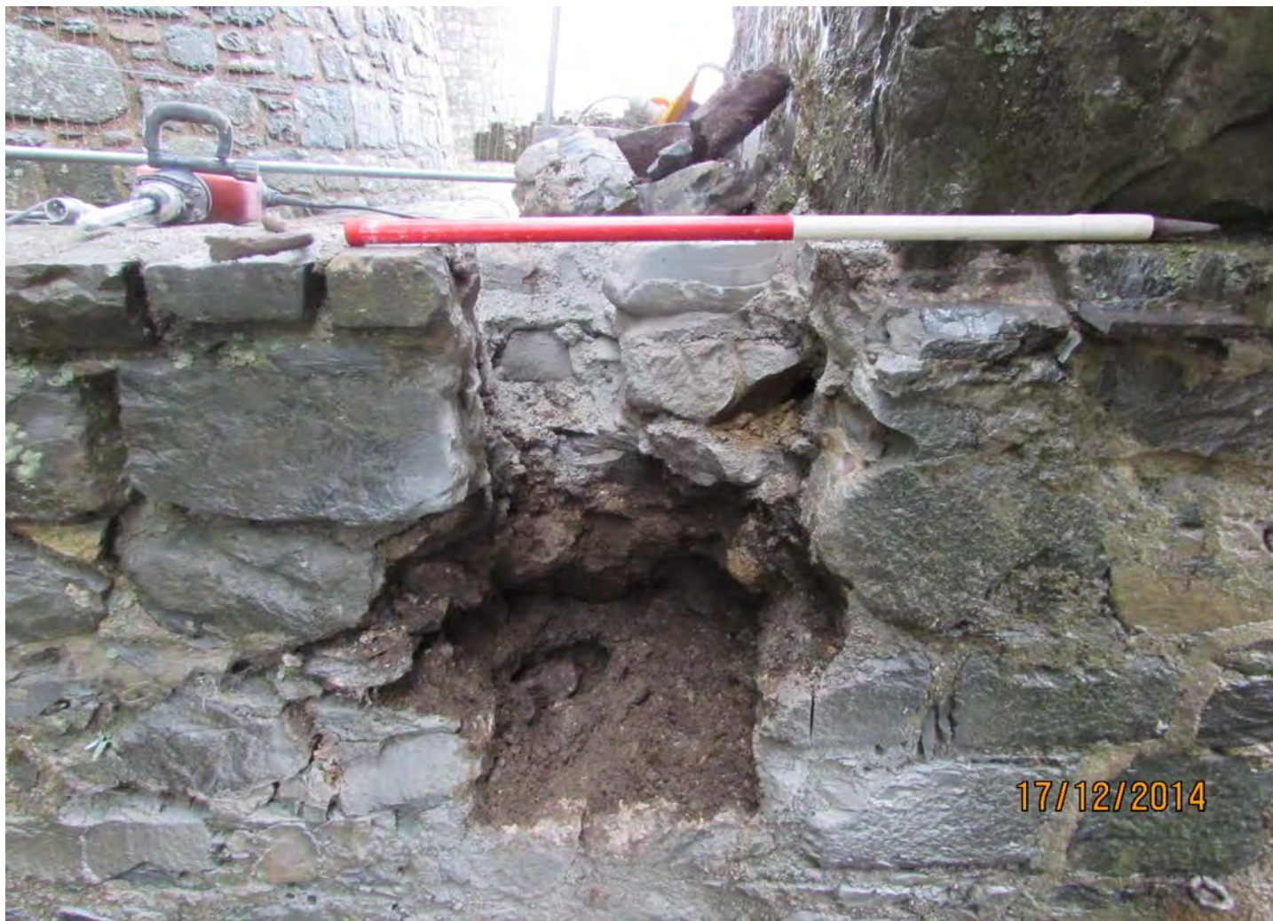
Removal of stone in upper Drawbridge pit south facing wall for new bridge socket - see fig.5 for location (looking north)
