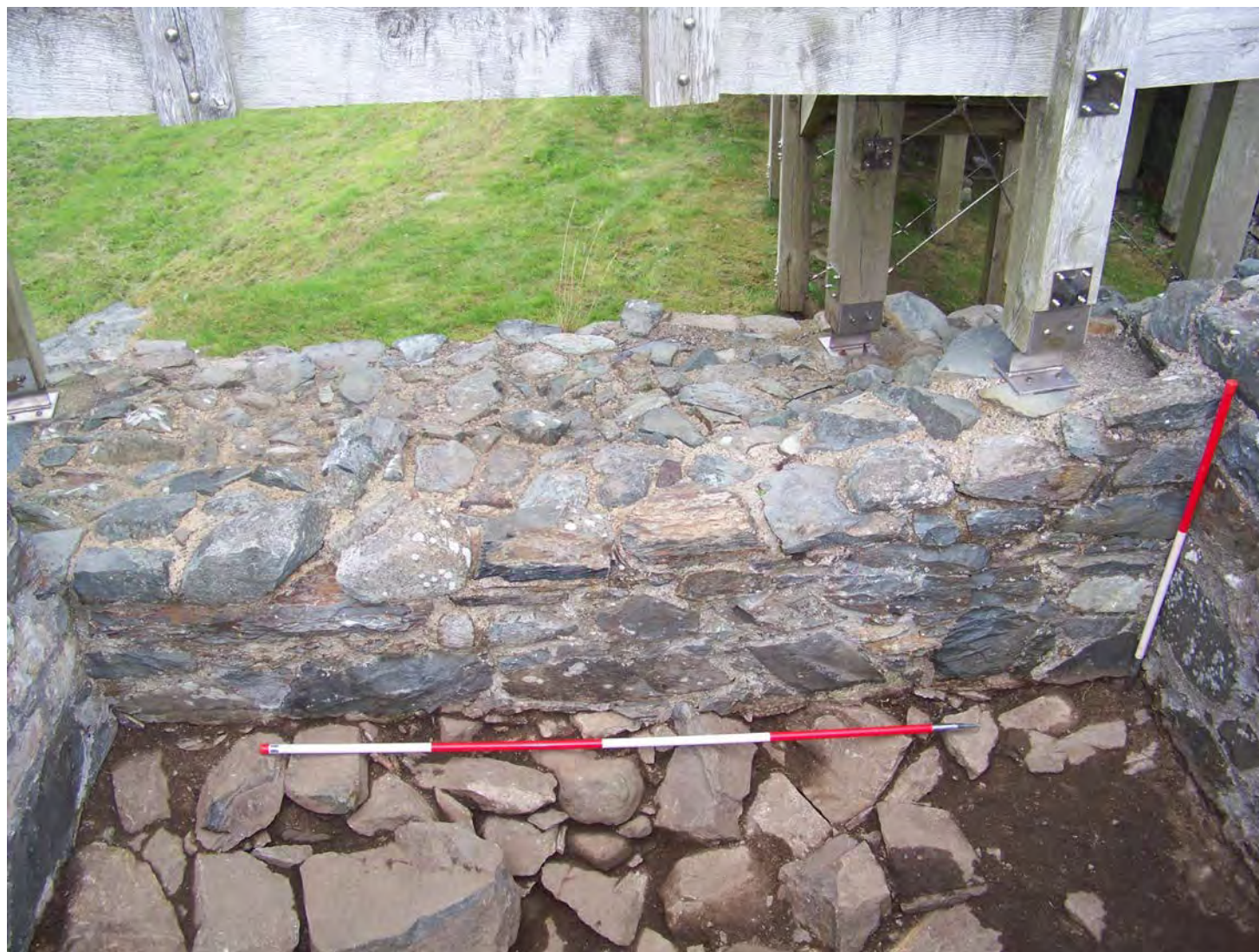
Foundation 3: Full elevation of south facing wall of pier base
