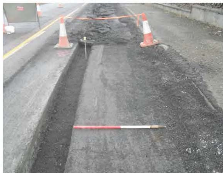
Photo 23. Section 6. Detail of pecked road surface, in advance of laying of new path surface. 1m scale. Facing North East.
