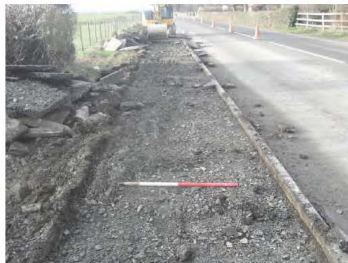
Photo 21. Underlying and pre-existing hardcore. 1m scale, Facing West.
