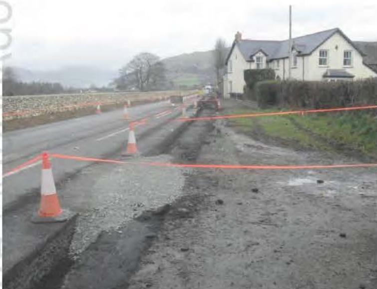
Photo 22. Section 6. General location shot after removal of top layer of existing road surface. Facing North East.
