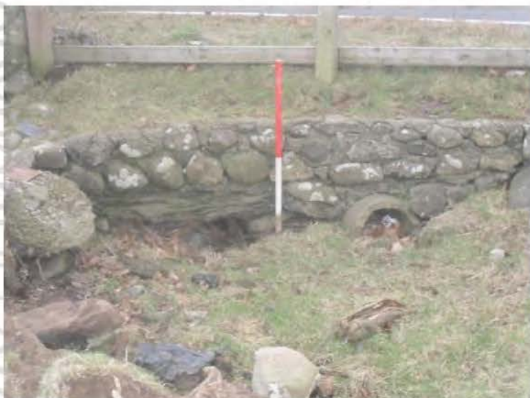
Photo 27. Section 7/8. 19 th century culvert carrying stream under present modern road. 1m scale, Facing North West.
