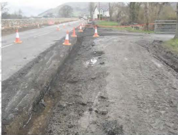
Photo 20. Section 5. Post excavation shot showing underlying and pre-existing hardcore. Facing North East.
