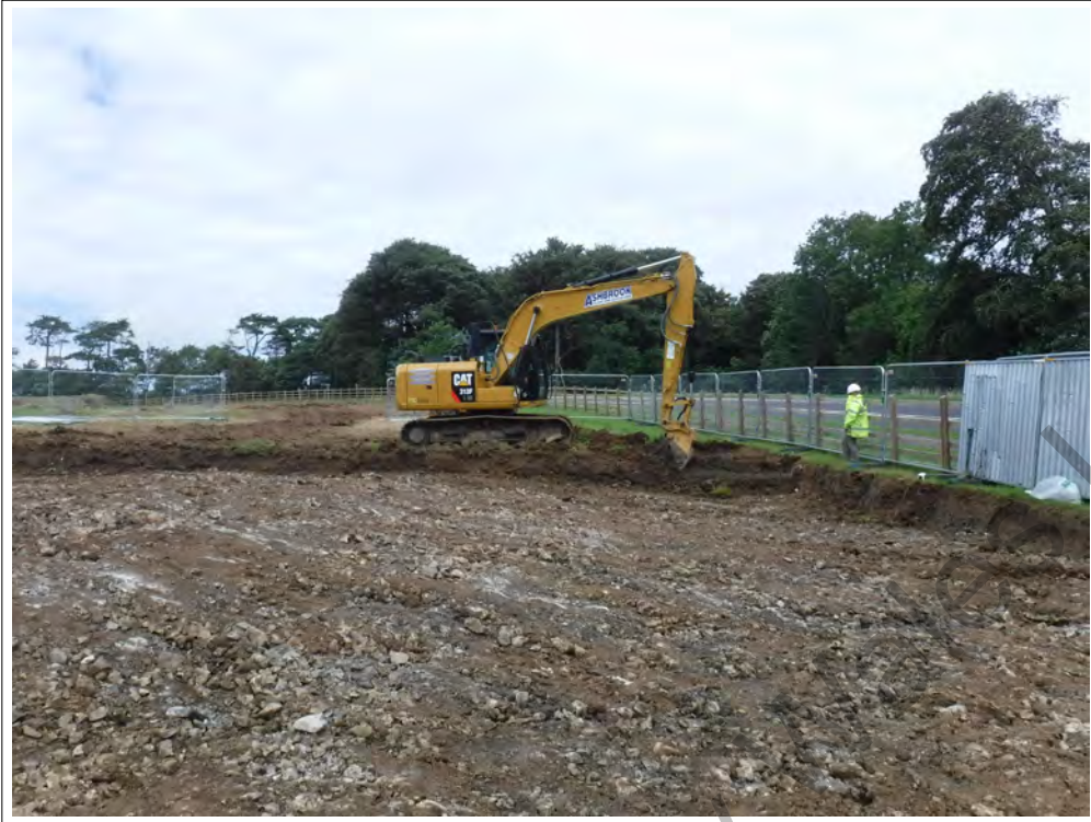
Plate 1. Working shot of topsoil stripping. Looking NE
