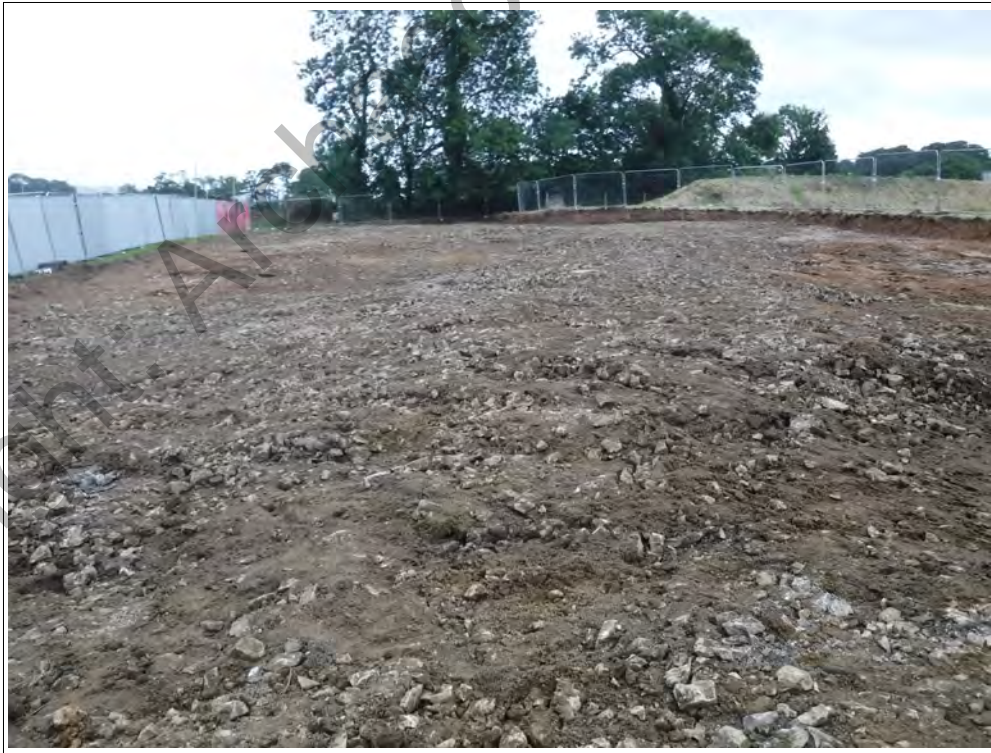
Plate 2. Stripping of site completed. Looking SW
