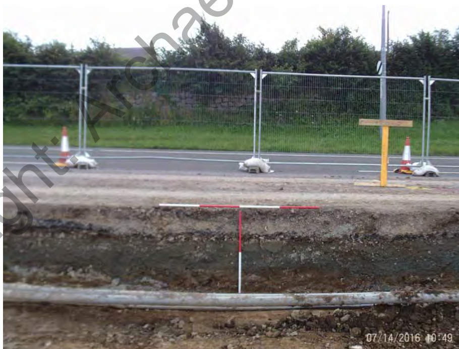
Plate 2. West facing section of site strip excavation, with services and road makeup
