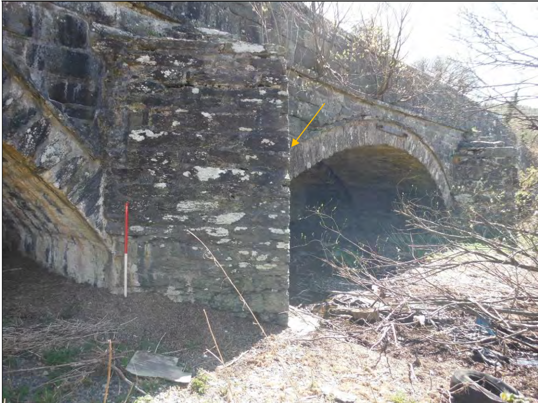
Photograph 14: Pont Mwnwgl-y-llyn North pier, west cut water.
