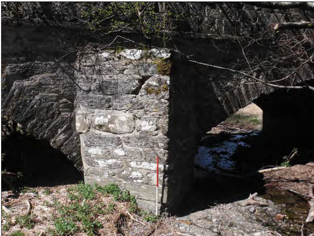
Photograph 22: South pier, east cutwater.
