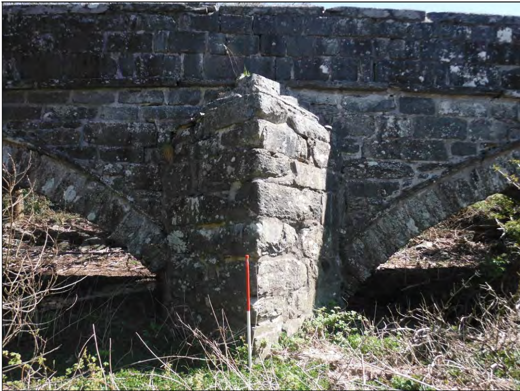
Photograph 21: Pont Mwnwgl-y-llyn south pier, west cutwater.
