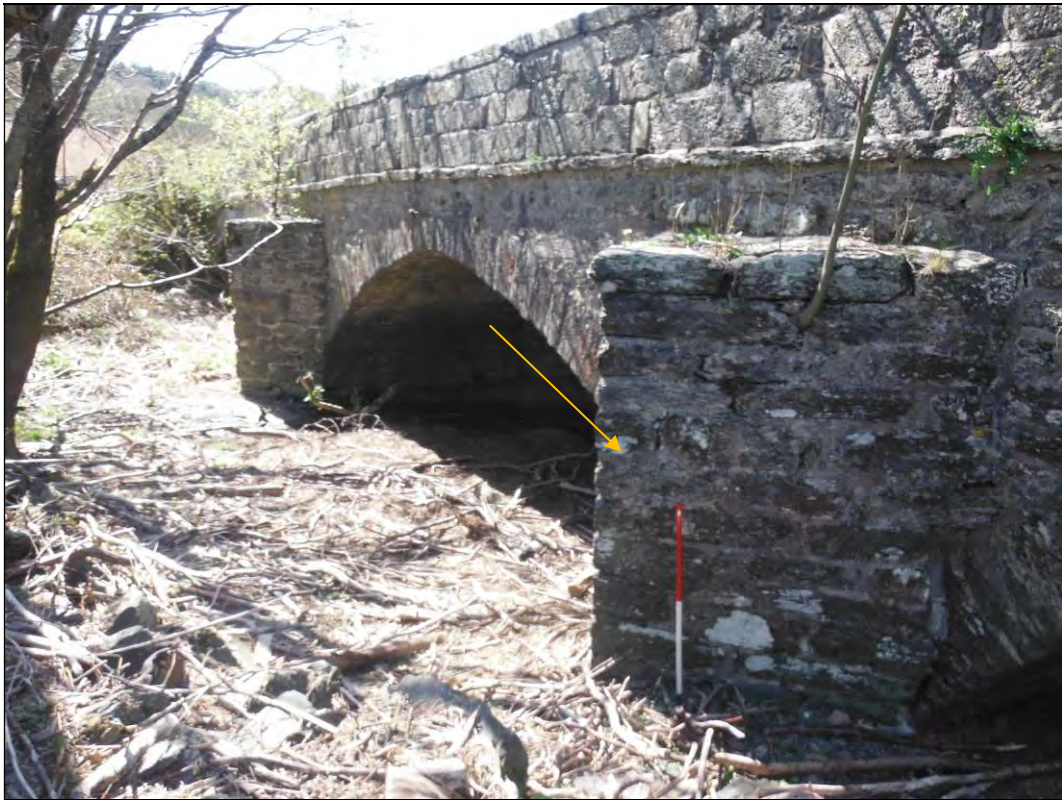
Photograph 15: North pier, east cut water.
