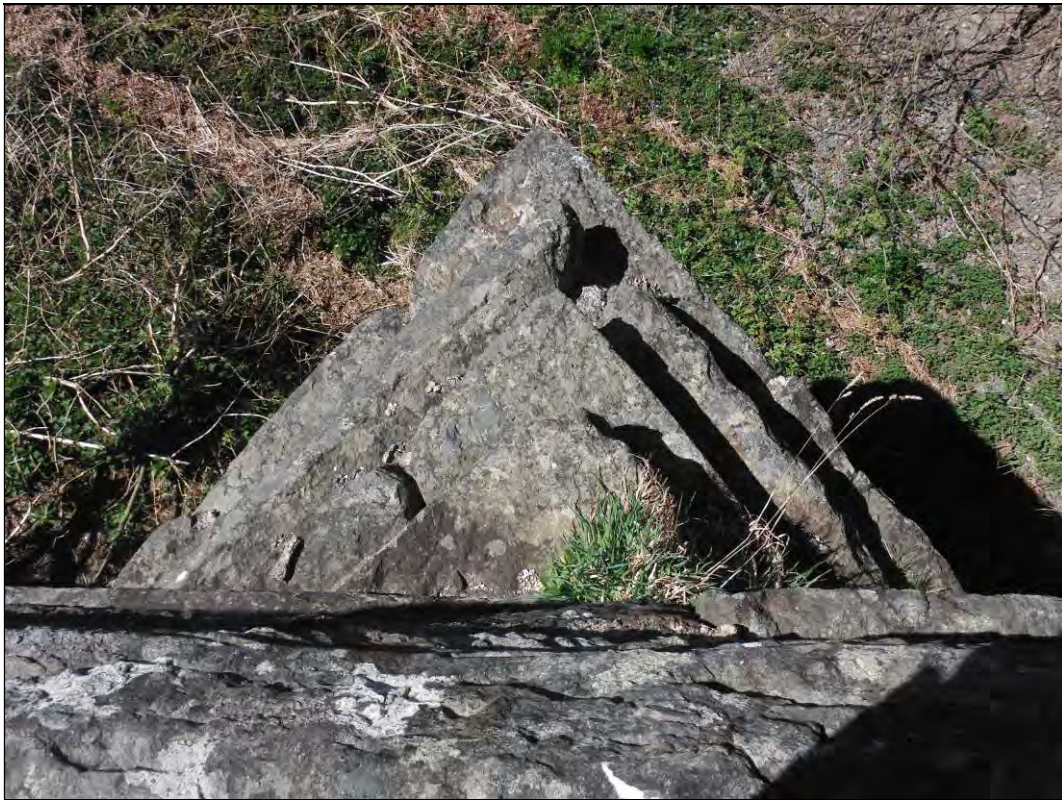
Photograph 23: South pier, cap of west cutwater.
