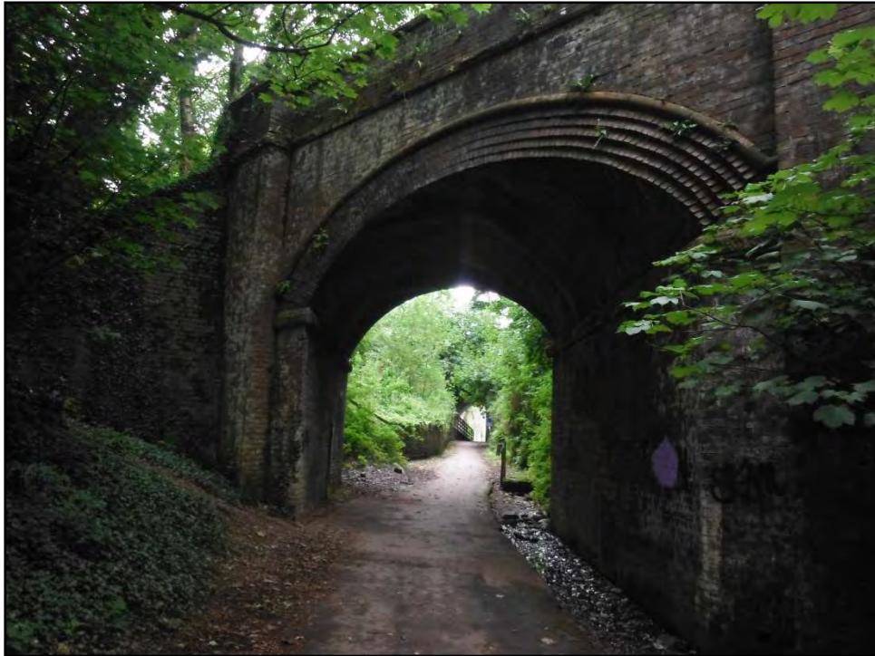
Photograph 17: View east towards the brick-built single-arch skew bridge (HER 65561) built to carry the Penrhyn Quarry Railway over the Bethesda branch of the London & North Western Railway (now the Ogwen Trail). The Tal Gae road bridge is in the distance.
