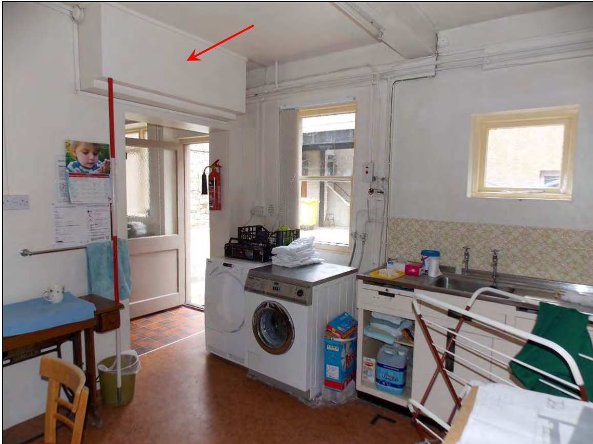
Plate 47: Truncated chimney breast (arrow), looking north-east (scale 2m).
