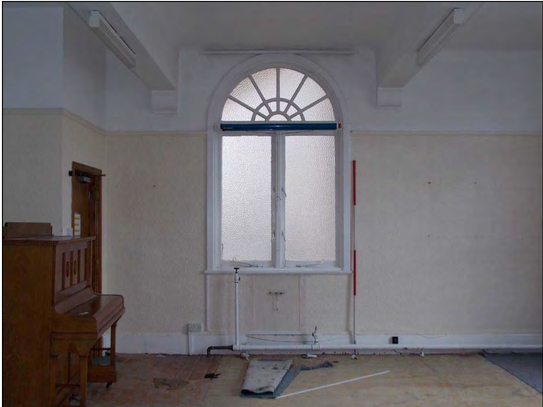
Plate 14: Detail of window opening with semi-circular arched head, looking east (scale 2m).
