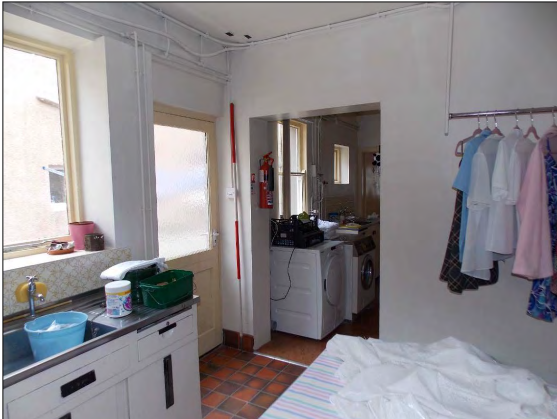
Plate 46: Inserted doorway within the dividing wall of the laundry, looking south-east (scale 2m).
