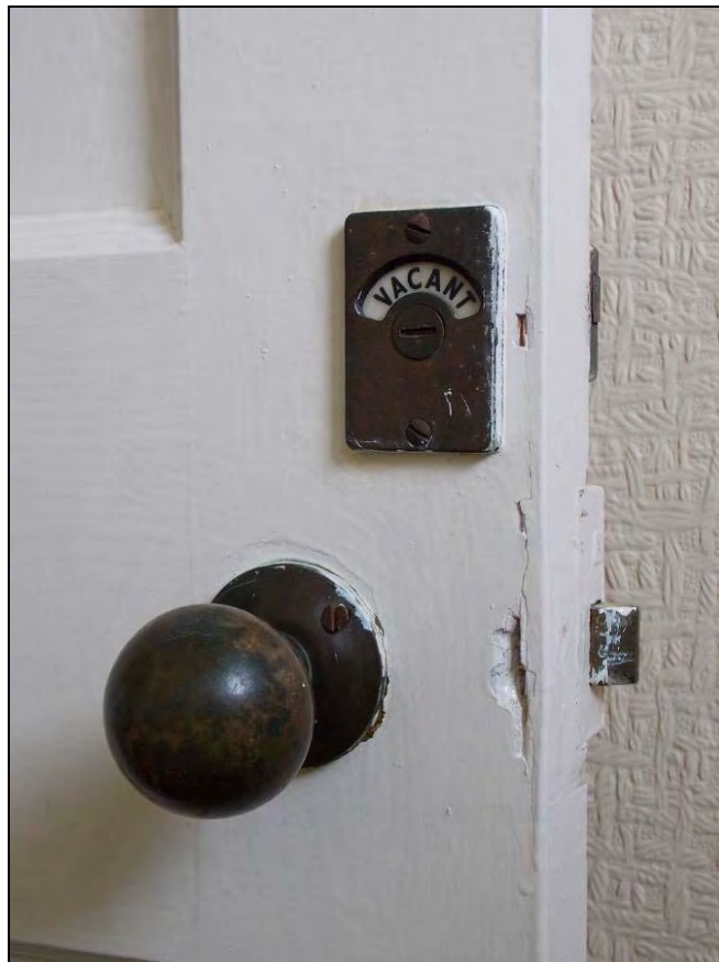
Plate 25: Detail of brass door lock
