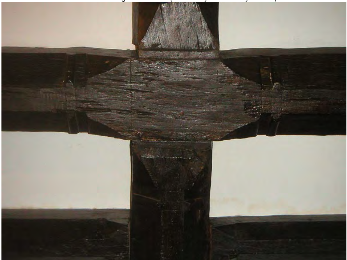
Plate 4 Ceiling to main hall (tertiary beams)
