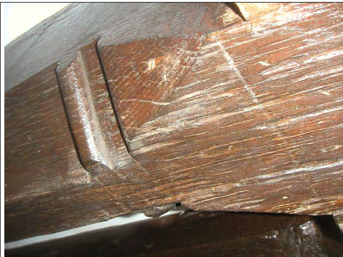
Plate 5 Detail of stop on tertiary beam
