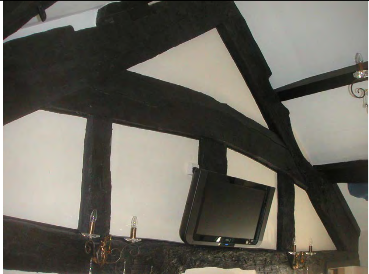
Plate 3 Truss 2 (W face)
