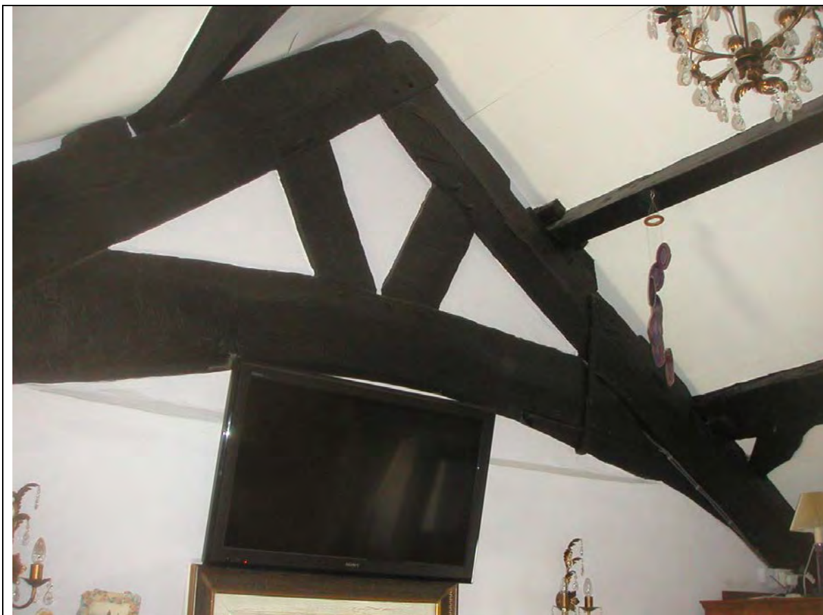
Plate 1 Truss 1 (E face)
