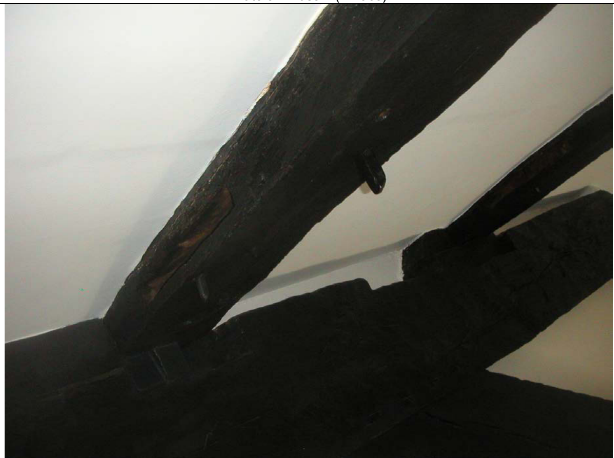
Plate 4 Truss 2 (slots and cut-outs for wind-braces)
