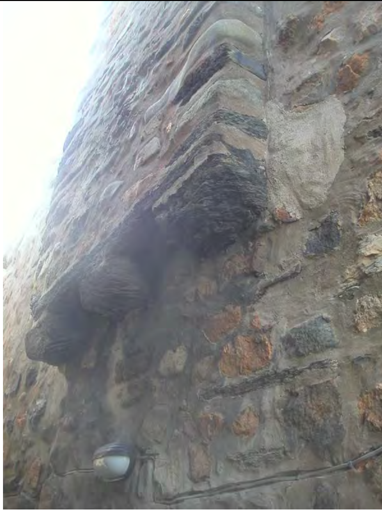
Plate 5 corbelled chimney at E gable
