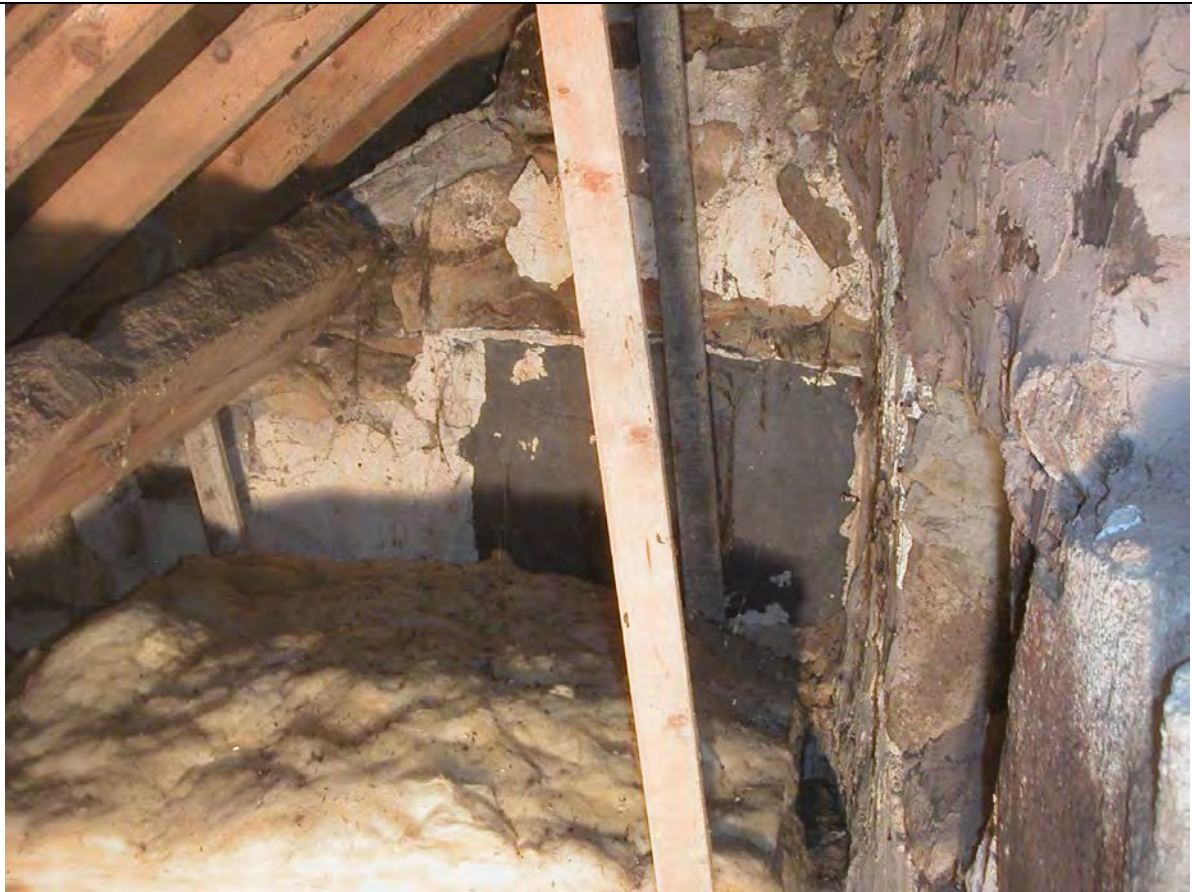
Plate 12 Possible blocked window in north gable
