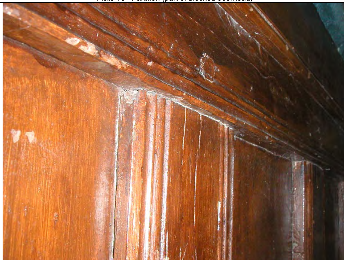
Plate 11 Partition (detail of post and head mouldings)
