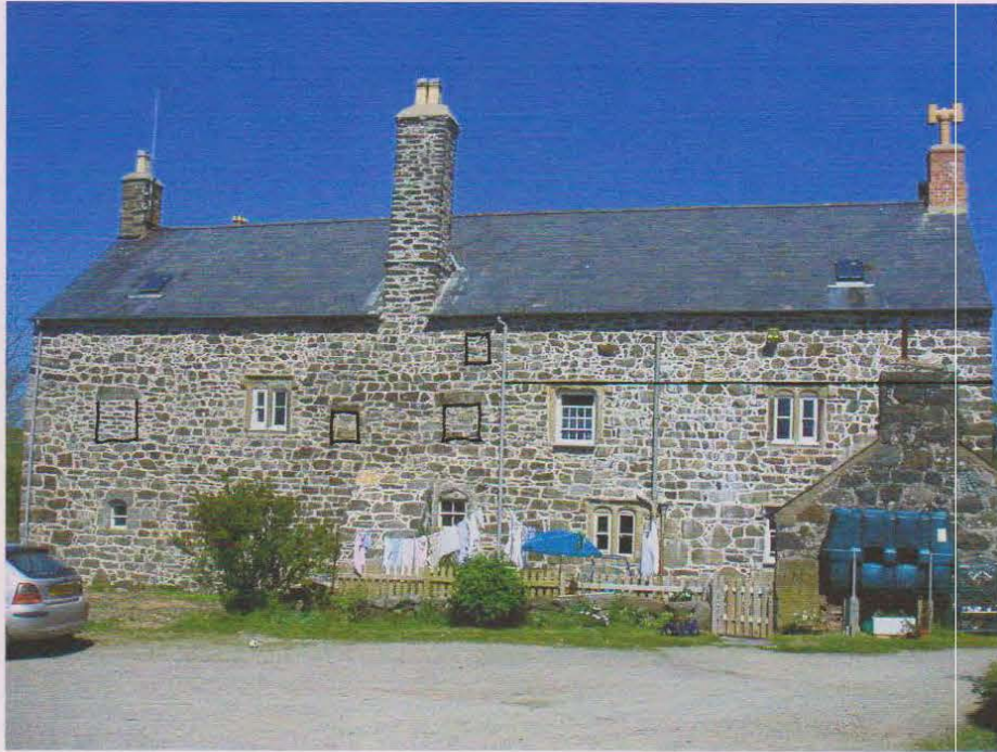
South elevation, marked up to show more clearly the blocked windows and the horizontal line at window head level at the east end
