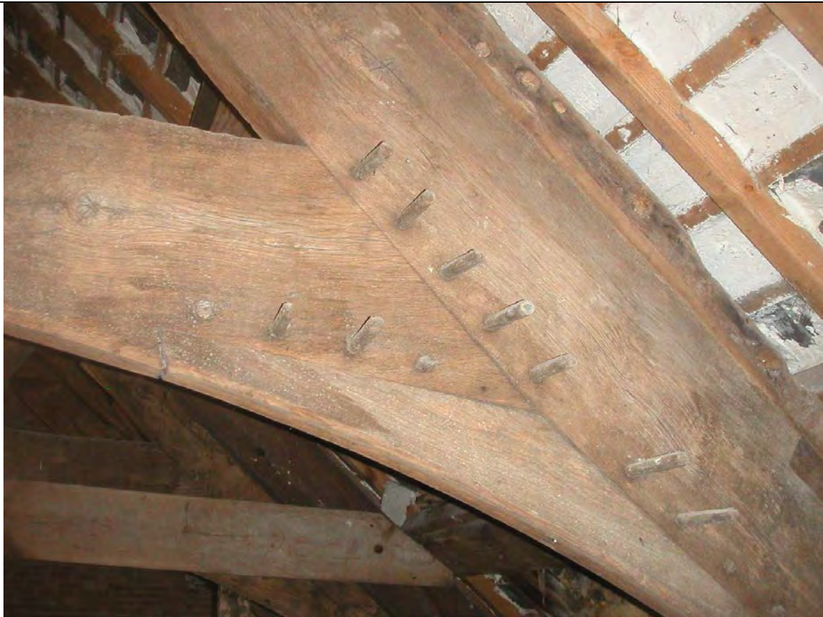
Plate 9 Truss T3, from west, showing pegged joint
