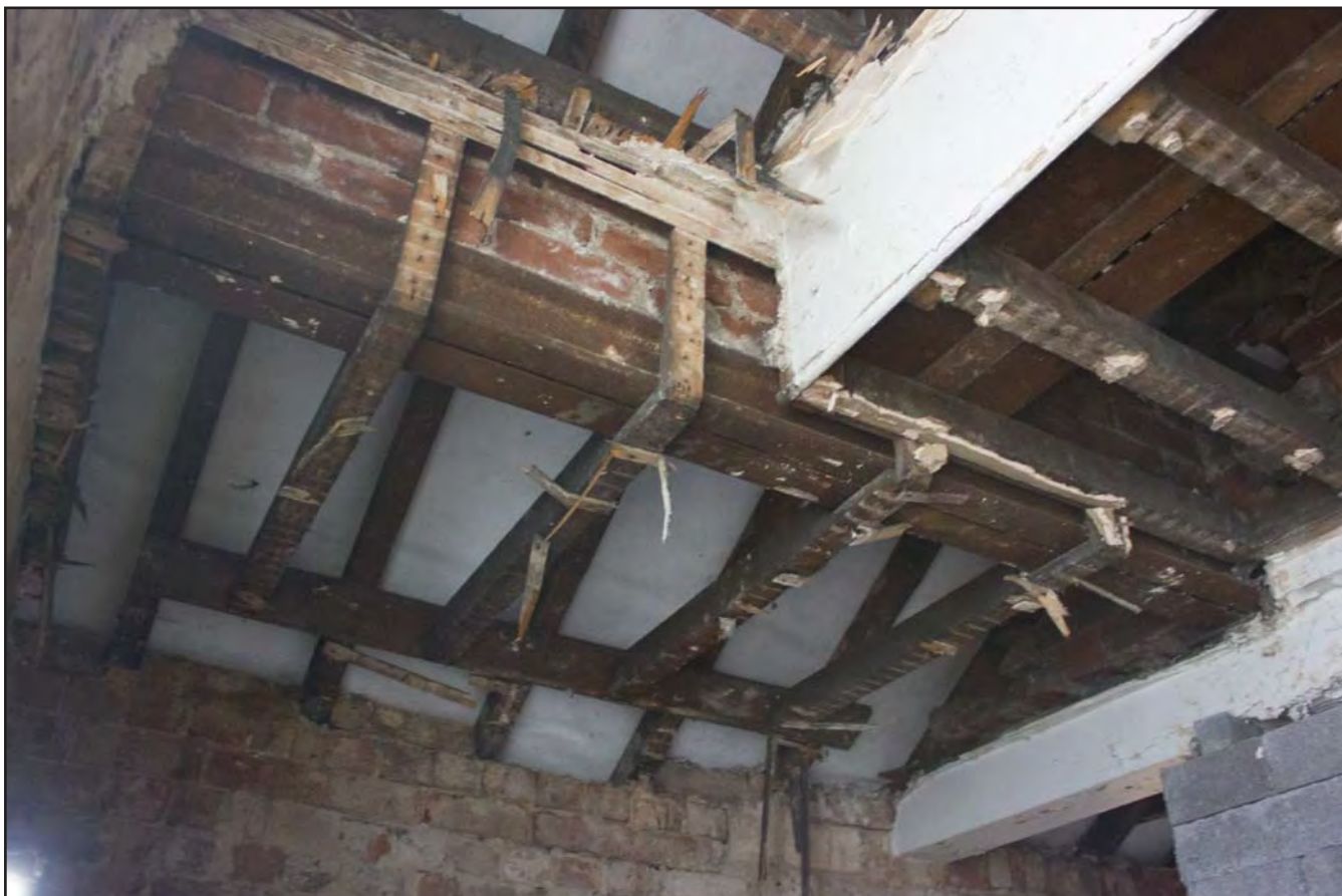
Plate 76: Railway Sleeper in exposed ceiling of Caretaker's Office the Main School Building, Ysgol Maelgwn, Llandudno, from the northeast - scale 1m
