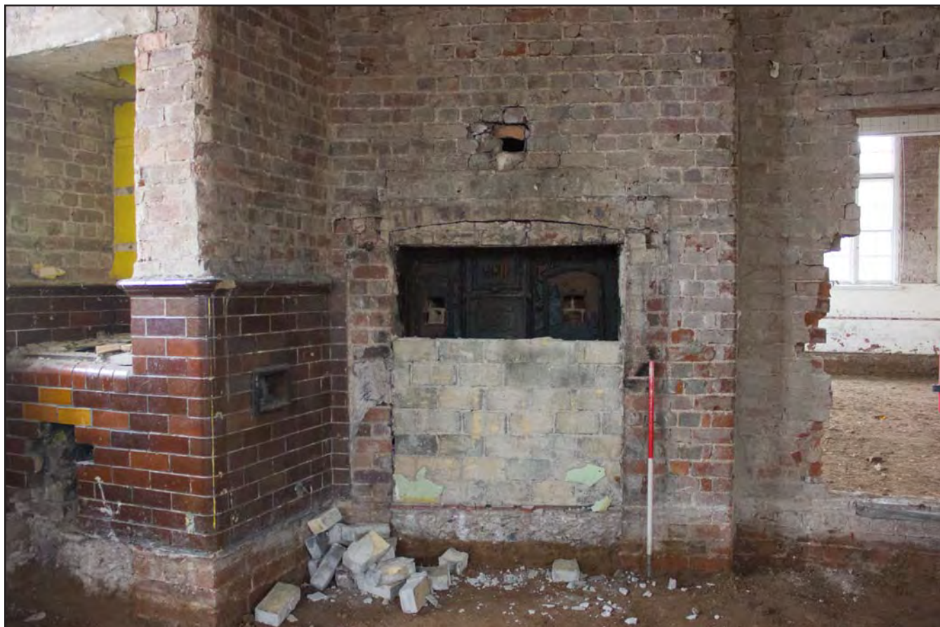
Plate 113: Blocked up stove within the Classroom Building, Ysgol Maelgwn, Llandudno, from the northeast - scale 1m
