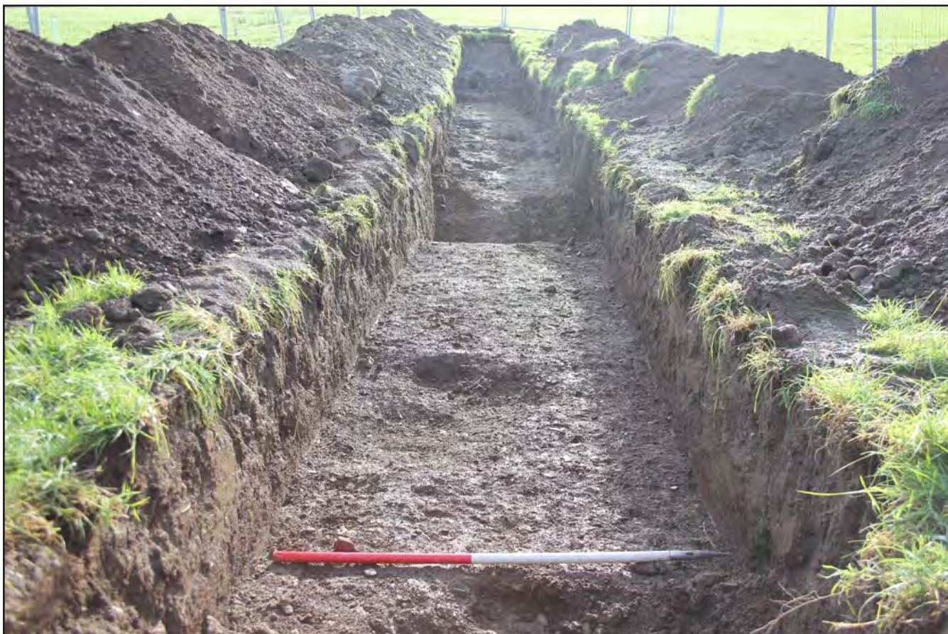
Plate 59: Test pit within Field H to locate water main - from the southwest - scale 1m
