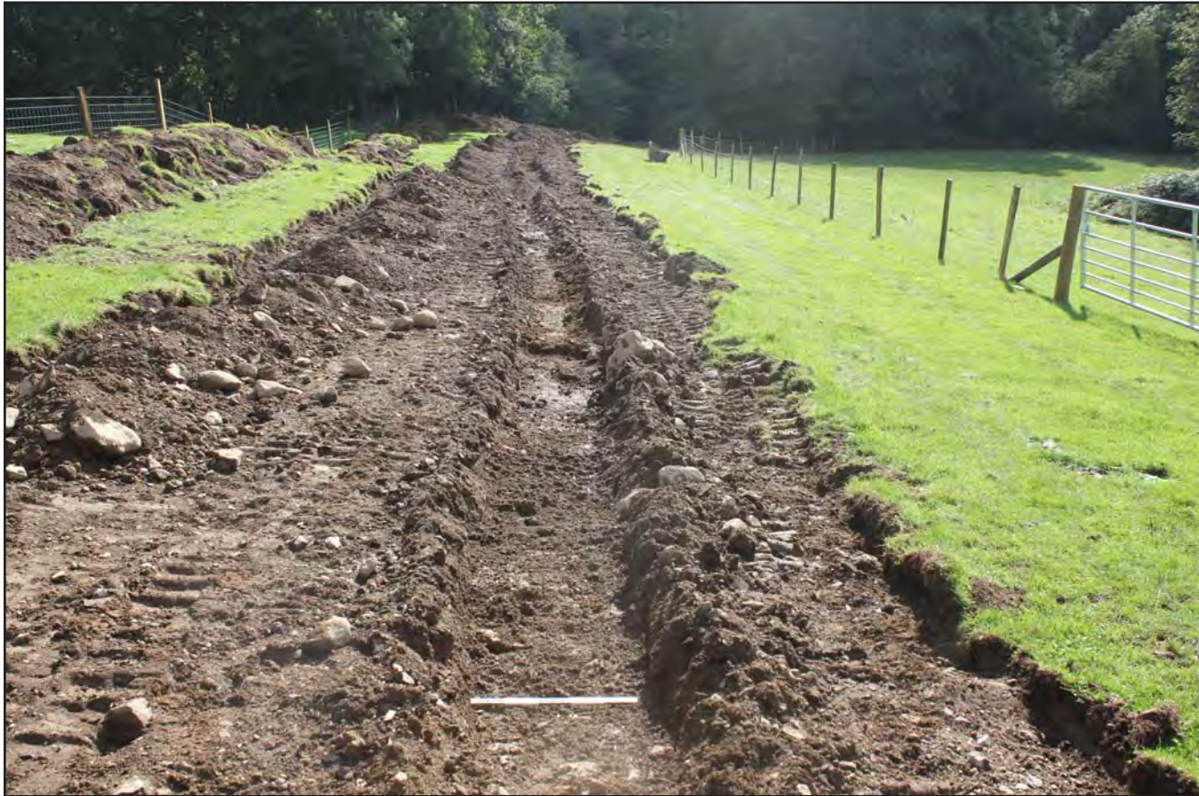
Plate 34: Pipe trench within Field G (top of slope) - Route 1 - from the north - scale 0.5m
