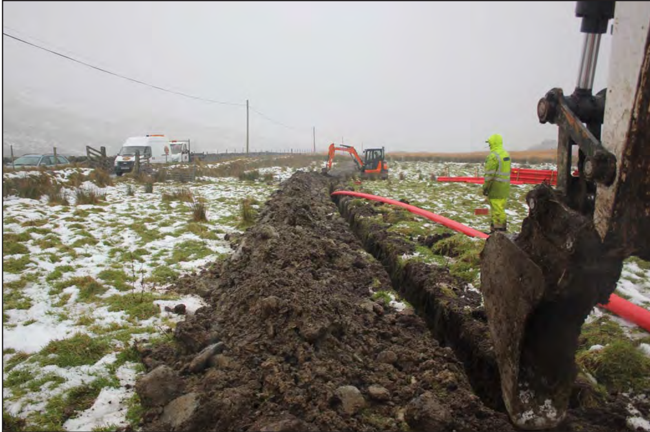
Plate 05: Post-excavation of Cable trench - near Pitt's Head and reception pit for directional drill - from the northwest - scale 1m
