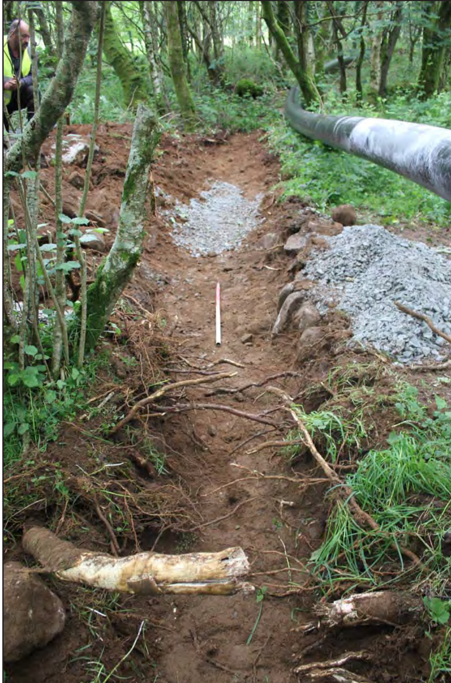
Plate 11: Penstock trench at location 2 across trackway feature 50 - from south - scale 1m
