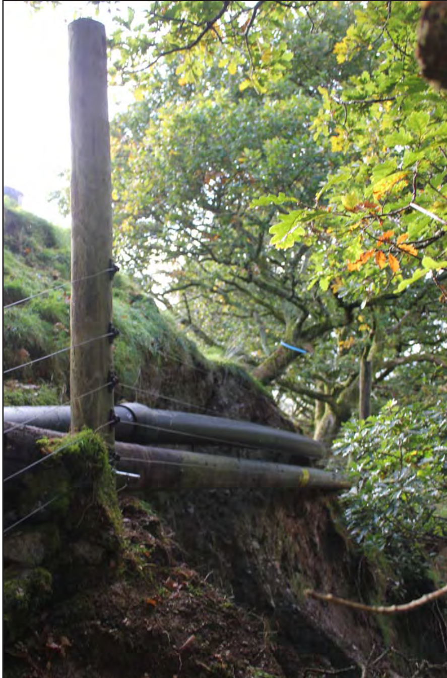
Plate 28: Completed works with pipe routed around the SAM erosion scar - no scale
