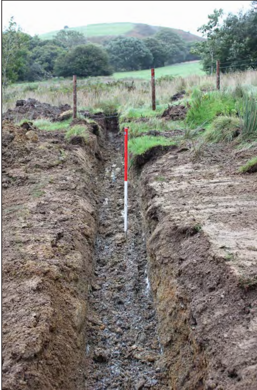
Plate 13: Penstock trench at CH500 looking South - 1m scale
