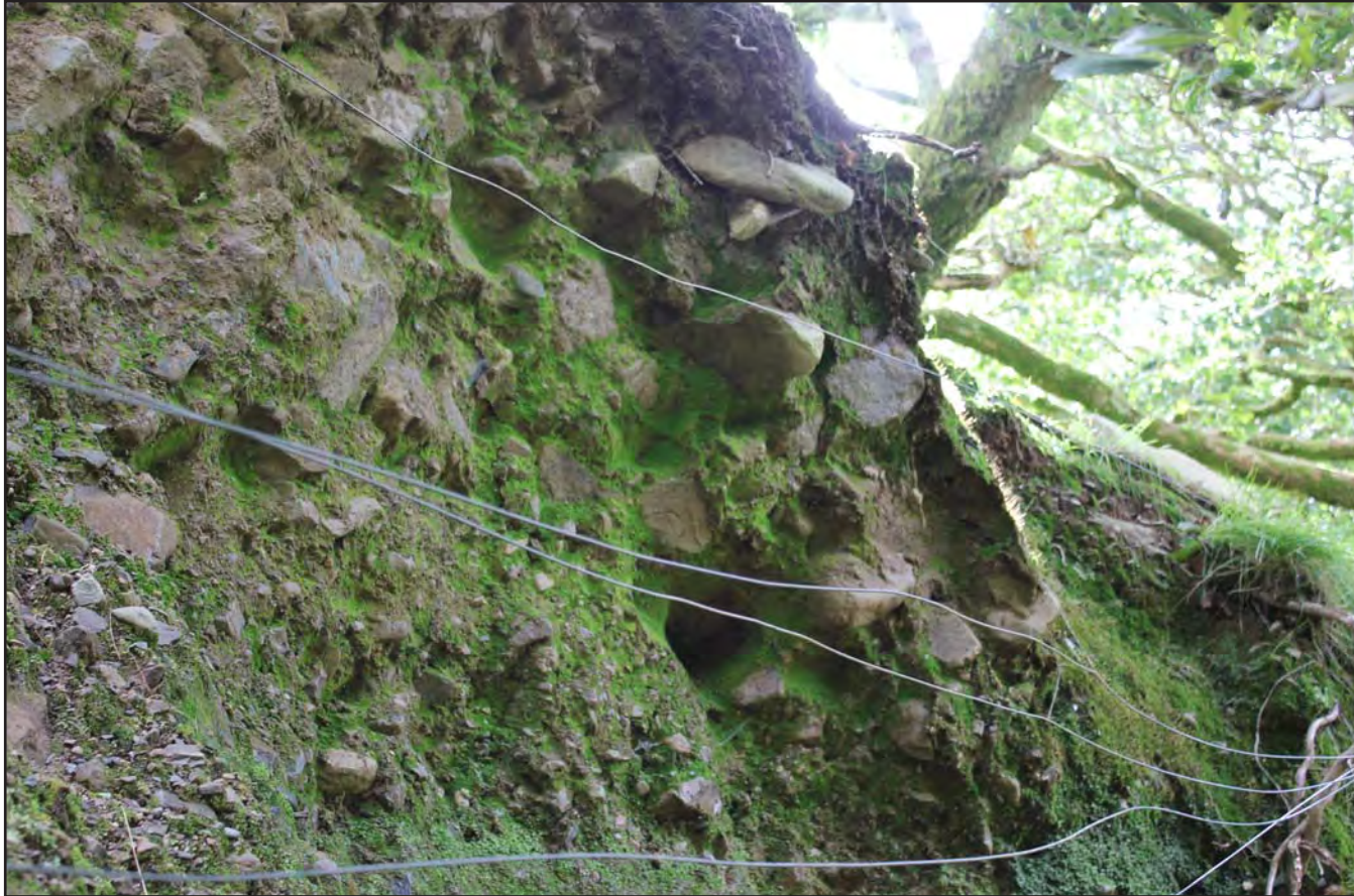
Plate 23: Close up of revetment stones revealed by the erosion scar (facing northwest) - no scale
