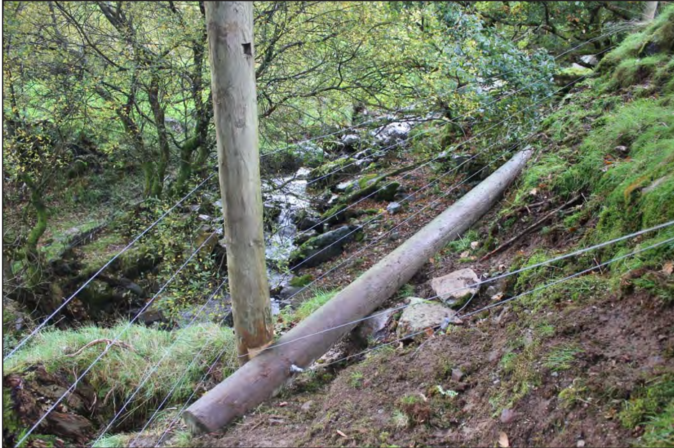
Plate 24: Mitigation response routing the pipe around the SAM erosion scar (Afon Drws y Coed to North) - no scale
