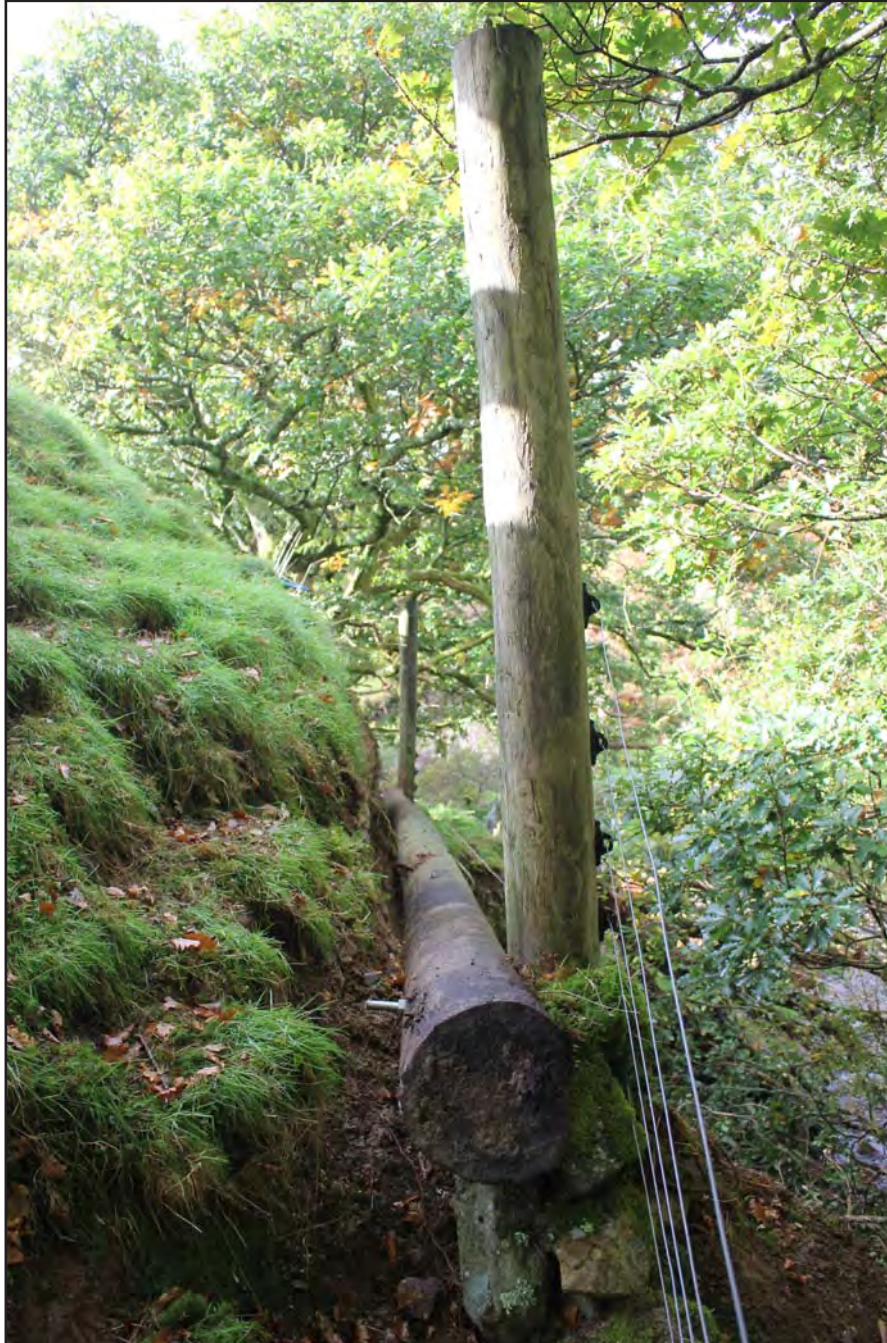
Plate 26: Mitigation response from the Northeast (upright timbers support the weight) - no scale
