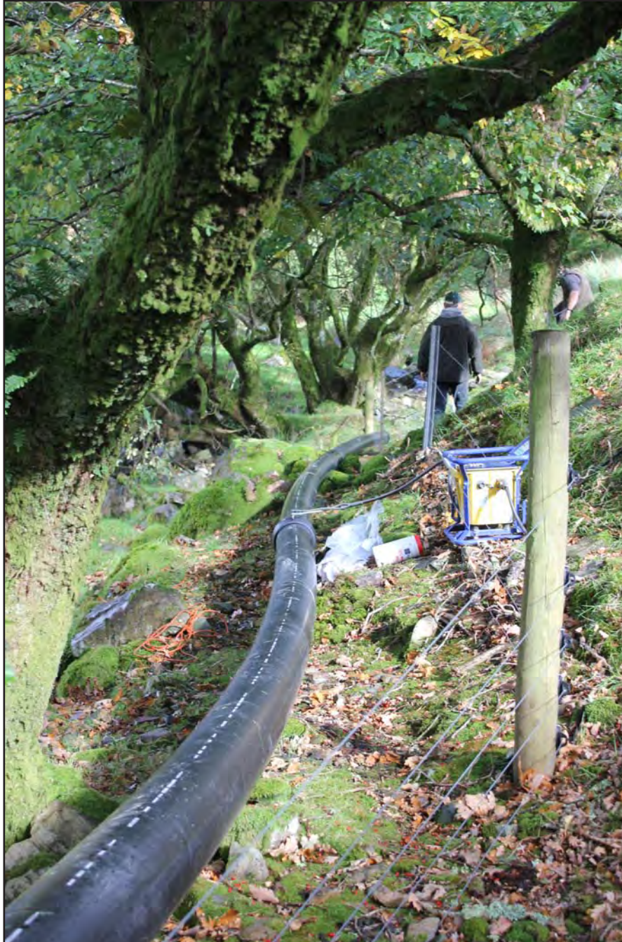
Plate 34: Example of pipe welding in the river gorge (shot facing Northeast) - no scale
