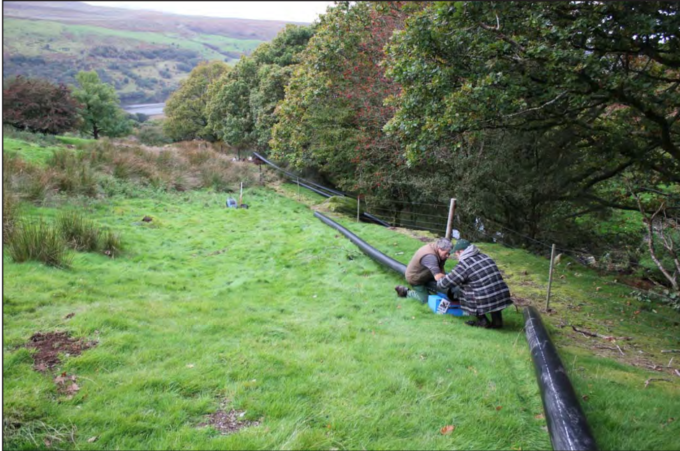
Plate 32: Laying out of pipe along route ahead of installation in the river gorge - no scale
