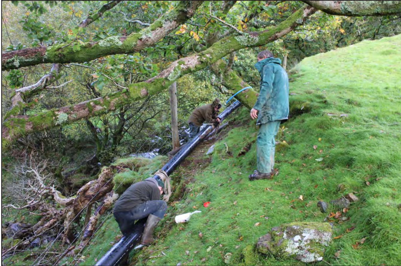
Plate 27: Working shot of assembly of the pipe around the SAM erosion scar - no scale
