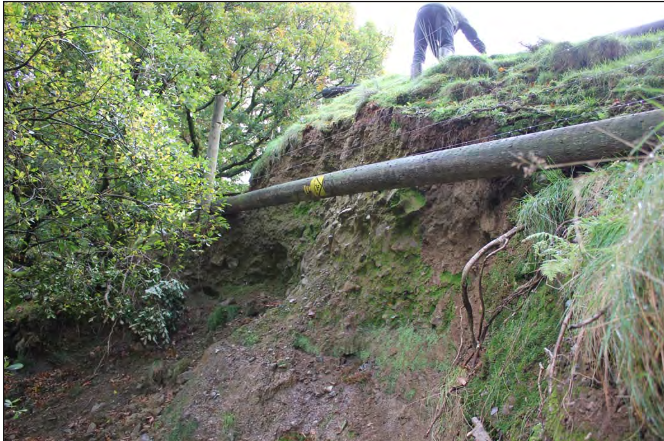
Plate 25: Mitigation response routing the pipe around the SAM erosion scar (Horizontal timber to support pipe) - no scale
