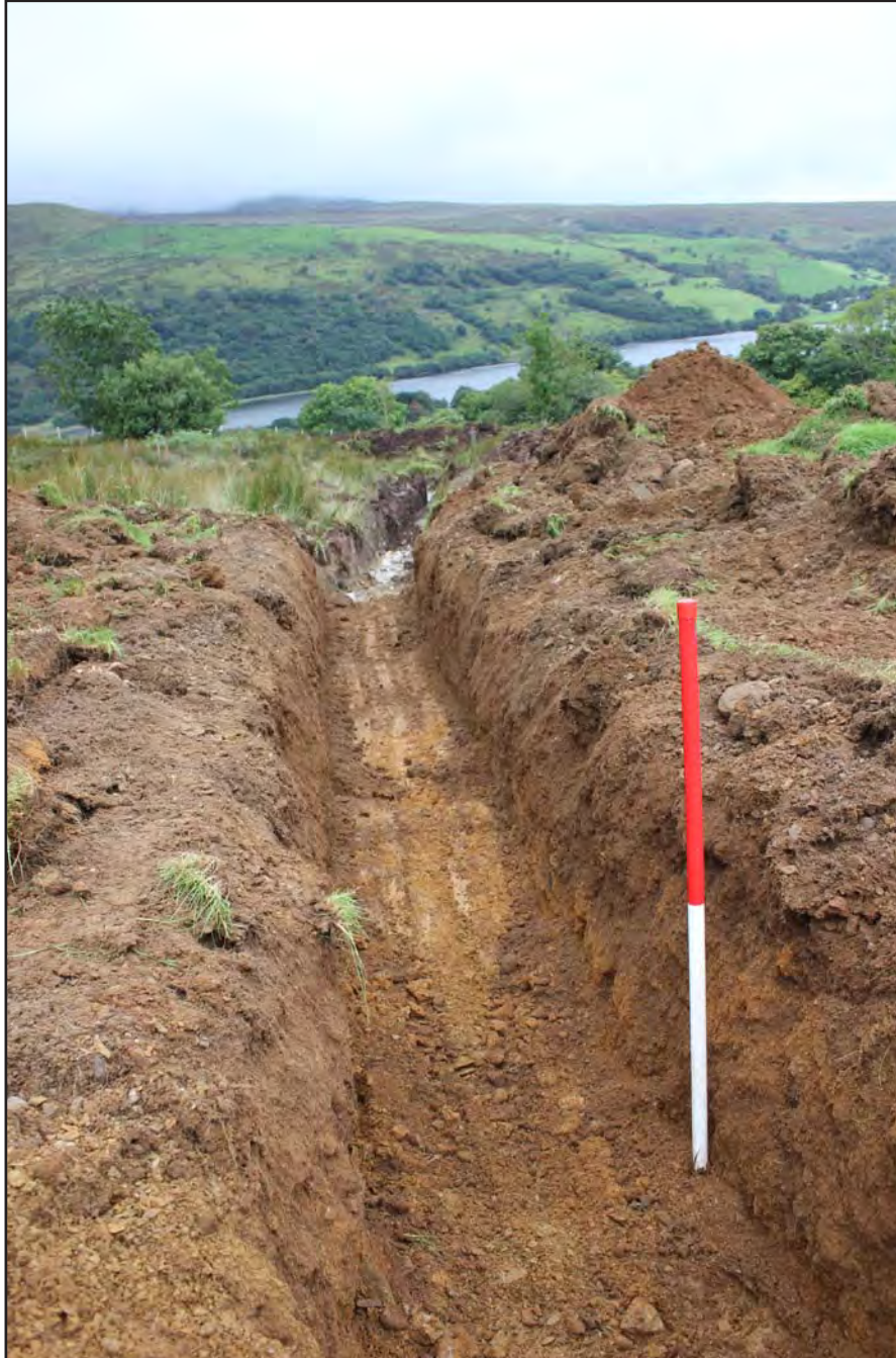
Plate 15: Penstock trench at CH450 looking South - 1m scale
