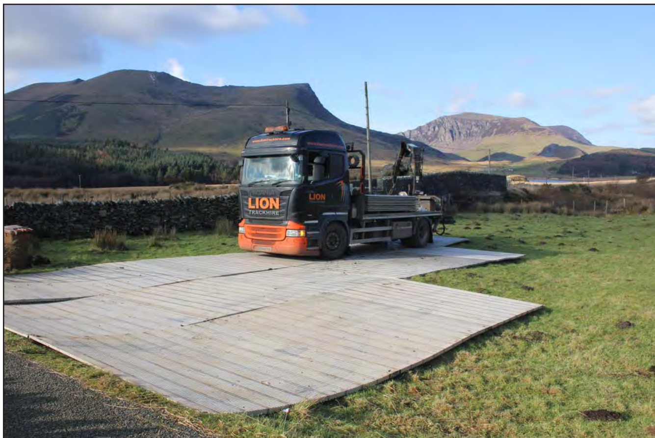
Plate 02: Laying down of temporary access track for launch pit, from the southeast.
