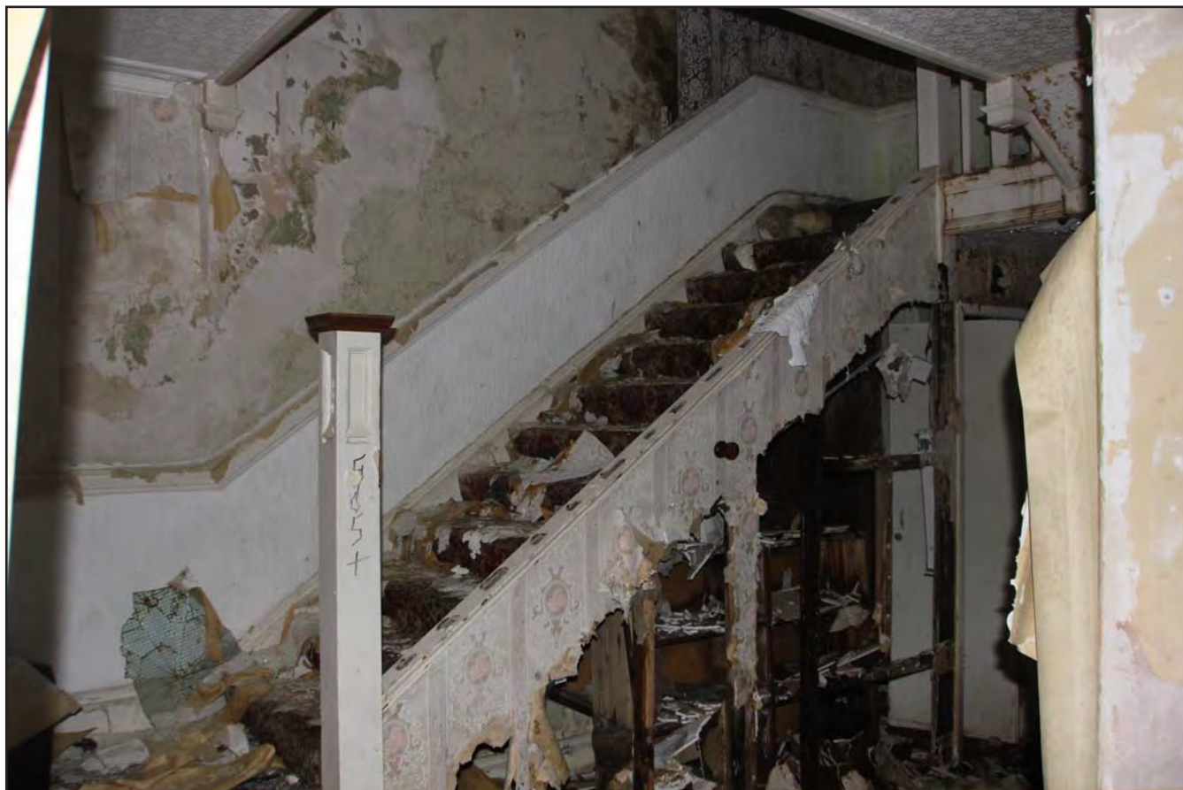
Plate 31: The Whitehouse Hotel ground floor Stairwell showing water damage, from the east.
