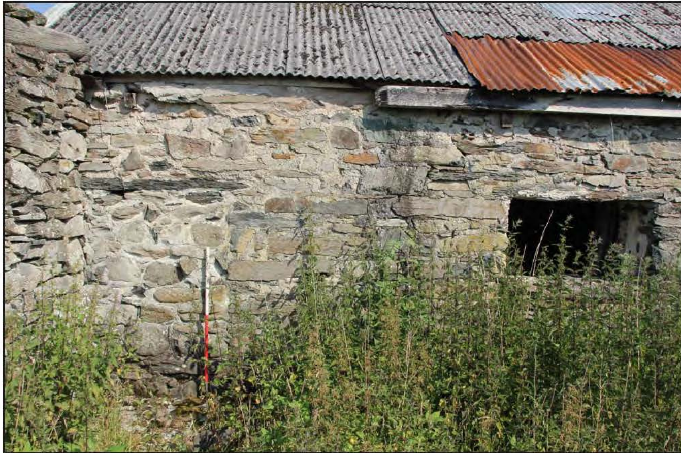
Plate 05: Southeast facing external elevation (southwest end) showing blocked doorway, from the southeast. Scale 1.0m.
