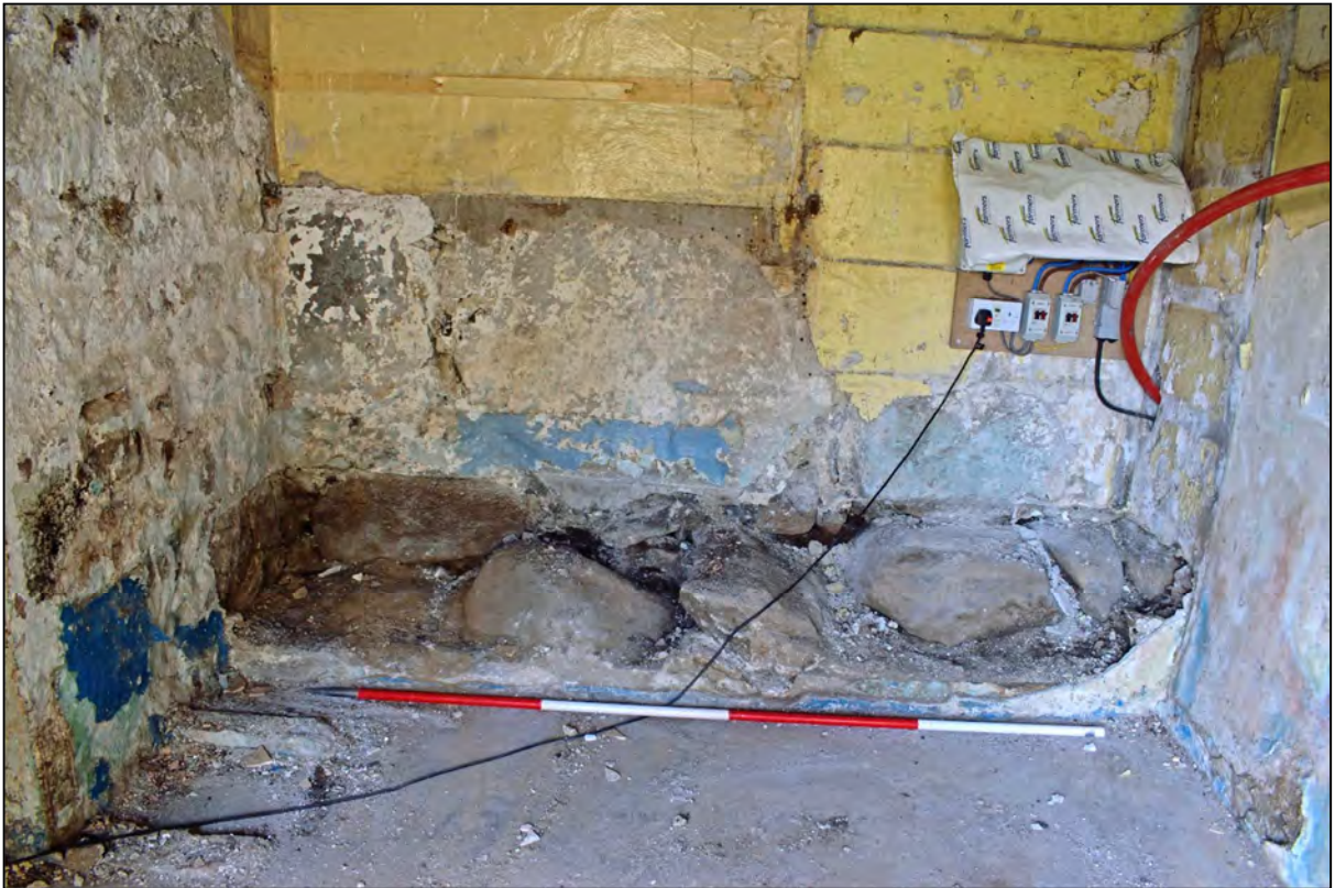
Plate 19: Foundation exposed in the Utility Room.
