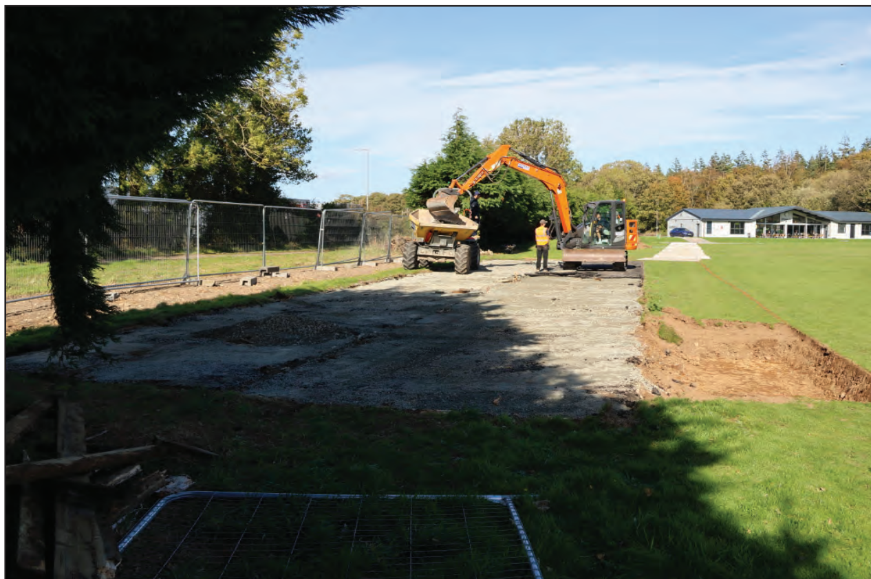
Plate 5: Removal of tarmac layer on existing practice area; scale not used; view from SSW (archive reference: E49366_016).
