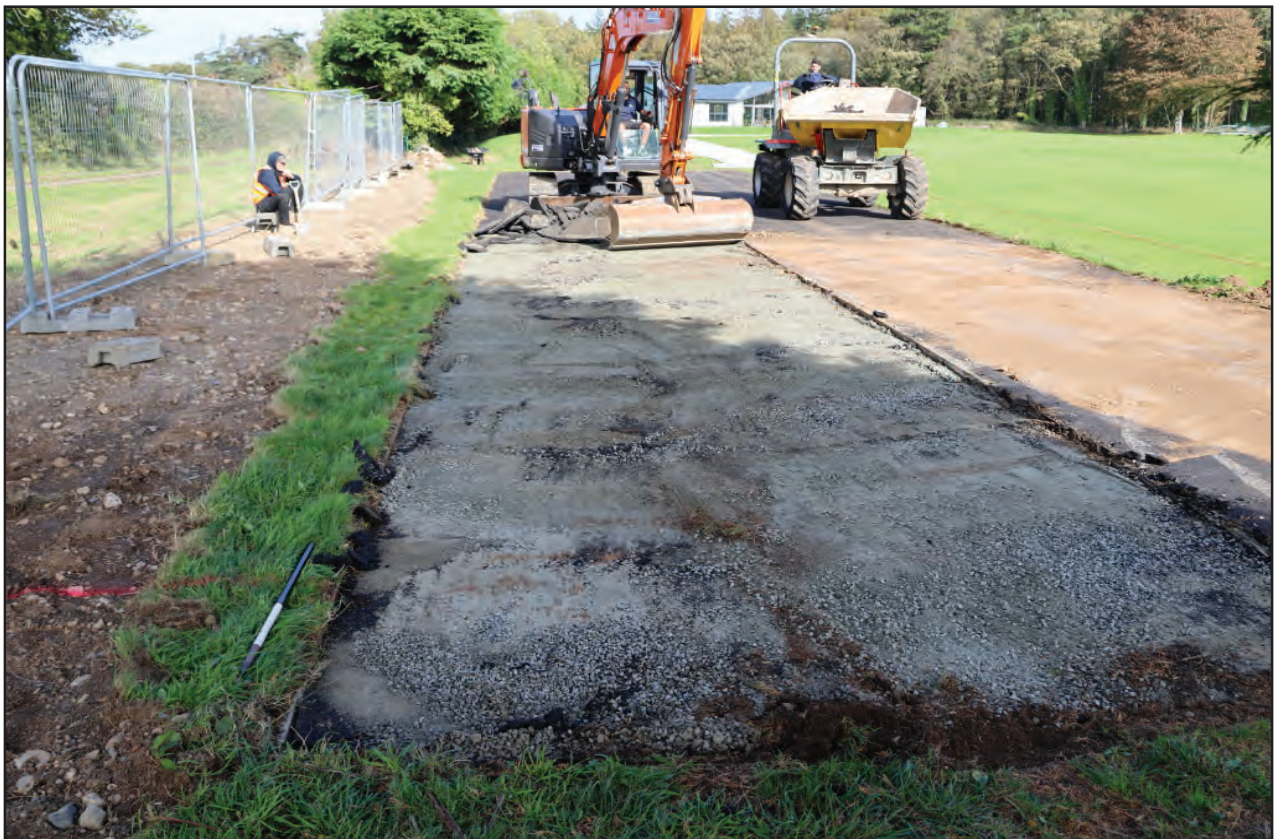
Plate 4: Removal of tarmac layer on existing practice area; scale 1x1m; view from WSW (archive reference: E49366_014).
