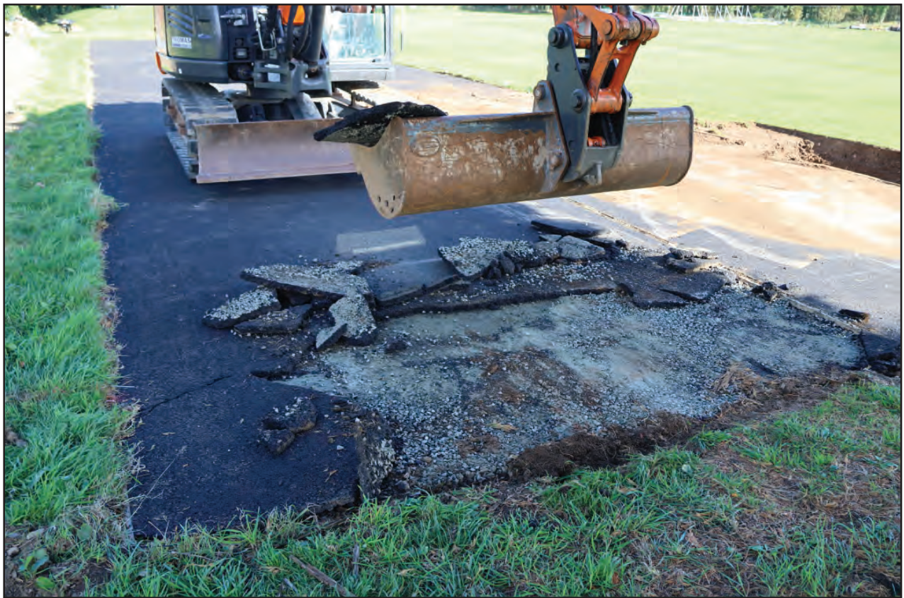
Plate 3: Removal of tarmac layer on existing practice area; scale not used; view from WSW (archive reference: E49366_012).
