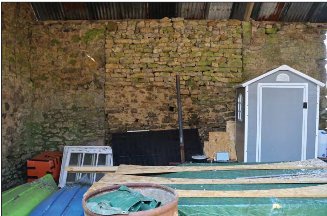
Plate 78: Interior - View showing blocked up opening in NW wall of OB8; scale not used; view from SE (archive reference: E49216_94).
