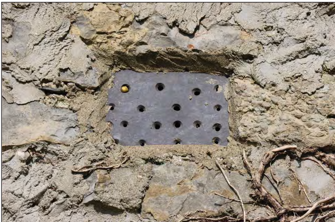
Plate 30: Exterior - Close-up shot of slate grate in E facing elevation of OB3; scale not used; view from E (archive reference: E49216_40).
