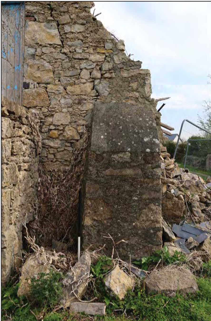
Plate 21: Exterior - View of modern buttress built to support SW gable end of R6 and R7; scale 1x1m; view from SW (archive reference: E49216_30).
