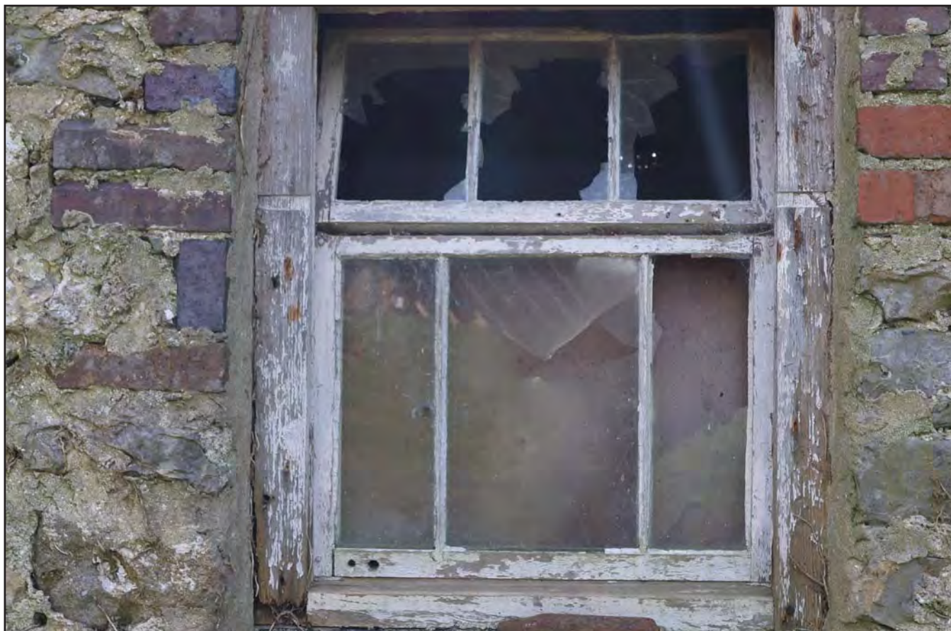
Plate 27: Exterior - Window in OB3 showing slate lintel and sill; scale not used; view from NW (archive reference: E49216_37).
