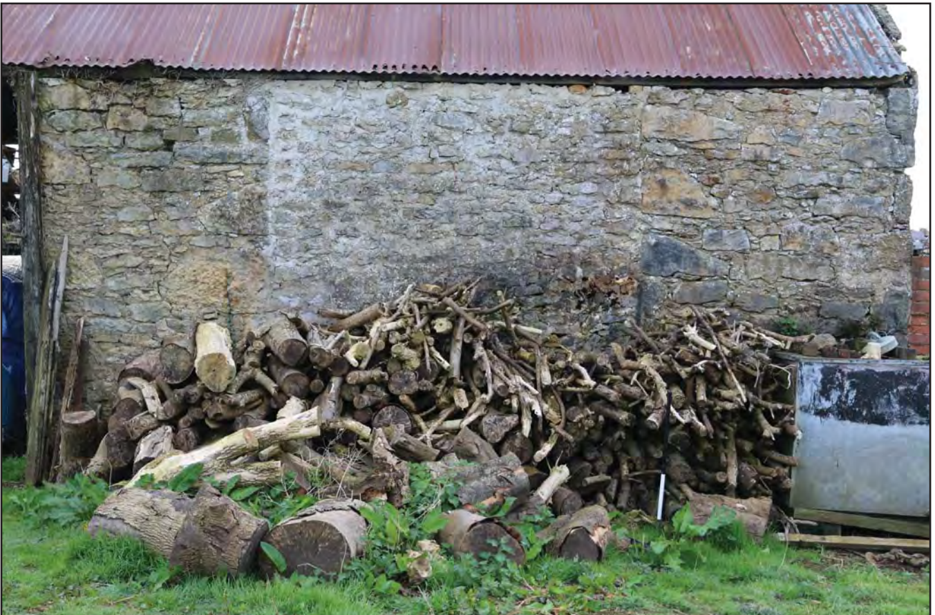
Plate 8: Exterior - NW elevation of the barn showing blocked up opening (OB8); scale 1x1m; view from NW (archive reference: E49216_09).
