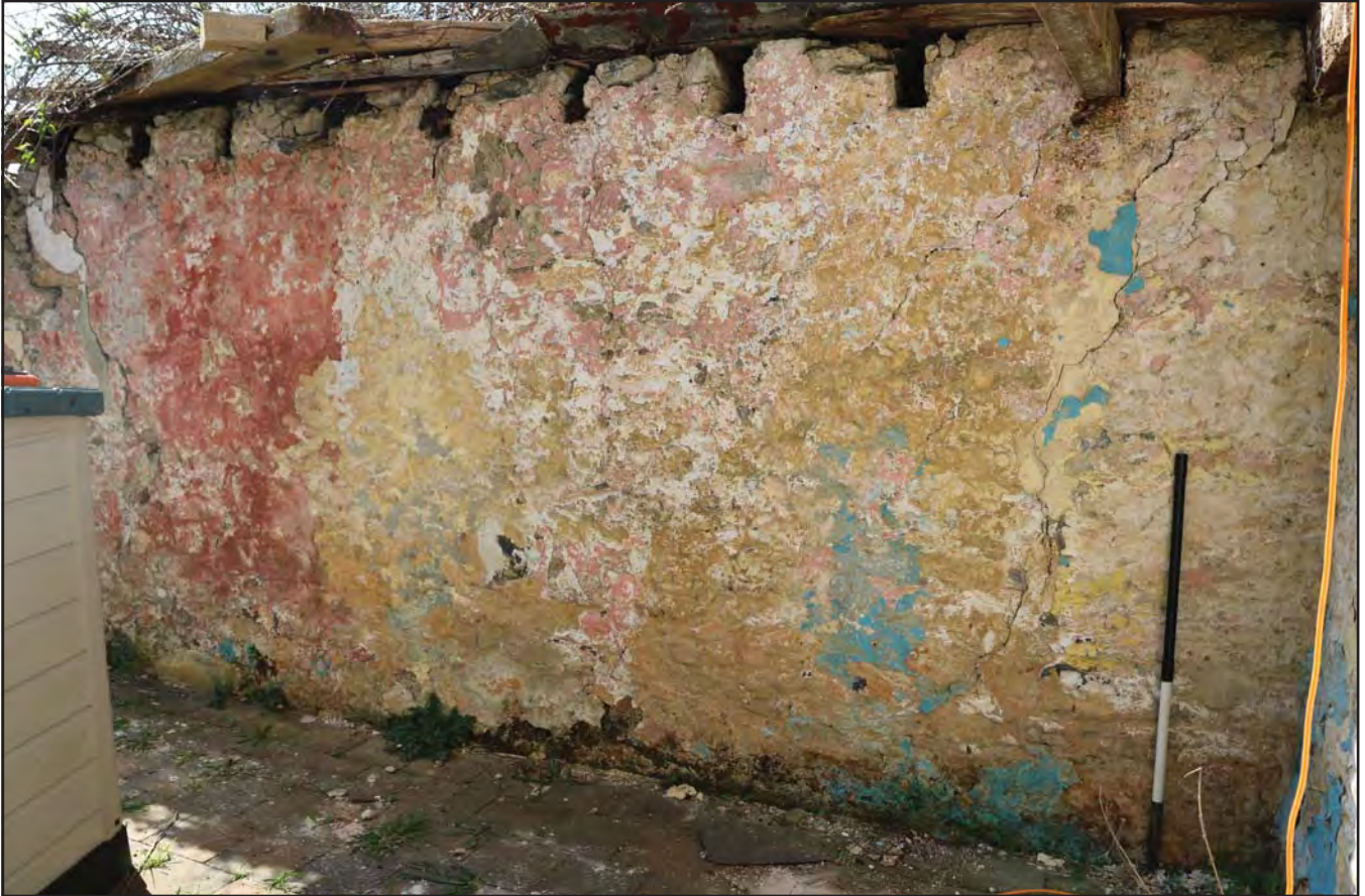
Plate 47: Interior - View of SW wall of R3 showing joist slots; scale 1x1m; view from N (archive reference: E49216_63).
