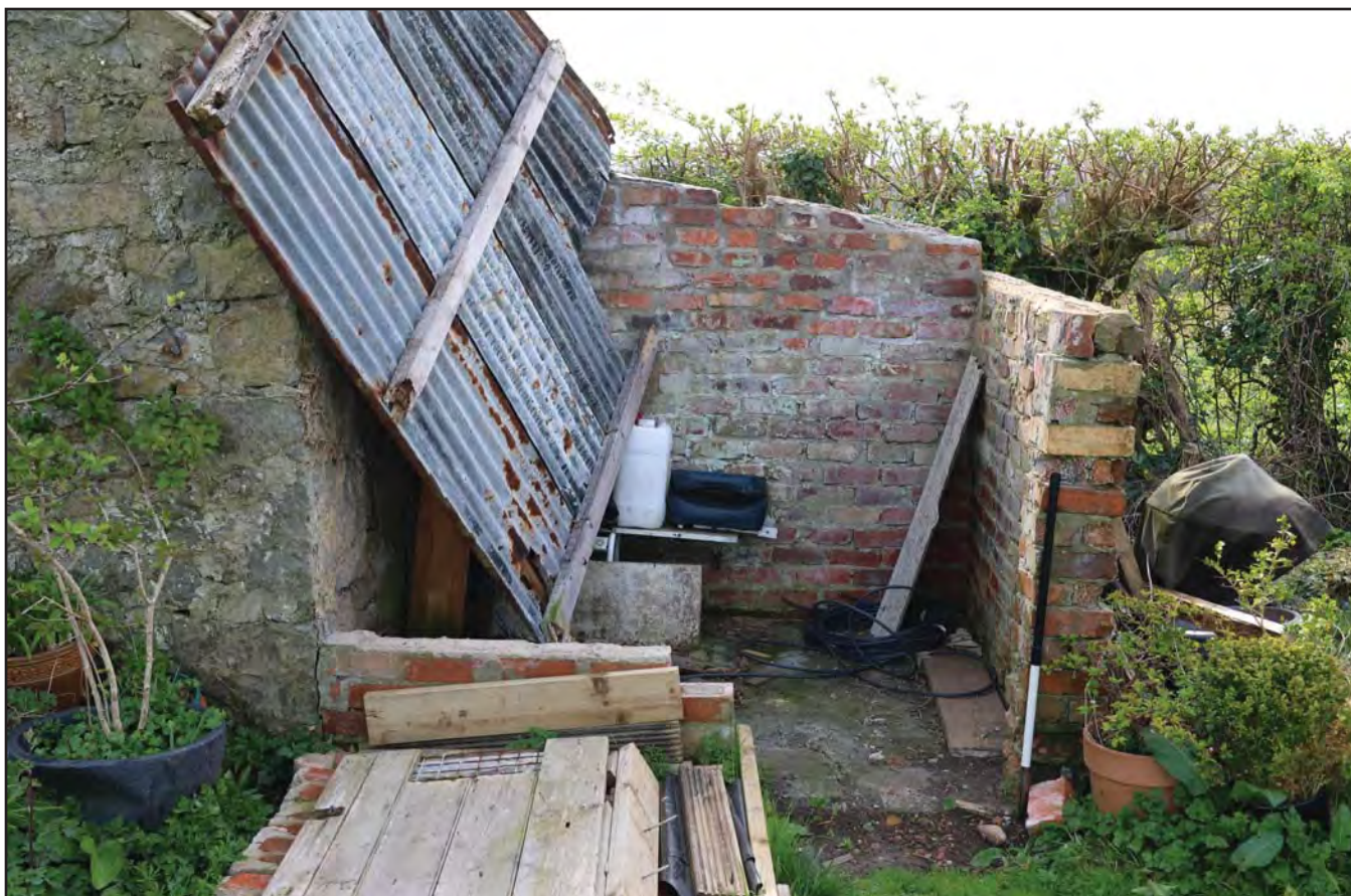
Plate 24: Exterior - View of NW elevation of OB 4 showing roof collapsed into R17; scale 1x1m; view from NW (archive reference: E49216_34).
