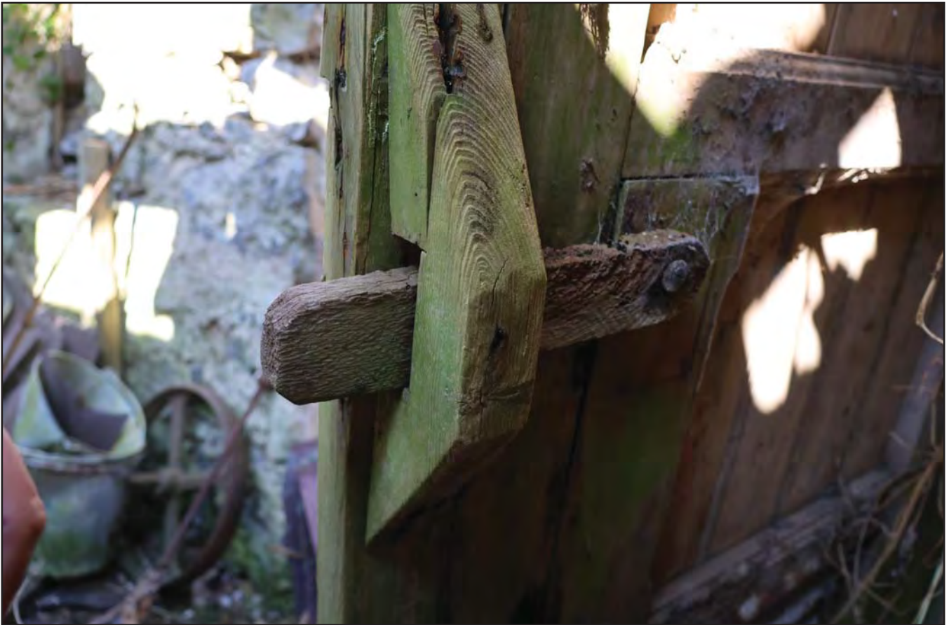
Plate 85: Interior - Wooden latch on back of door of OB6; scale not used; view from SW (archive reference: E49216_101).
