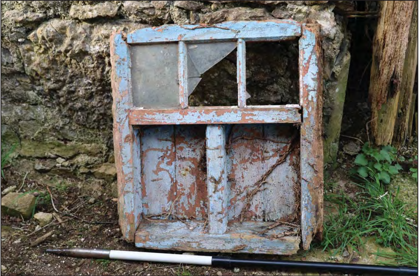
Plate 15: Exterior - View of an original window with wooden frame, 3 panes of glass above a shuttered bottom opening previously removed (front); scale 1x1m; view from NE (archive reference: E49216_22).
