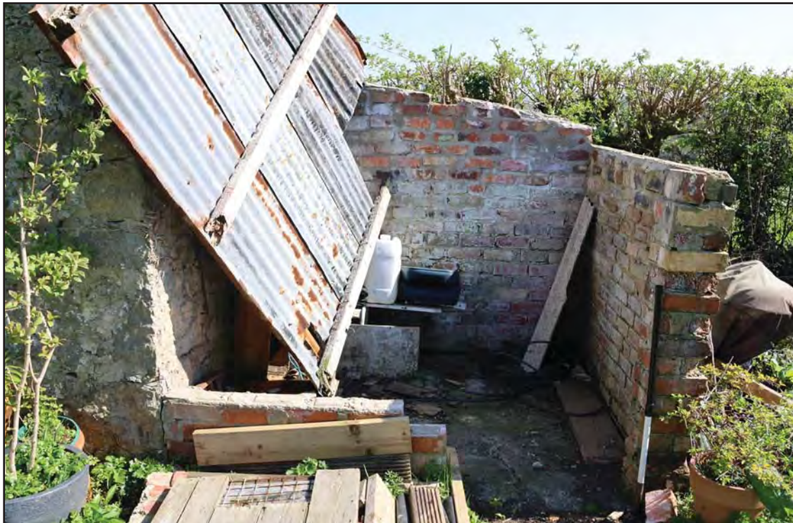
Plate 94: Interior - View of OB4, collapsed roof and wall; scale 1x1m; view from NW (archive reference: E49216_111).
