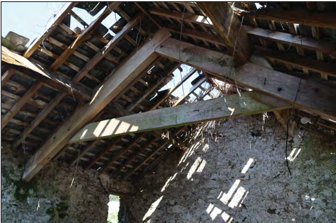
Plate 75: Interior - View of wooden A frame in roof of R5; scale not used; view from SW (archive reference: E49216_91).
