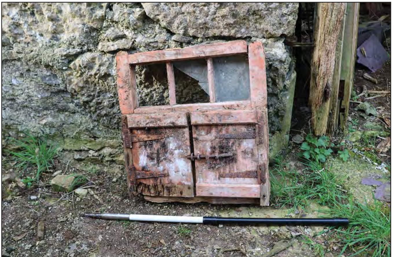
Plate 14: Exterior - View of an original window with wooden frame, 3 panes of glass above a shuttered bottom opening previously removed (rear); scale 1x1m; view from NE (archive reference: E49216_20).
