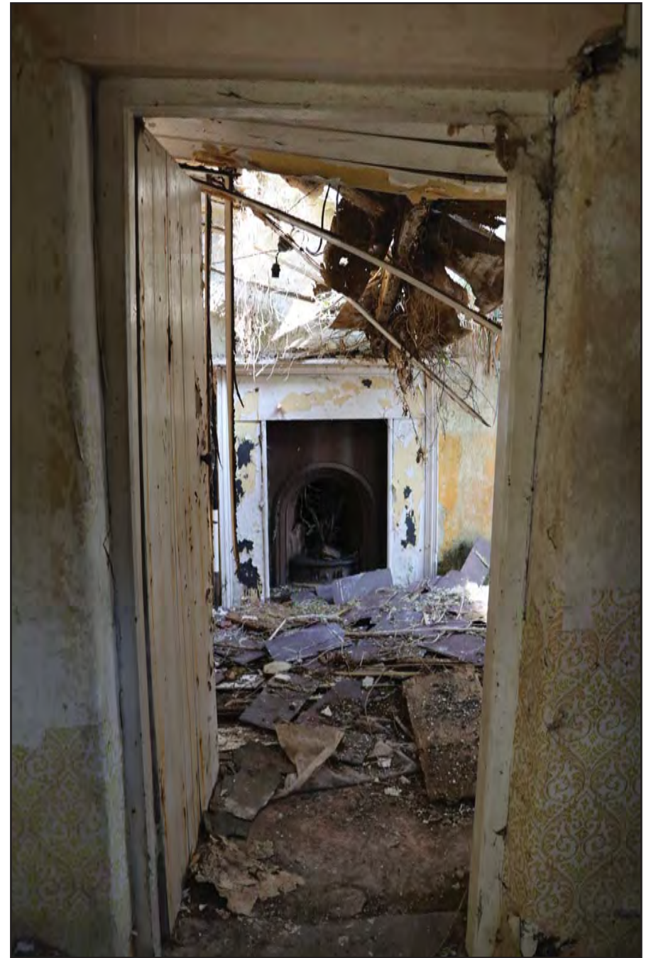
Plate 40: Interior - View showing collapsed ceiling in R2; scale not used; view from SW (archive reference: E49216_55).
