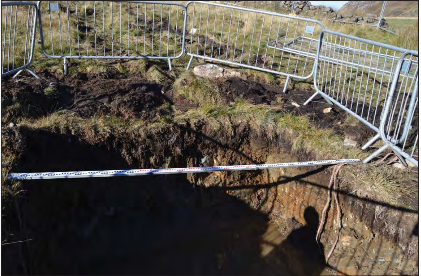
Plate 1: View of tower base pit showing topsoil and bedrock and length of pit; scale 1x3m; view from SE (archive reference: G2816_001).
