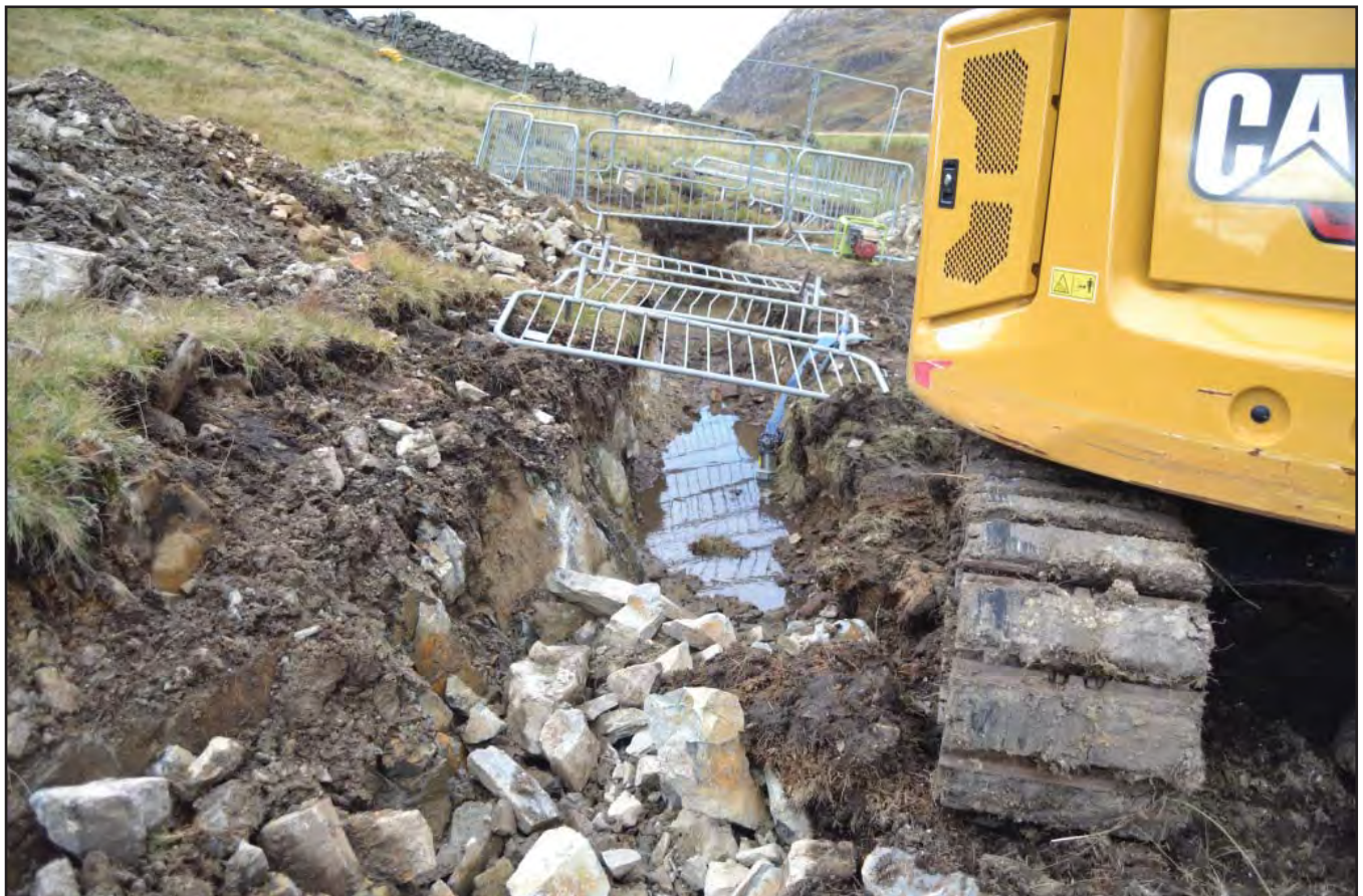
Plate 18: View along partially excavated cable duct trench; scale not used; view from ESE (archive reference: G2816_018).
