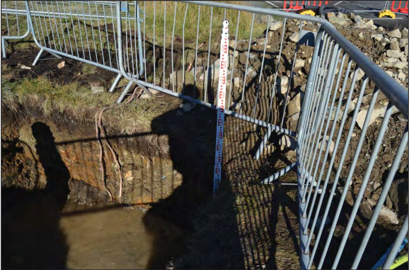
Plate 5: View of tower base pit showing topsoil and bedrock showing depth; scale 1x3m; view from SSE (archive reference: G2816_005).
