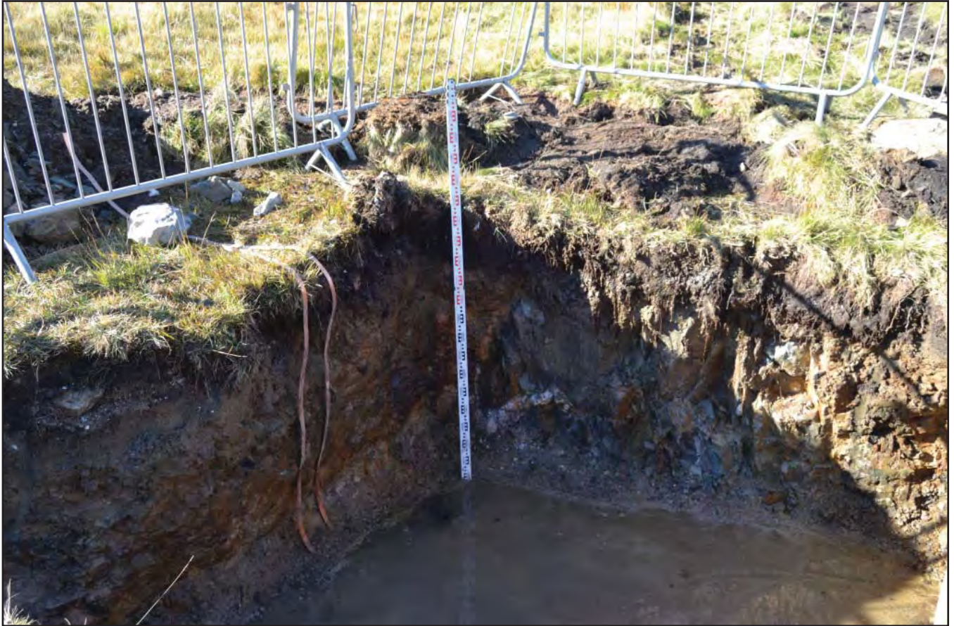
Plate 3: View of tower base pit showing topsoil and bedrock showing depth; scale 1x3m; view from E (archive reference: G2816_003).
