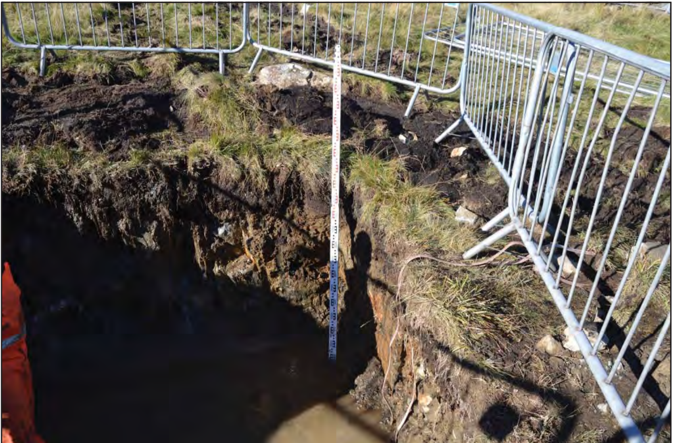
Plate 4: View of tower base pit showing topsoil and bedrock showing depth; scale 1x3m; view from SSE (archive reference: G2816_004).
