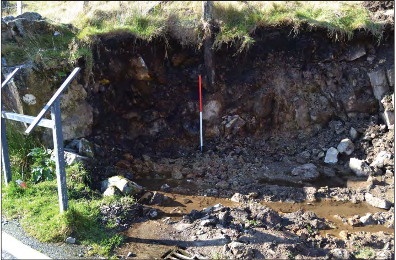
Plate 17: View of excavated area for cabinets showing depth of soil, fence post and bedrock in section; scale 1x1m; view from ESE (archive reference: G2816_017).
