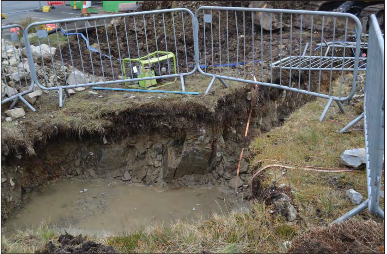
Plate 21: View of excavated pit for tower base and cable duct trench; scale not used; view from SW (archive reference: G2816_021).
