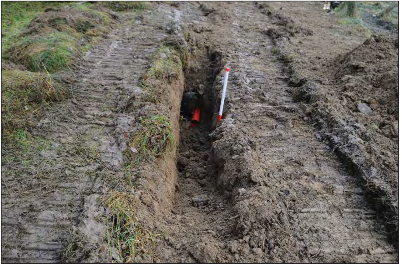
Plate 23: Mast/Shed Area - View showing part backfilled area in trench 2 with the cable duct in-situ; scale 1x1m; view from ENE (archive reference: HD24-054_023).
