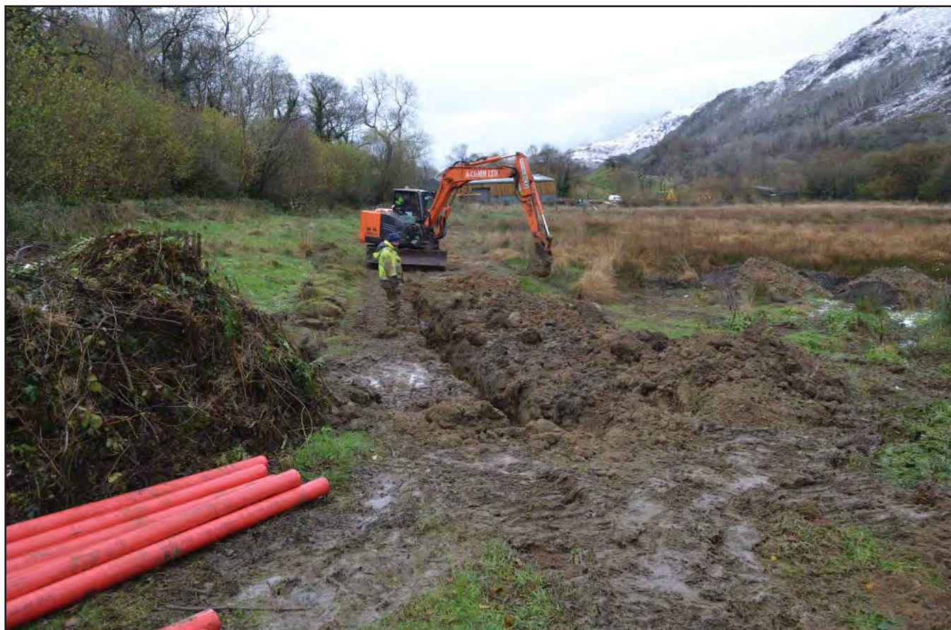
Plate 14: Field 1 - General working shot of cable duct trench excavation; scale not used; view from ENE (archive reference: HD24-054_014).
