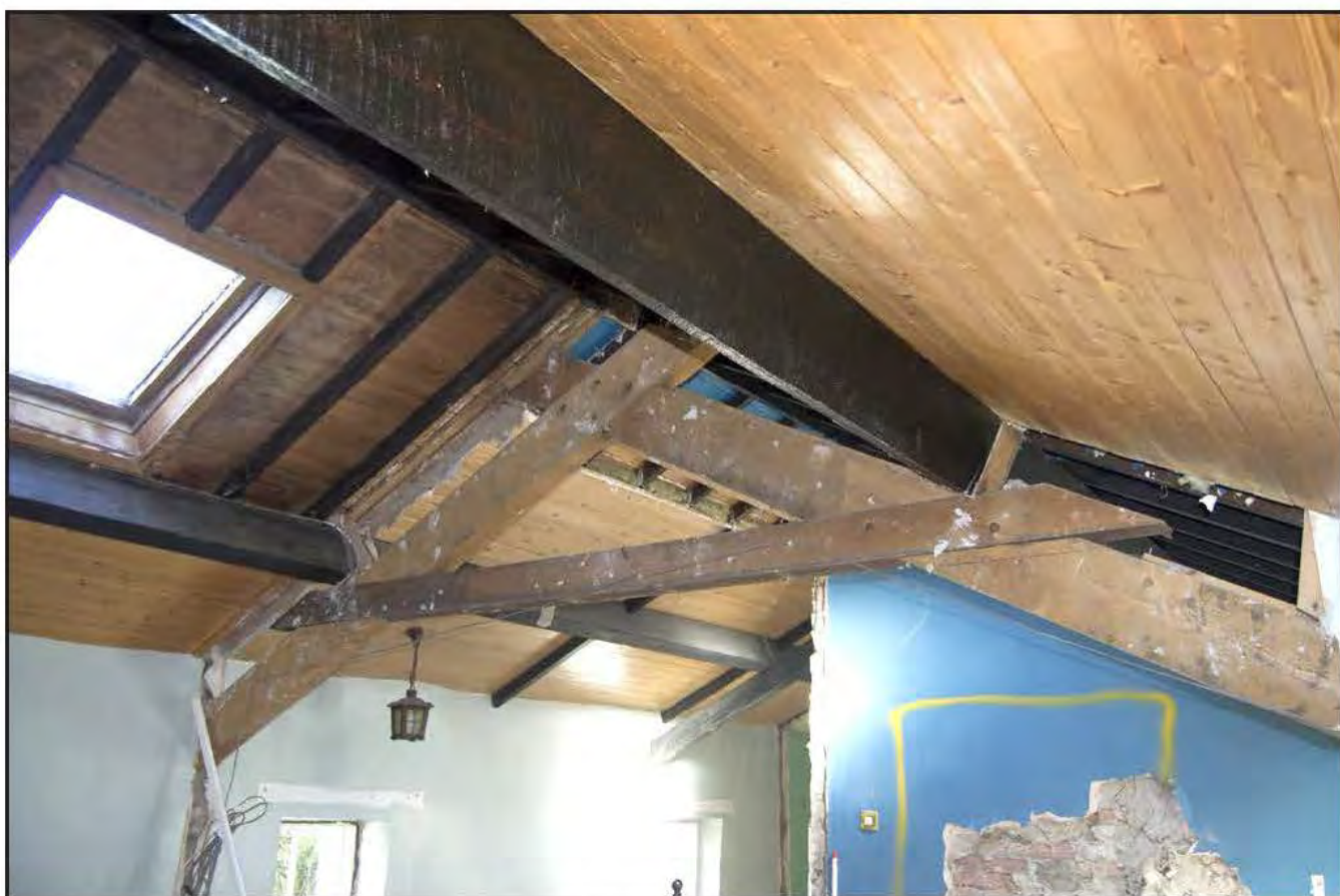
Plate 44: Room 06 - View of A-shaped truss, purlins and wooden roof beams; scale 1m; view from SW (archive reference: G2806_44).
