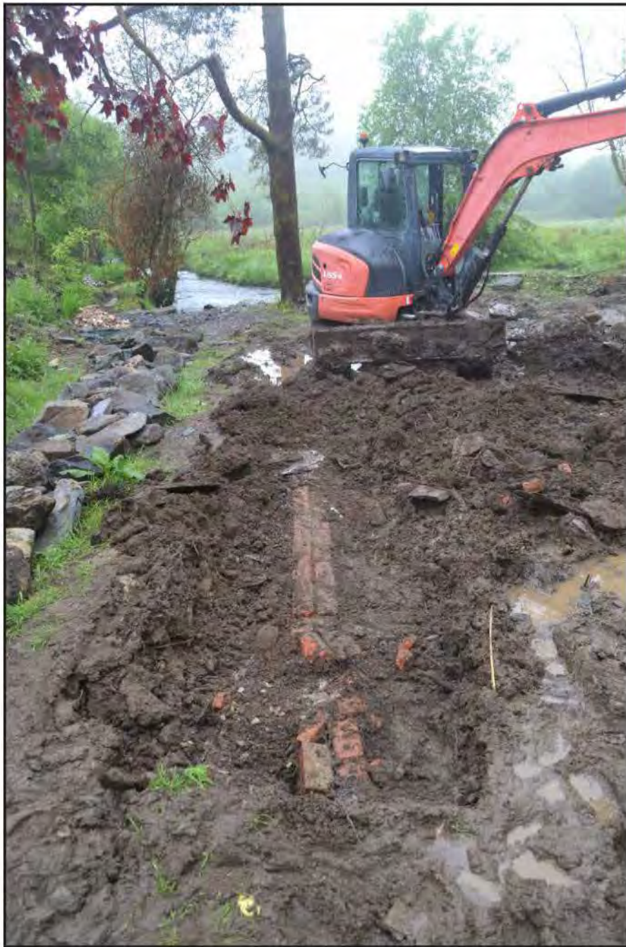
Plate 59: Excavated brick wall which was run off for the old septic tank, view from the north; scale: not used (archive reference: G2806_59).
