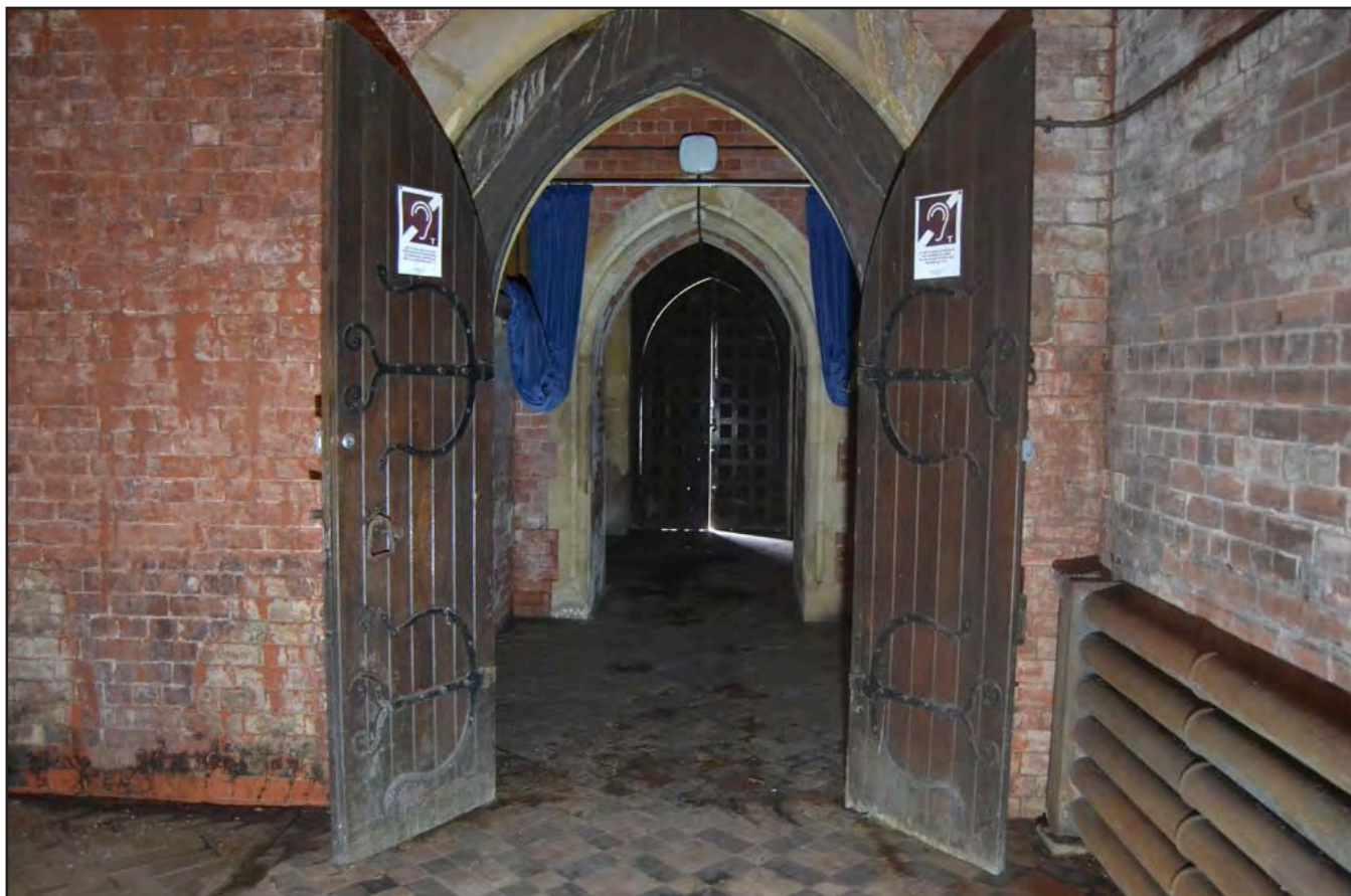
Plate 31: View of entrance door to nave showing heavy cast wooden door supported by blacksmith made elaborate and large scroll hinges, from the northwest - ; scale: not used (archive reference: G2824_53).
