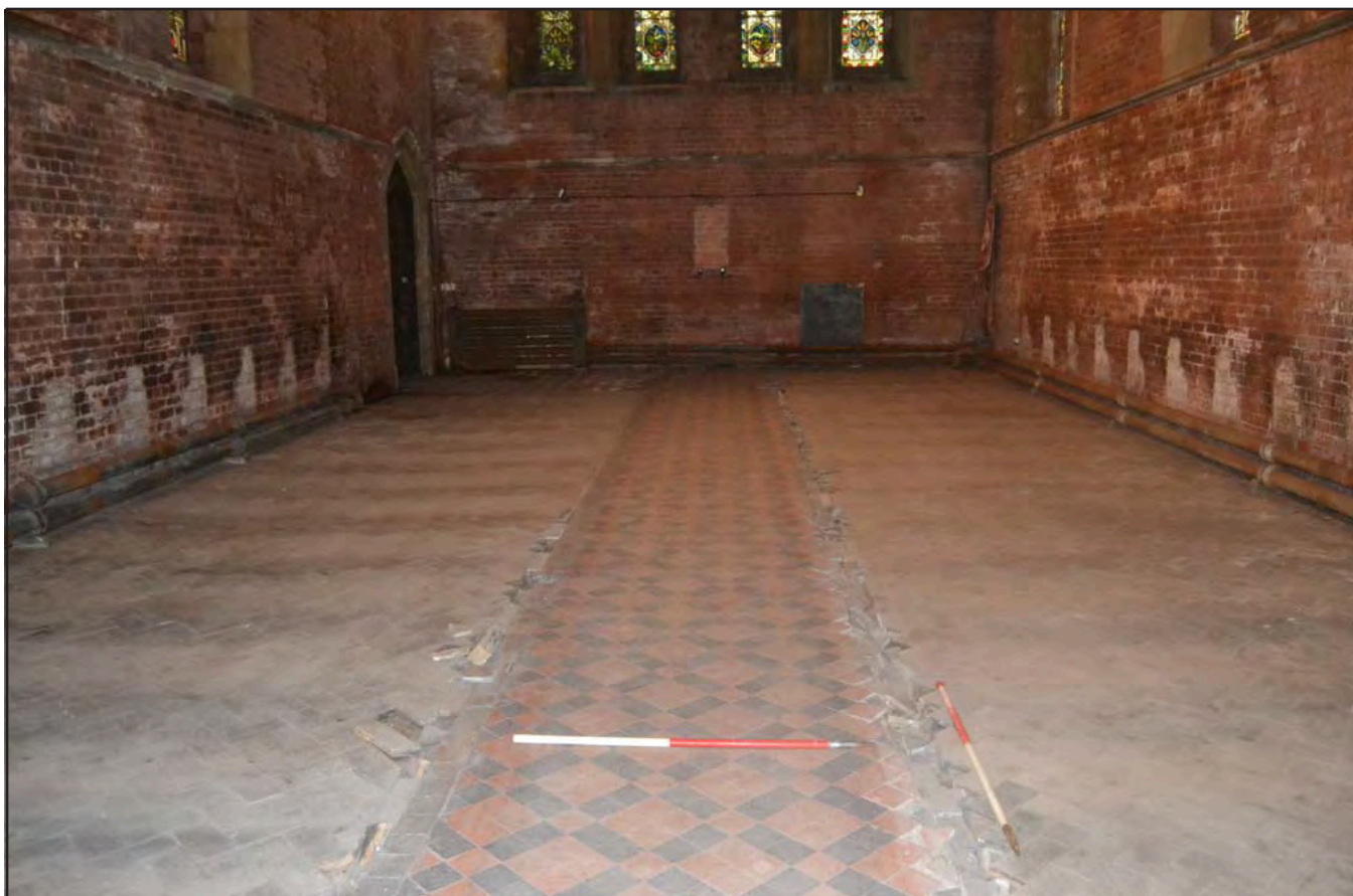
Plate 08: View of Parquet floor placed each side of nave and beneath the pews with a tiled centre (red carpet removed) leading up to the chancel, from northeast- ; scale: 2x1 m (archive reference: G2824_30).
