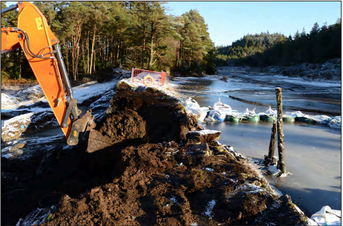
Plate 19: Excavation of spillway through embankment; Scale: Not used; view from SSW (archive reference: G2826_020).
