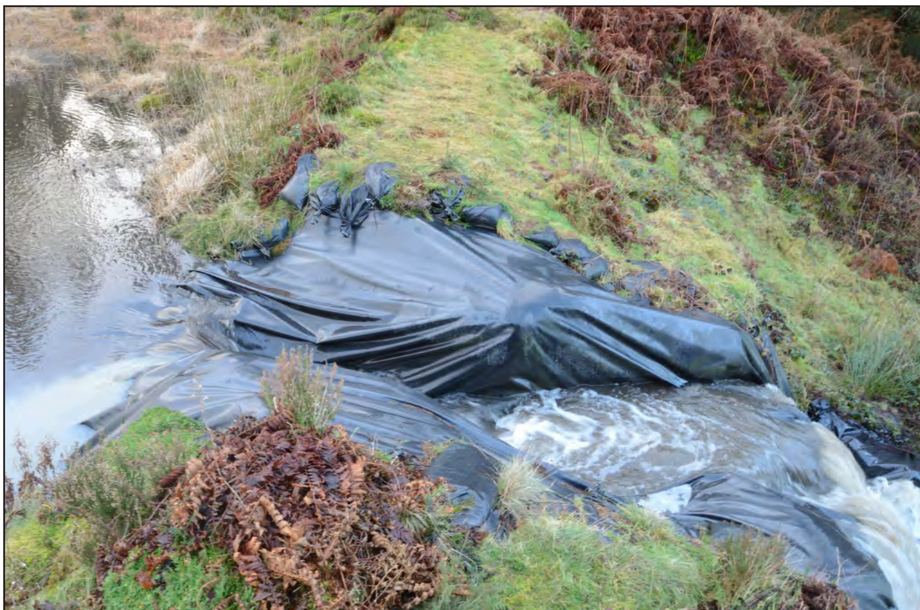
Plate 8: Tarpaulin covered breach through lower embankment; Scale: Not used; view from NNE (archive reference: G2826_058).
