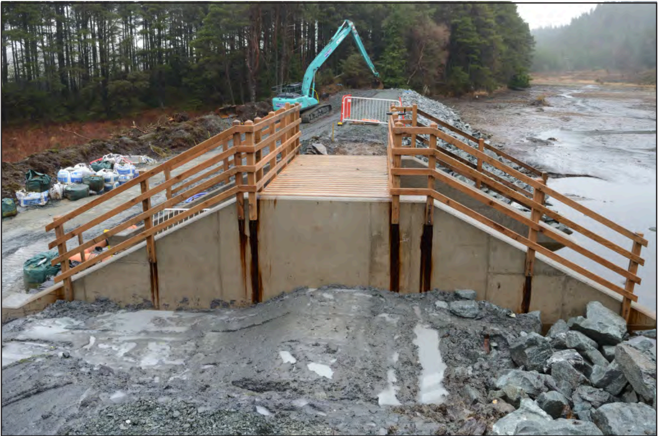
Plate 29: Completed spillway and bridge inserted within upper embankment; Scale: Not used; view from SW (archive reference: G2826_071).
