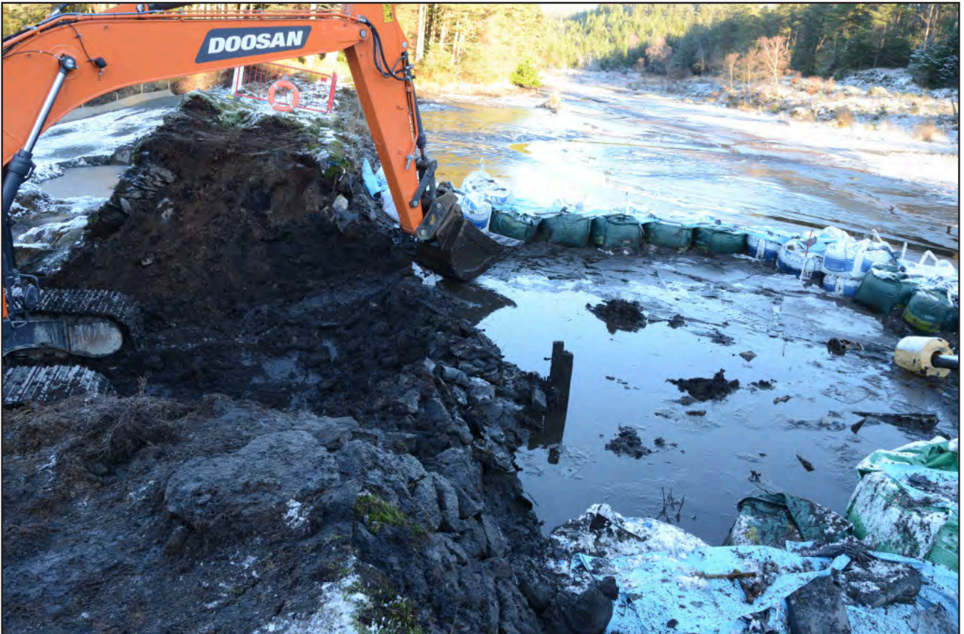
Plate 21: Excavation area of spillway within embankment and collar dam; Scale: Not used; view from SW (archive reference: G2826_041).
