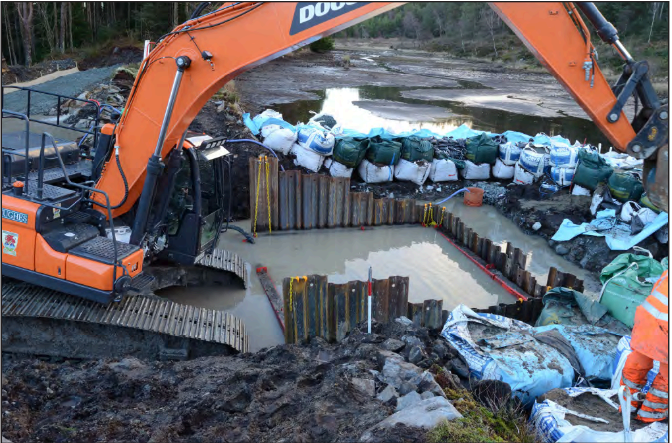
Plate 23: Steel coffer dam in place within spillway dig; Scale: Not used; view from SW (archive reference: G2826_044).
