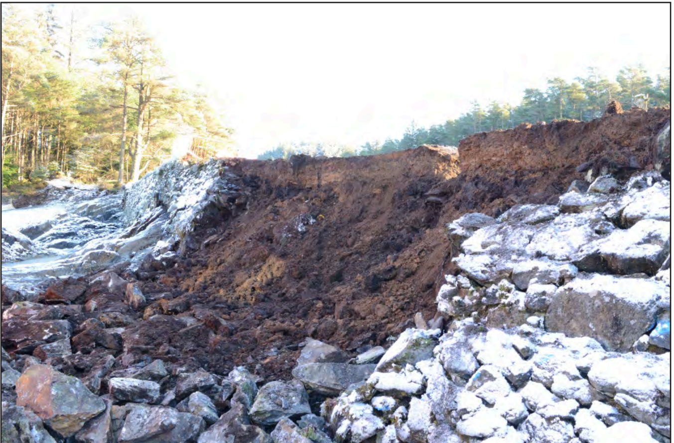
Plate 18: View of earth core of embankment exposed; Scale: Not used; view from SSW (archive reference: G2826_018).
