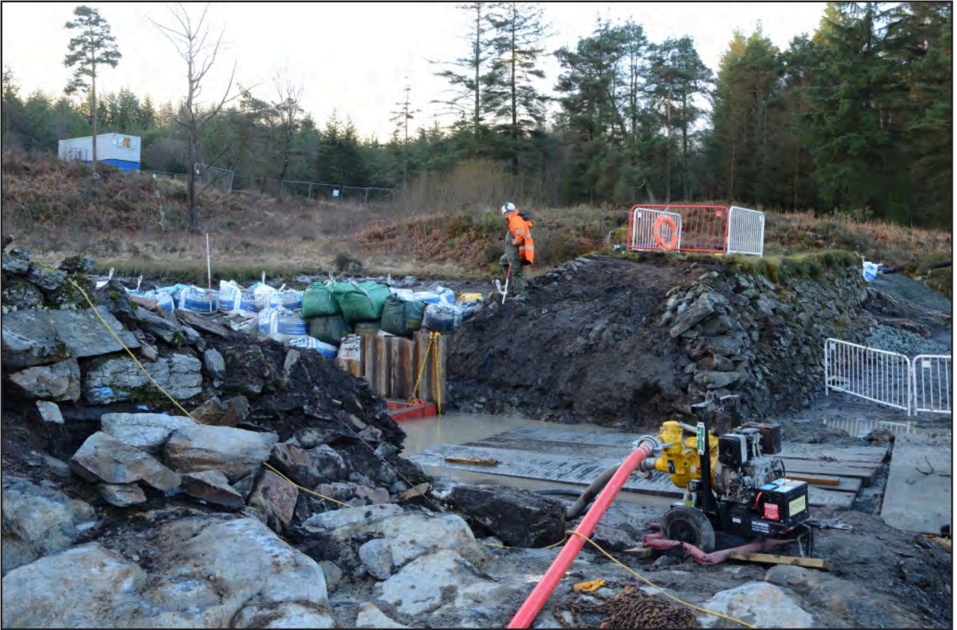
Plate 24: View of excavation for new spillway through embankment; Scale: Not used; view from N (archive reference: G2826_045).
