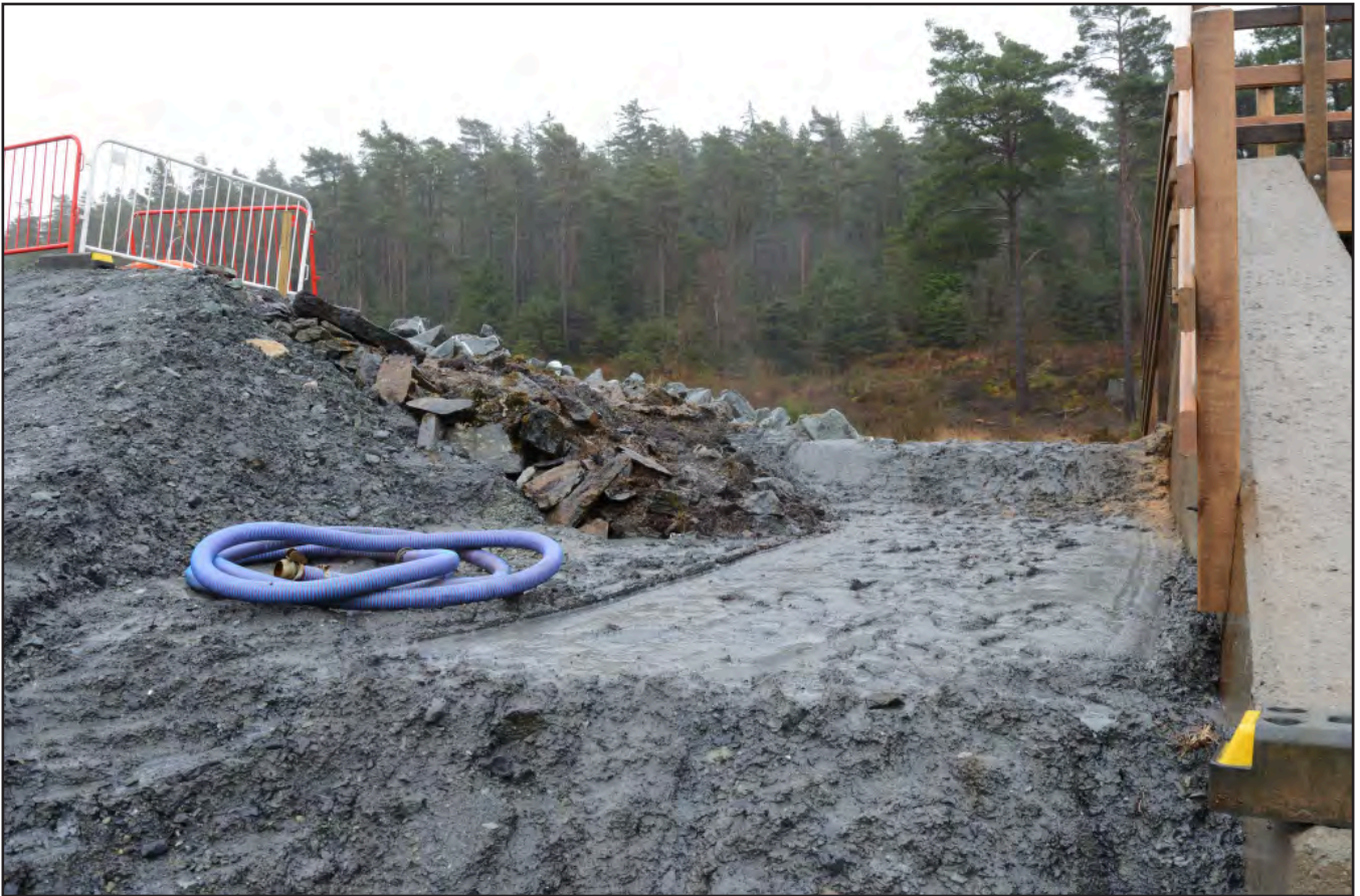
Plate 31: Imported clay over original embankment and next to spillway; Scale: Not used; view from W (archive reference: G2826_073).
