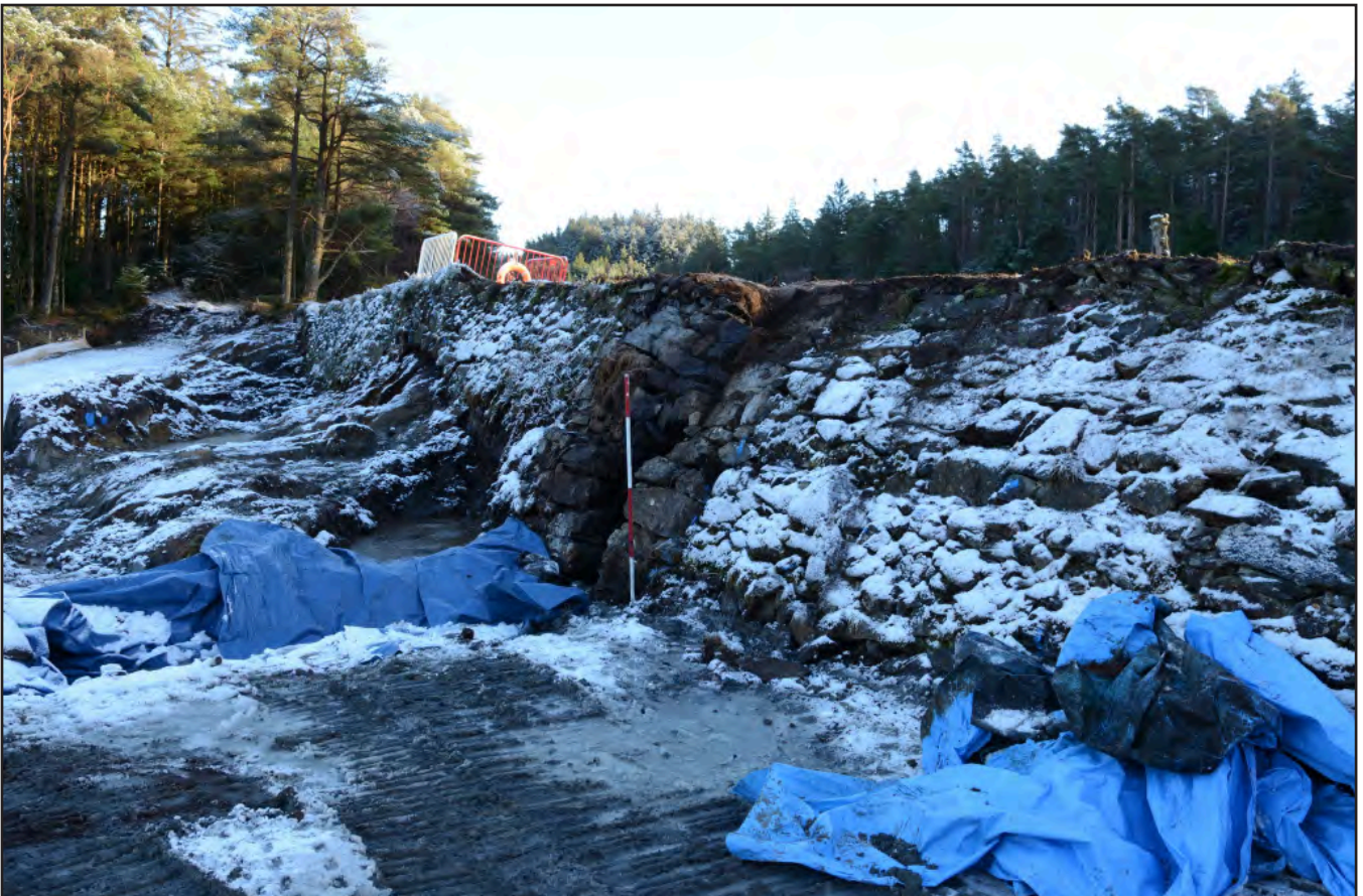
Plate 16: Location of breach and sluice opening in embankment; Scale: 1x2m; view from SW (archive reference: G2826_005).
