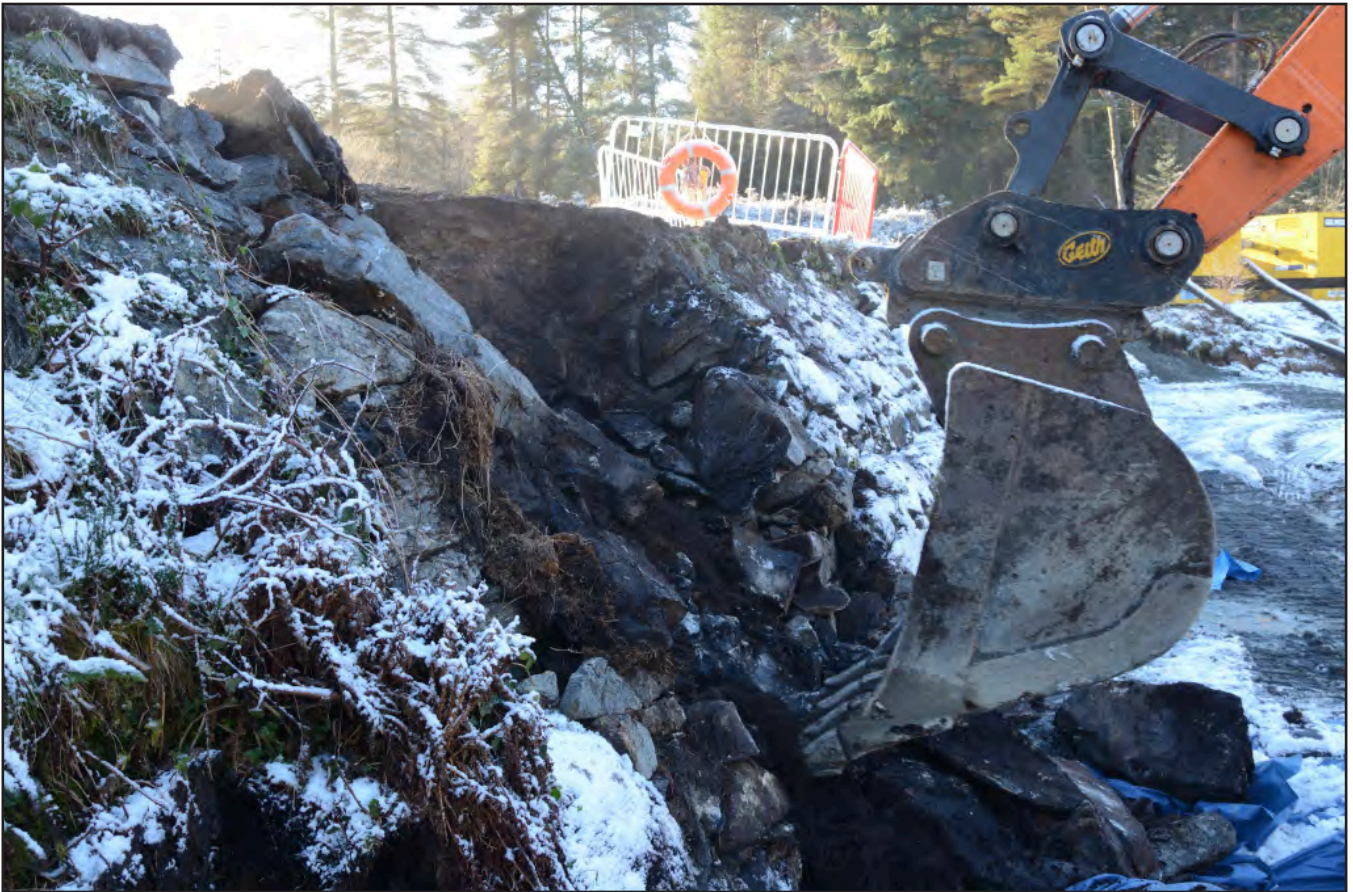
Plate 17: Excavation of spillway break of embankment wall; Scale: Not used; view from NNE (archive reference: G2826_011).
