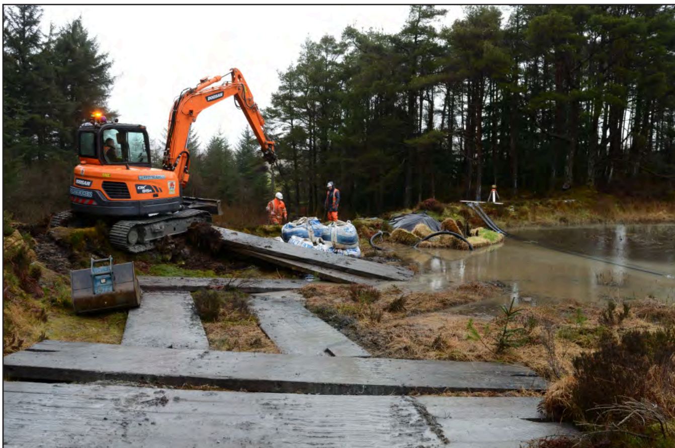
Plate 36: Bog mats and preparation for excavation; Scale: Not used; view from S (archive reference: G2826_067).
