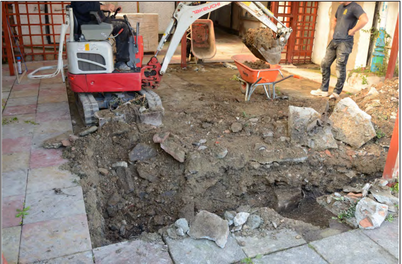
Plate 01: Excavation of foundation trench and removal of spoil with wheelbarrows; scale: not used (archive reference: ERN46808_013).
