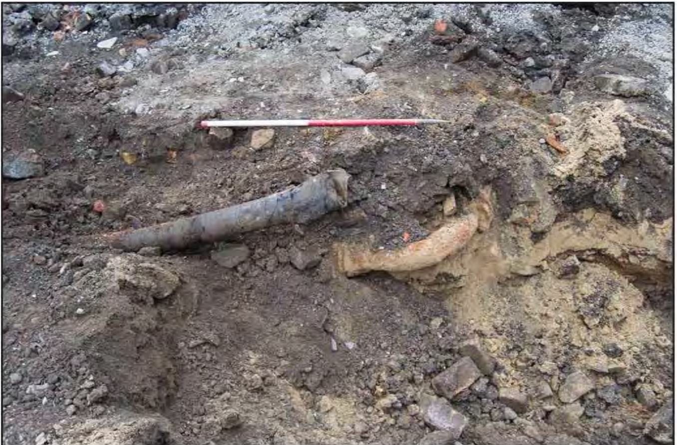
Plate 18: Additional two pipes discovered within pipe trench, one cast 90° bend and one mild steel wrapped in felt-; scale: 1x1m. View from: NE (archive reference: G26809_103).
