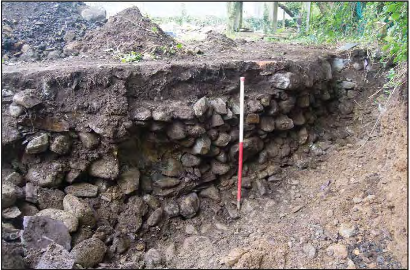
Plate 07: View of rubble stone exterior wall of circular gas work building-; scale: 1x1m. View from: W (archive reference: G26809_041).
