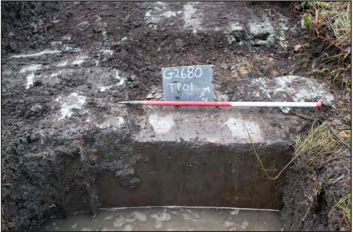
Plate 01: View of concrete foundation block of historic gas tank from the southeast-; scale: 1x1m. View from: SE (archive reference: G26809_008).
