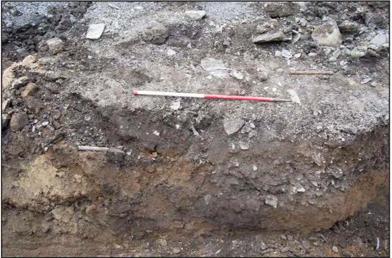
Plate 15: Representative section showing made ground and sand to the left from uncovered cast iron pipe-; scale: 1x1m. View from: NE (archive reference: G26809_102).
