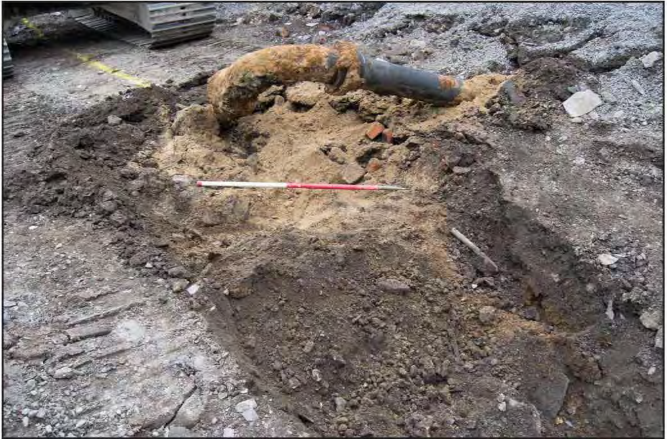
Plate 17: 250mm dia cast iron pipe with 90° bend exposed within pipe trench-; scale: 1x1m. View from: NNW (archive reference: G26809_100).
