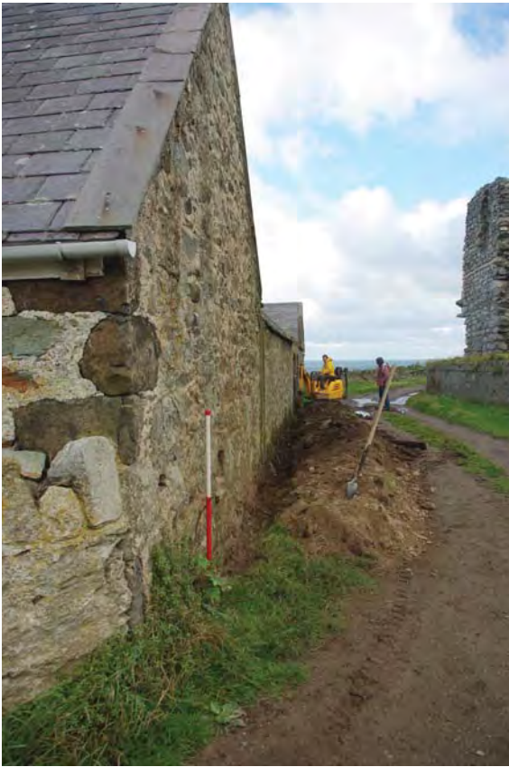
Plate 1. Cable trench being dug along-side Tŷ Nesaf/Tŷ Bach Barn
