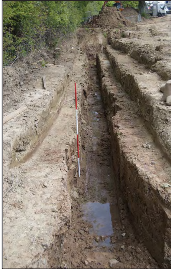
Plate 11: Gas mains pipe trench excavated. View from the west. 2 x 2m scale.
