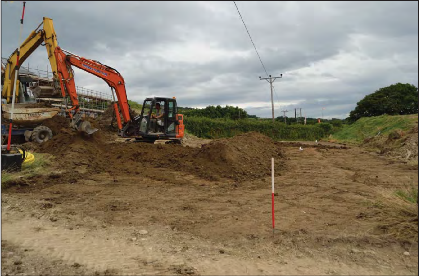
Plate 04: View of topsoil strip of Plots 49-52 with soil stored along outer perimeter. View from the south west. 1 x 1m scale.
