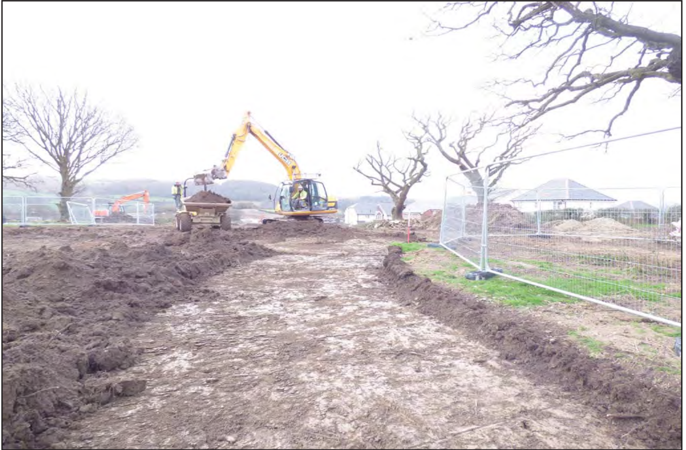
Plate 03: Topsoil strip of Build Phase B with 360° excavator and dumper. View from the north. 1 x 1m scale.
