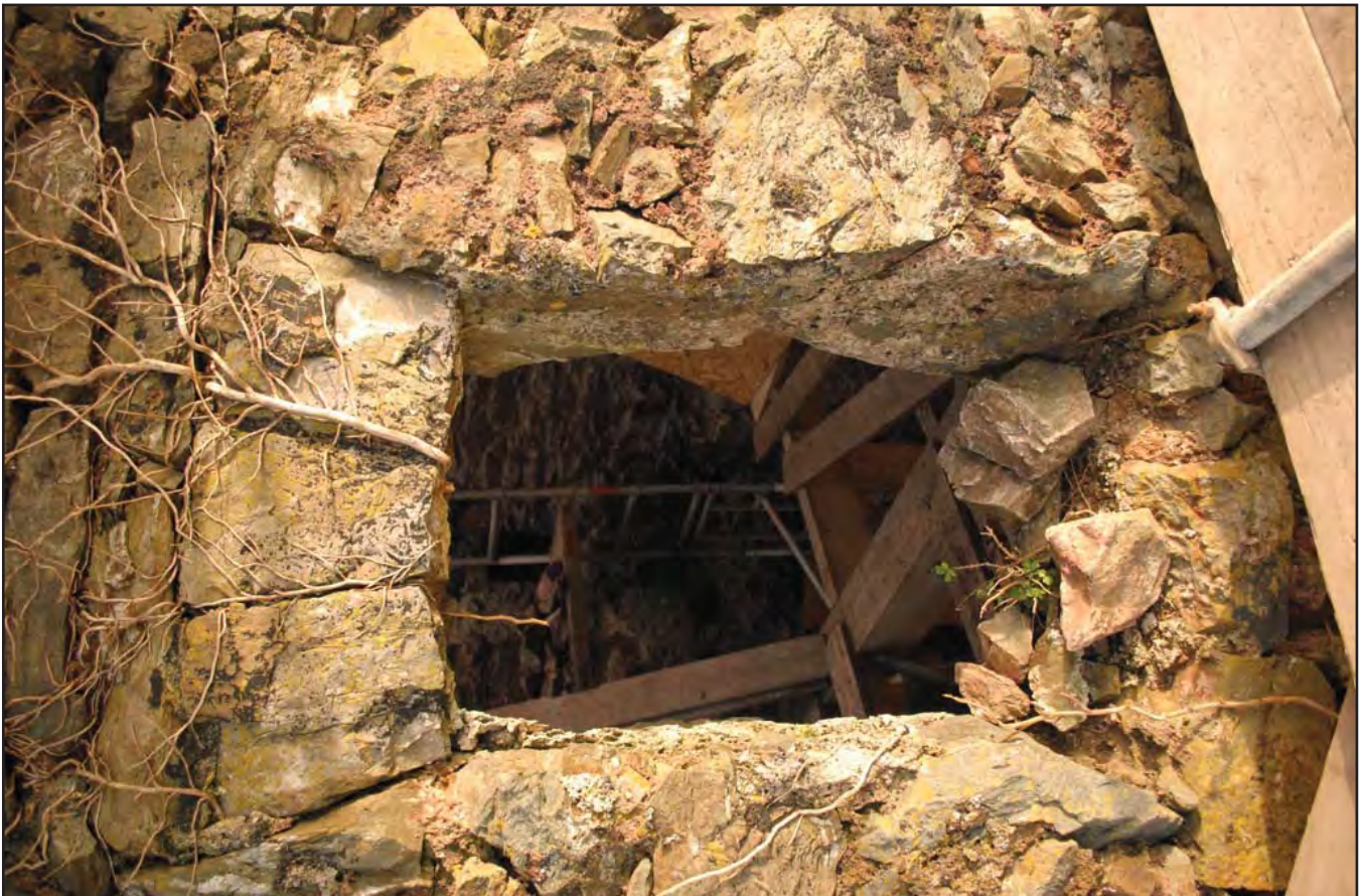
Plate 22: 2nd storey window detailing stone voussoirs. Photograph taken from the south east
