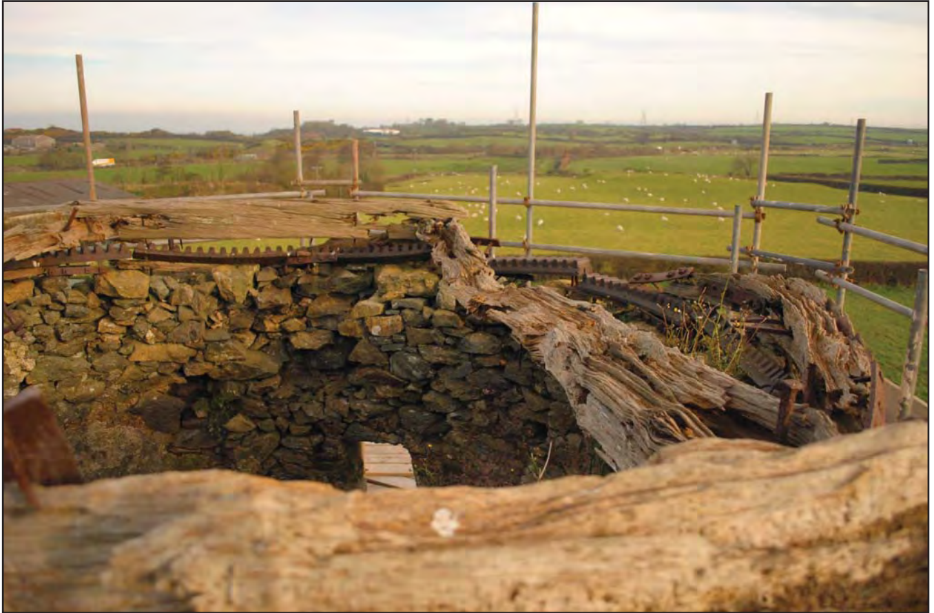
Plate 27: General view of turning cap detailing unstable upper wall & also revealing displaced cog wheel in segments. Photograph taken from the south
