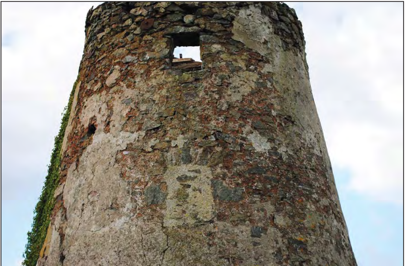
Plate 08: Shot looking upwards showing one blocked window on the 2nd floor & open window on the 3rd floor & significant surviving original lime render. Photograph taken from the north east
