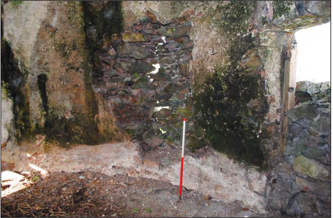
Plate 18: Shot detailing evidence of wall damage & wall render on undamaged surface. Photograph taken from the east
