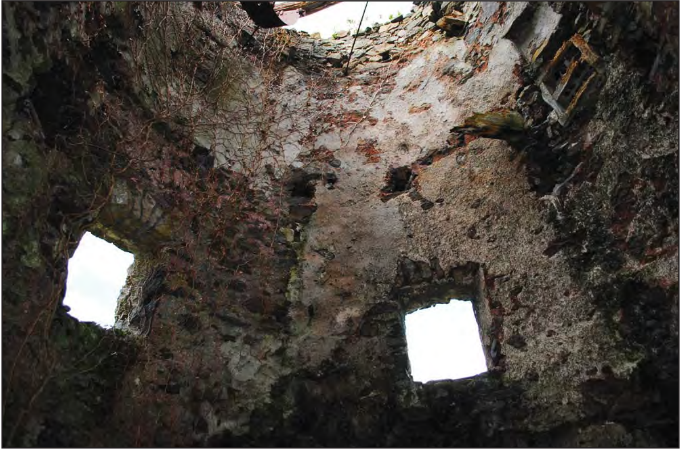
Plate 13: Shot looking upwards showing 2 open windows on the 2nd floor, blocked window on 3rd floor & remnants of roof joists and roof joist holes. Photograph taken from the east
