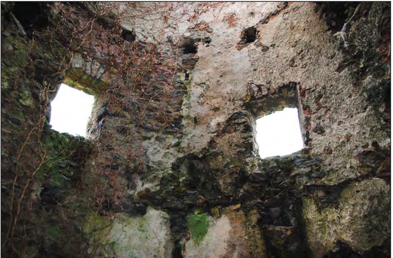
Plate 14: Shot looking upwards showing 2 open windows on the 2nd floor & roof joist holes. Photograph taken from the east
