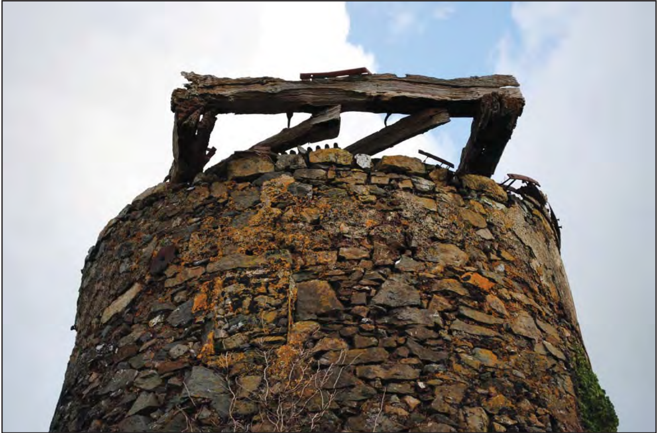
Plate 09: Shot of blocked window on 3rd floor & remnants of turning cap above. Photograph taken from the south
