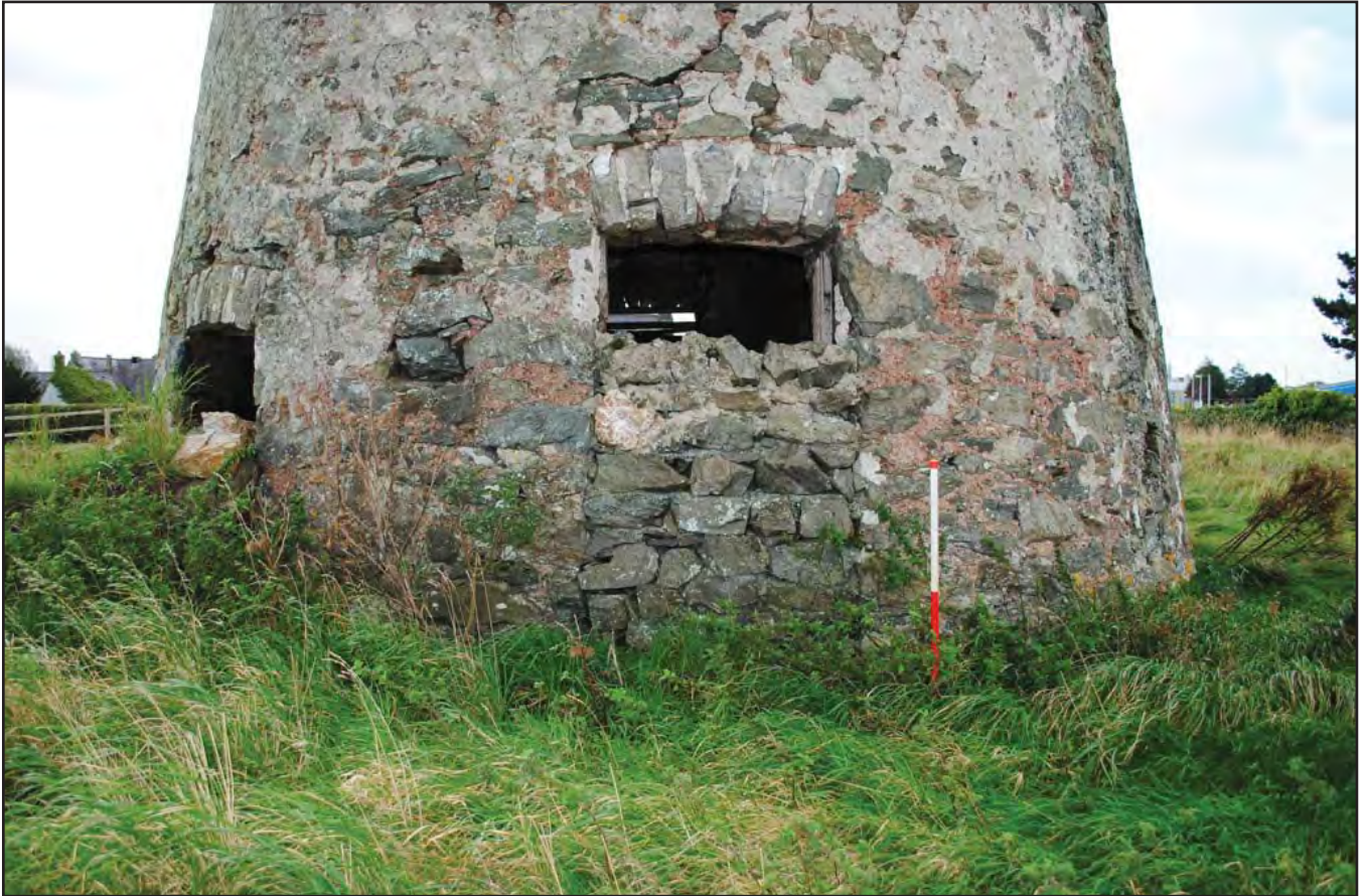
Plate 06: Shot detailing partially blocked doorway & sack hoist chute entrance to the left. Photograph taken from the north
