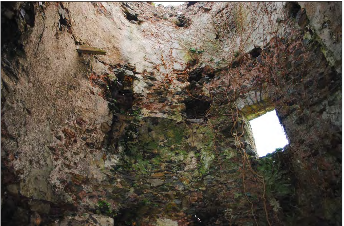
Plate 12: Shot looking upwards showing open window on the 2nd, and blocked window on 3rd floor, as well as roof joist holes. Photograph taken from the south
