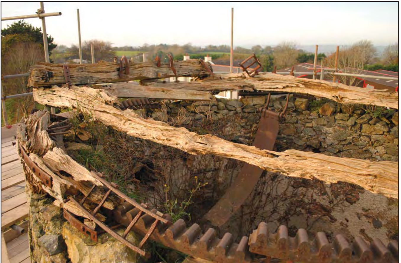
Plate 28: Shot of turning cap showing metal brackets attached to wooden elements of turning cap. Note the iron band which once encircled the brake wheel. Photograph taken from the north west
