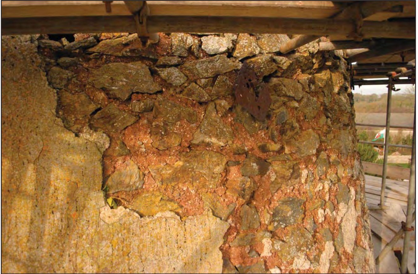
Plate 23: Detailed shot showing original lime render & metal tie plate on the 2nd floor. Photograph taken from the south west
