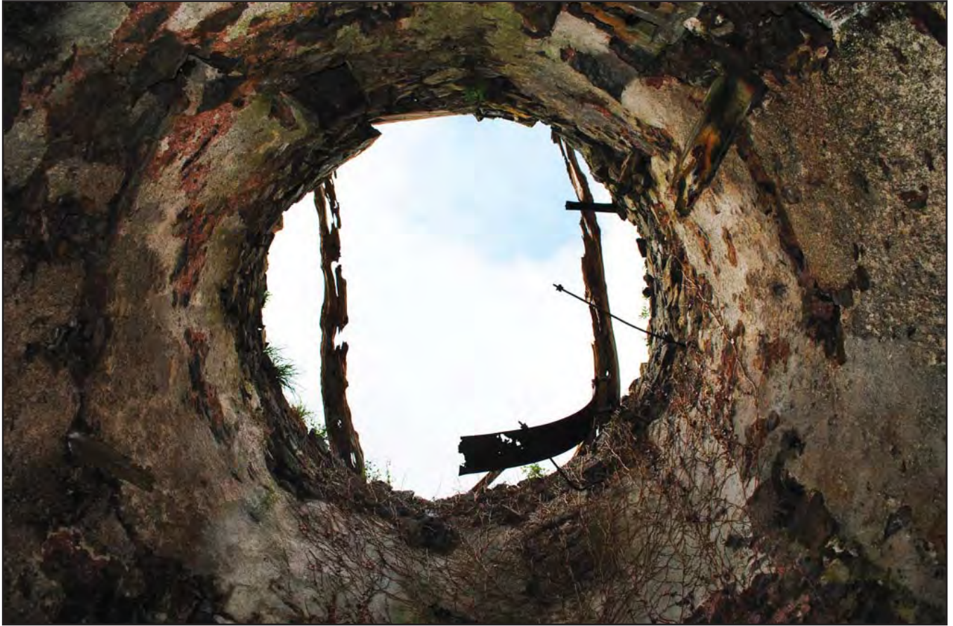
Plate 15: Shot looking directly upwards showing remnants of roof joists & turning cap
