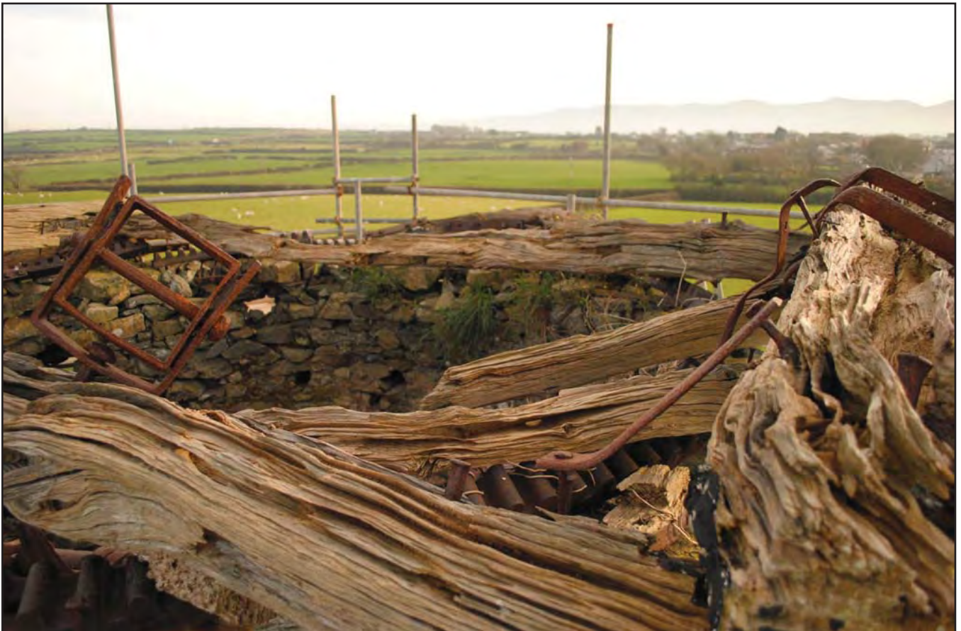
Plate 26: Detailed shot of turning cap revealing serious decay of both wooden and metal elements. Photograph taken from the east
