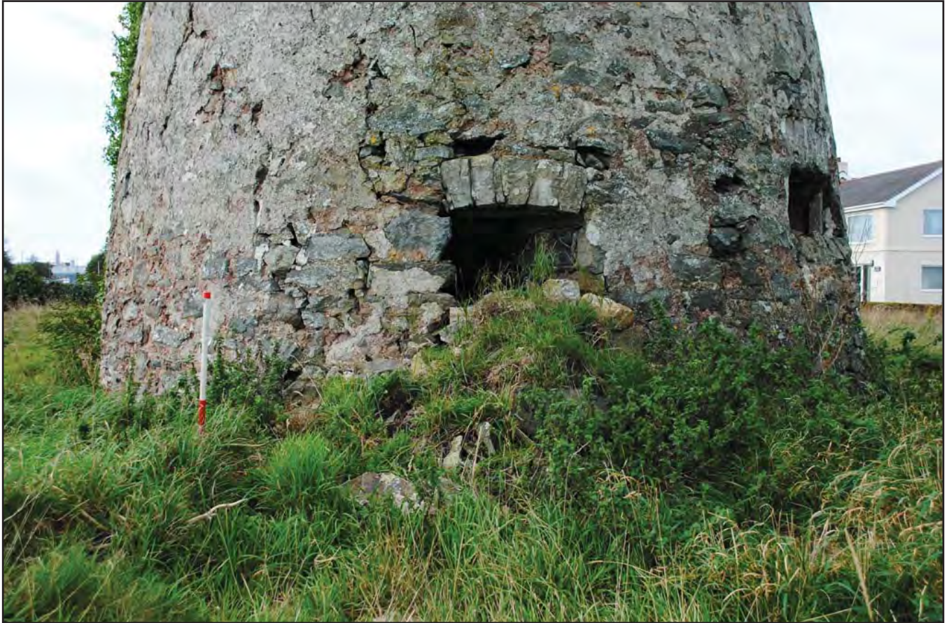
Plate 07: Shot of partially blocked sack hoist chute. Photograph taken from the north east
