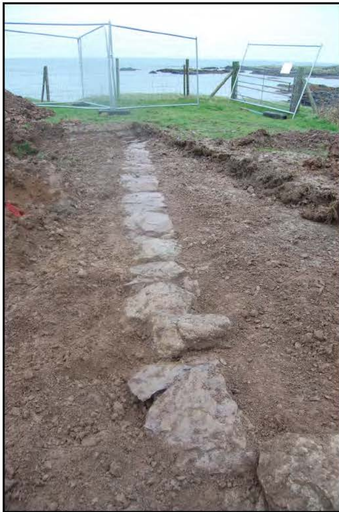
Plate 15: The capstones of a stone built culvert (Feature 19) running nnw-sse across the se end of OT603 (F56).
