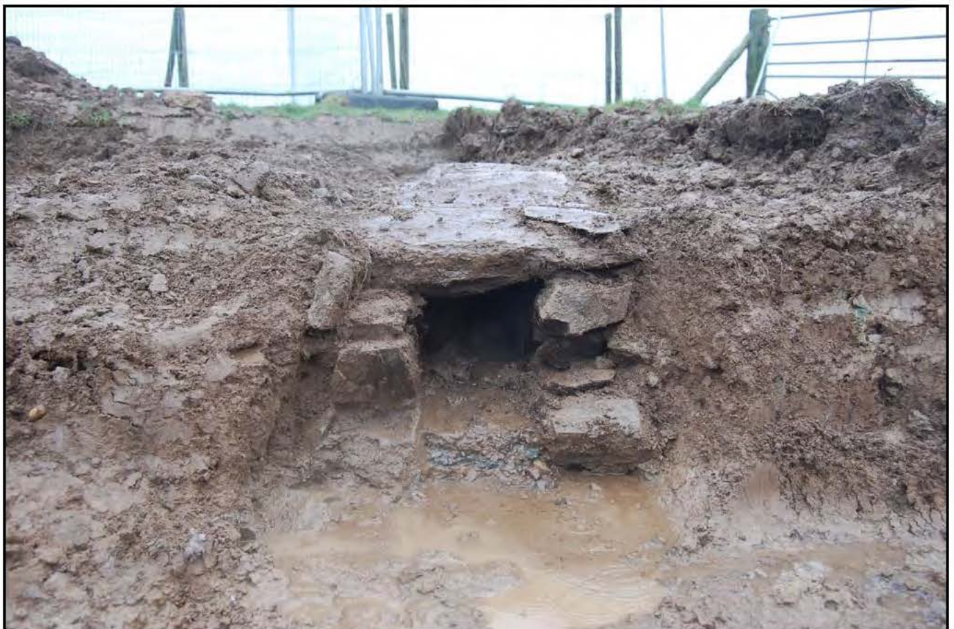
Plate 16: The SSW facing cross section of a stone built culvert (Feature 19).
