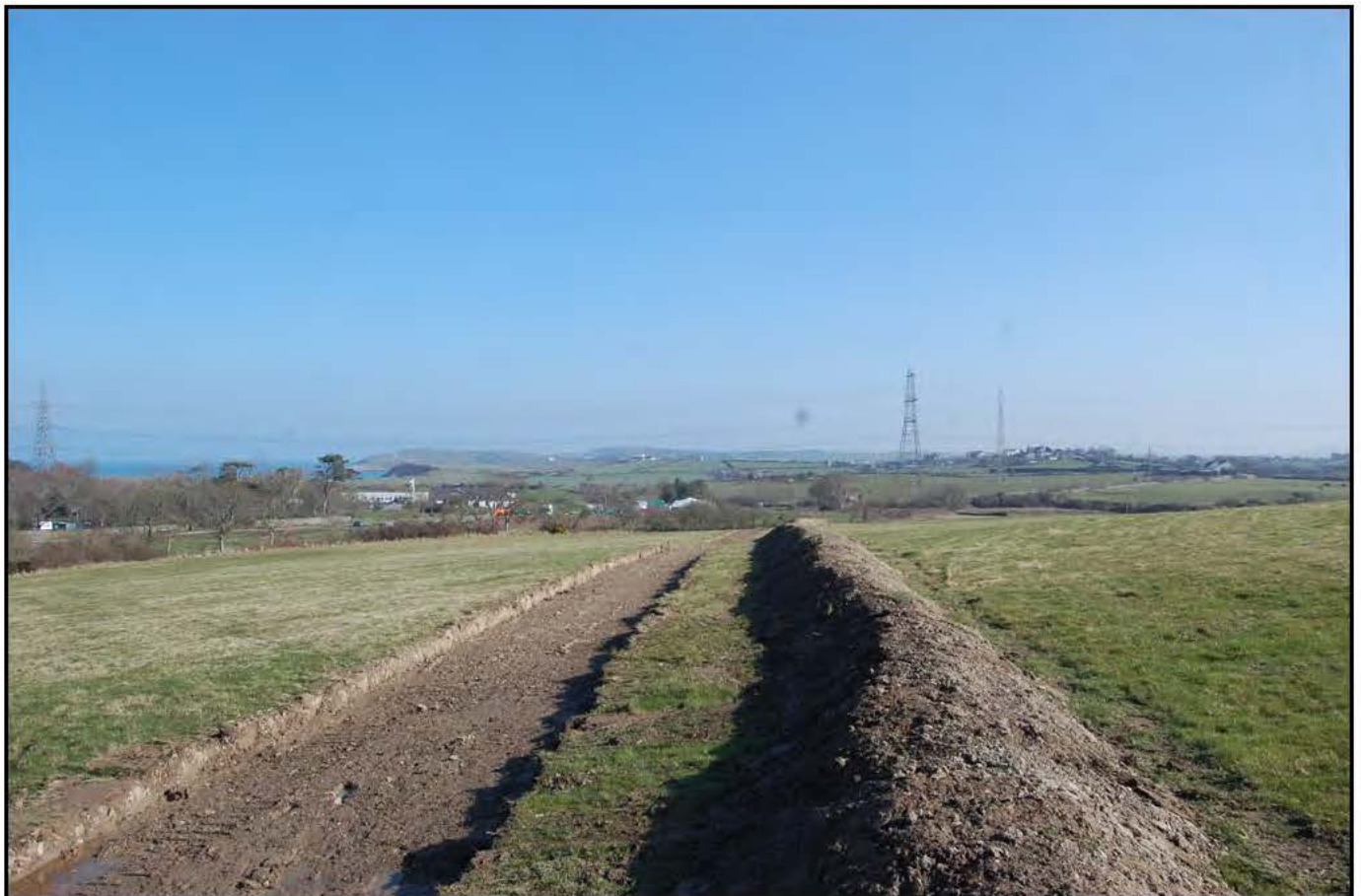
Plate 02: An example of a completed section of haul road trench (F10).
