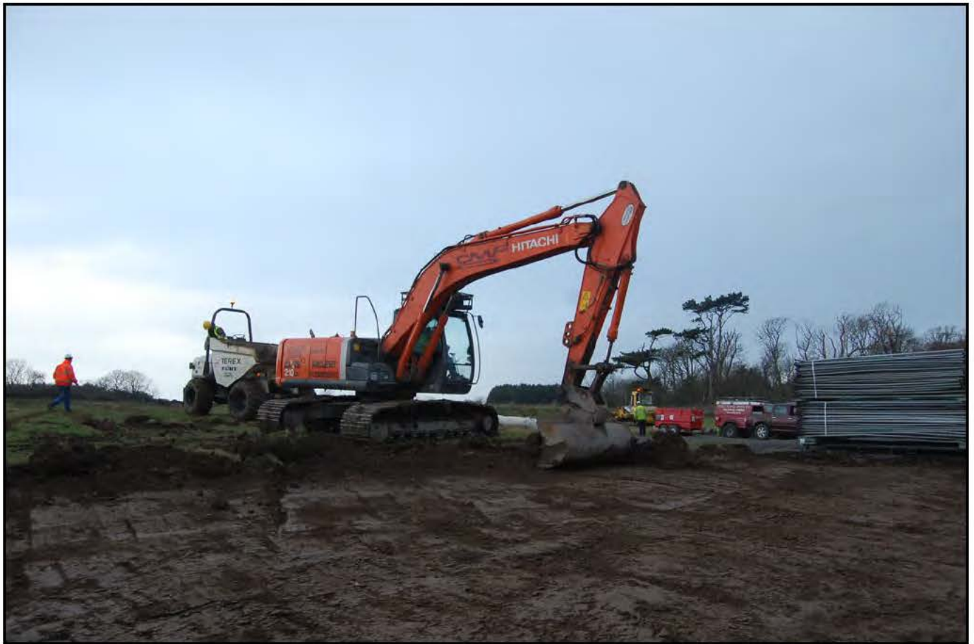
Plate 01: Working shot showing the stripping of the compound area in F9.
