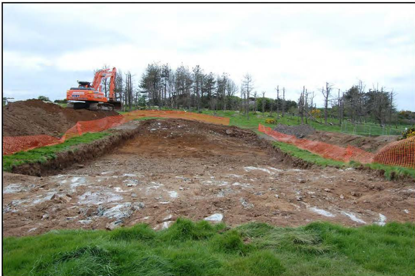
Plate 08: An example of a large Seismic Hazard Observation Trench (OT604B within F56).
