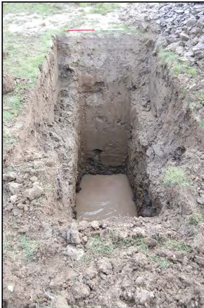
Plate 05: An example of a machine excavated GI Trial Pit (TP 571 within F9) (Scale 1.0m).
