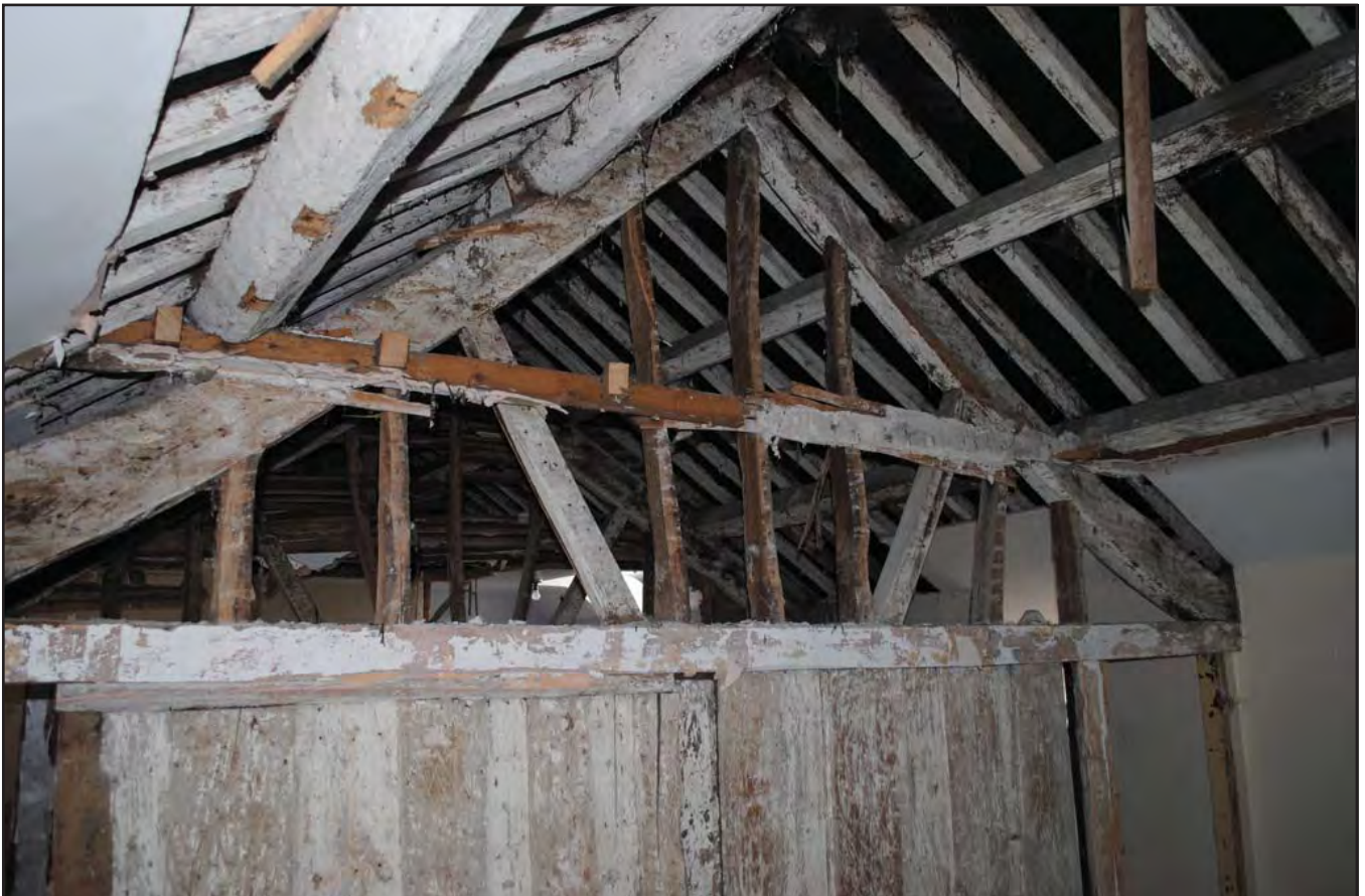
Plate 24: Roof structure and stud panelling between bedrooms 2 & 3. Photograph taken from the south west
