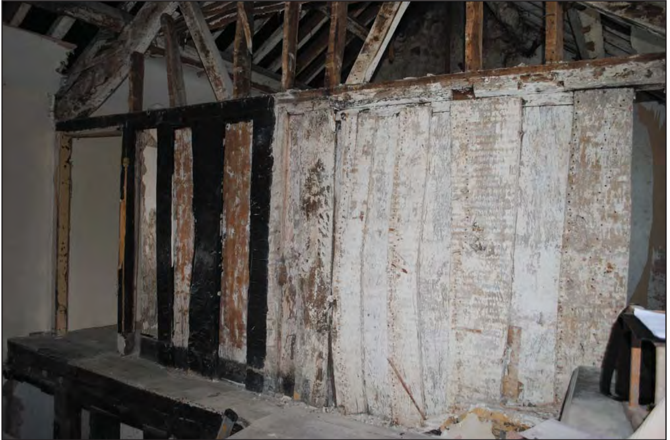
Plate 29: Roof truss and stud panelling between bedrooms 2 & 3. Photograph taken from the north west
