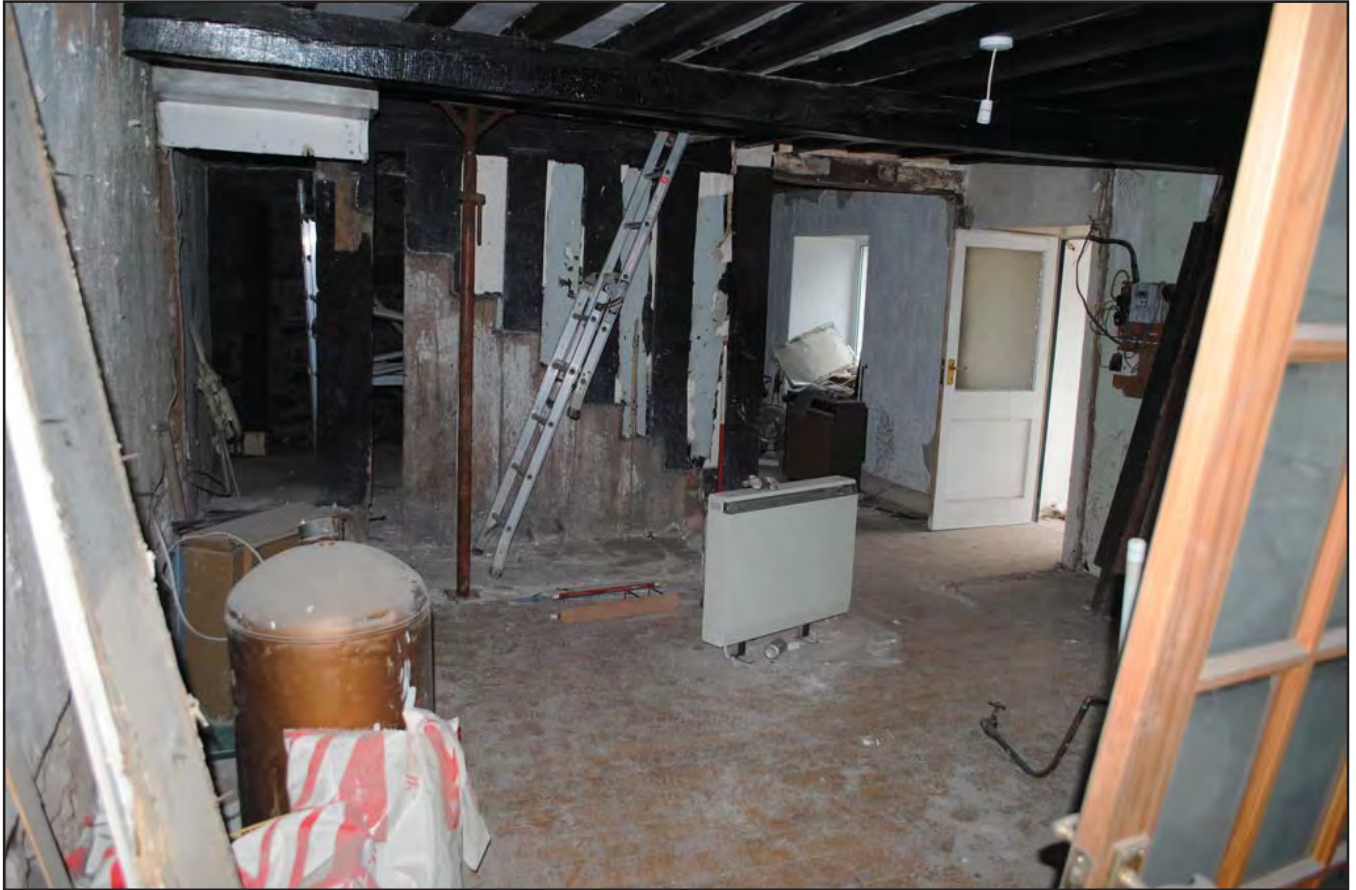
Plate 09: Stud panelling between the main room and parlour. Photograph taken from the north west
