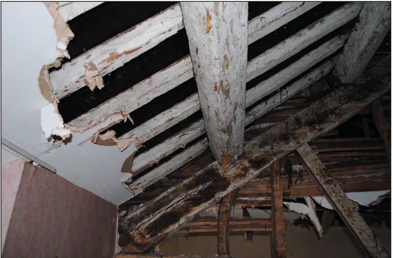
Plate 22: Purlin and Common Rafters in bedroom 2. Photograph taken from the south west
