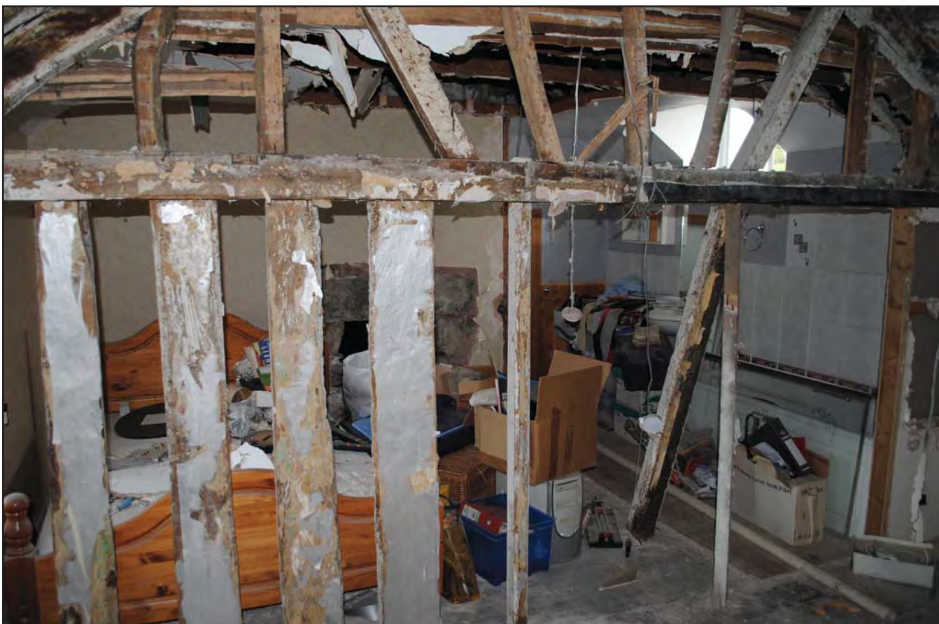
Plate 20: Detail of remnants of stud panelling between bedrooms 2 & 3. Photograph taken from the south
