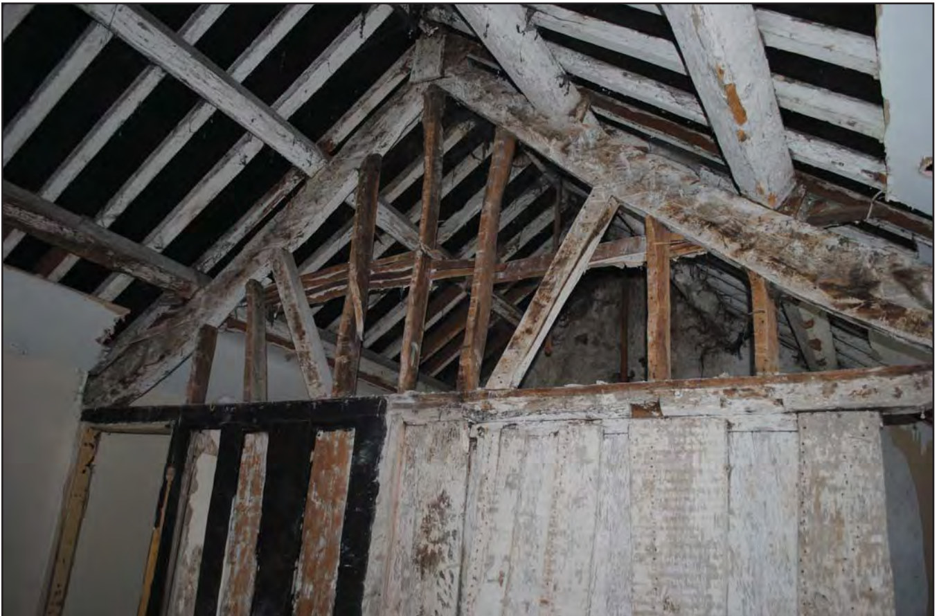
Plate 28: Roof truss showing raked braces between bedrooms 2 & 3. Photograph taken from the north
