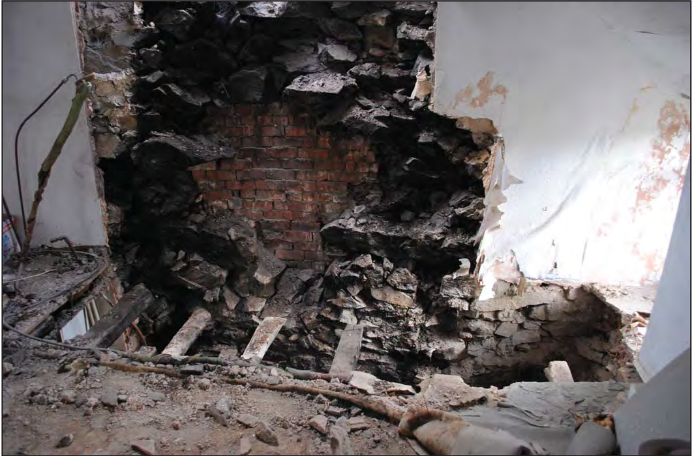
Plate 33: Evidence of fire destruction and removed fireplace in bedroom 1. Photograph taken from the south east
