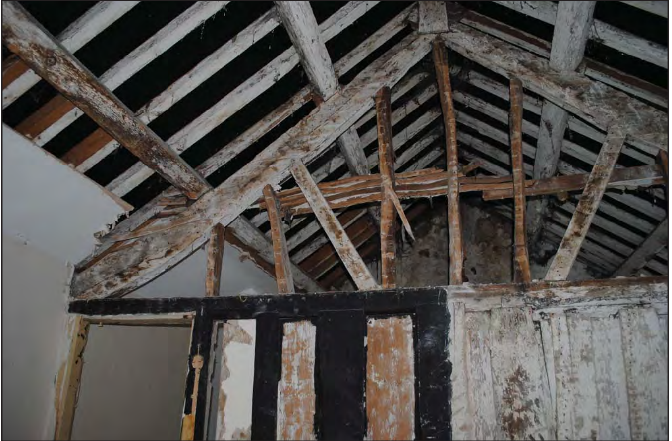
Plate 27: Roof truss and stud panelling between bedrooms 2 & 3. Photograph taken from the north west
