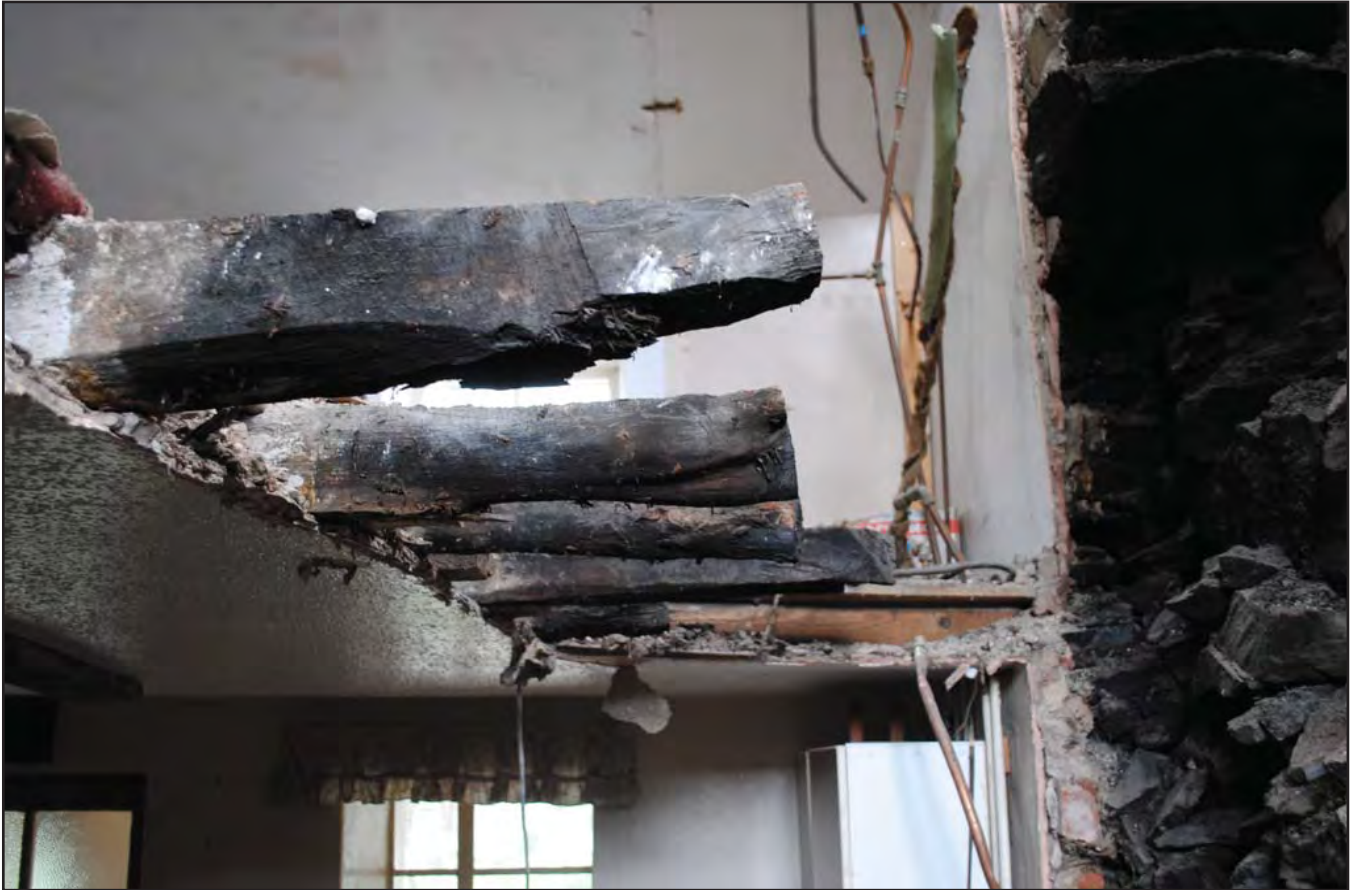
Plate 08: Burnt floor joists in kitchen extension
