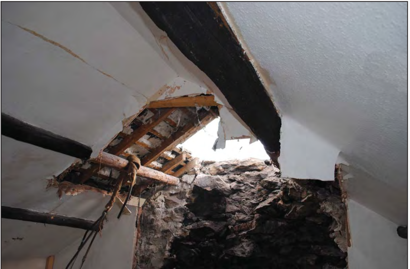
Plate 32: Open roof structure with chimney removed in bedroom 1. Photograph taken from the east
