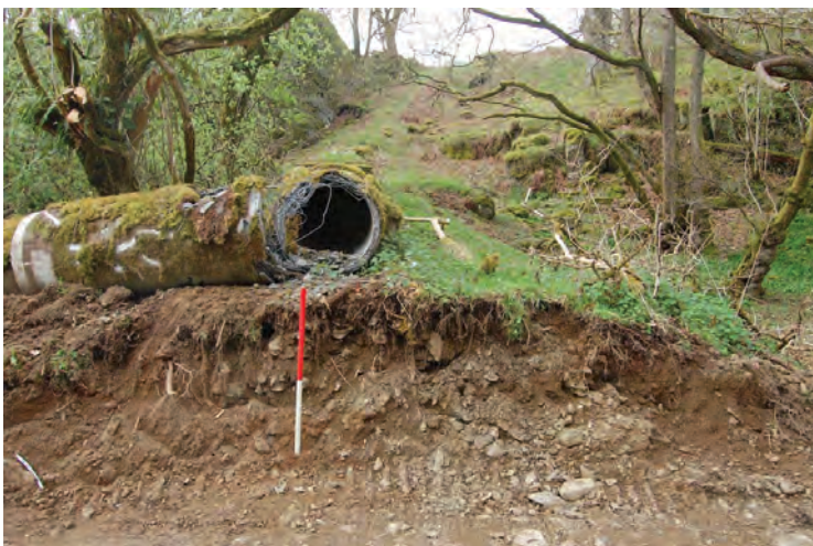
Plate 11. Disused surge pipe (F90) broken through to allow access to borehole 15
