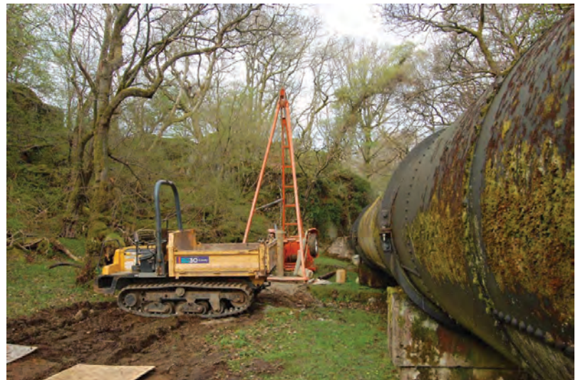
Plate 10. Cable percussive borehole rig in place on BH 15
