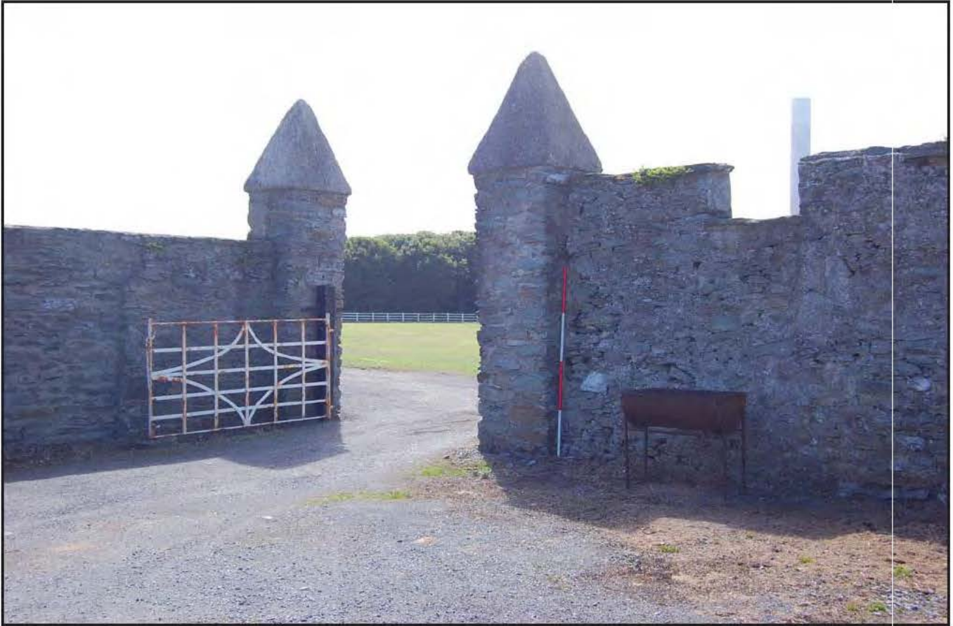
Plate 05: Gateway into Penrhos Home Farm (15). Photograph taken from the north west
