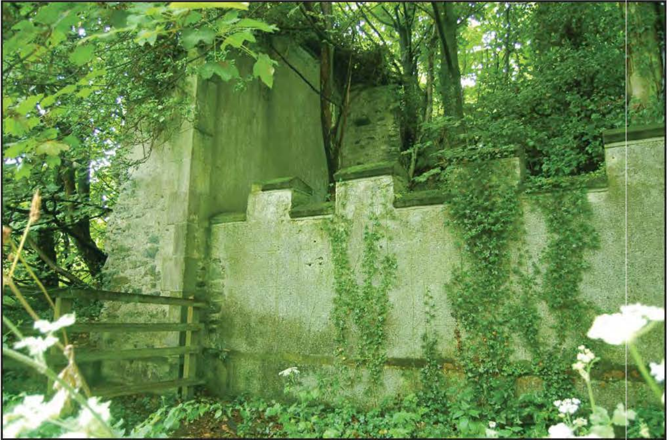
Plate 11: Remnants of rear elevation of Penrhos House. Photograph taken from the south east
