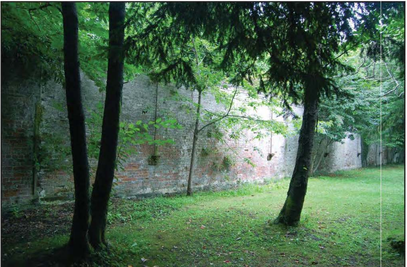
Plate 12: Boundary wall of kitchen garden of Penrhos House. Photograph taken from the south west
