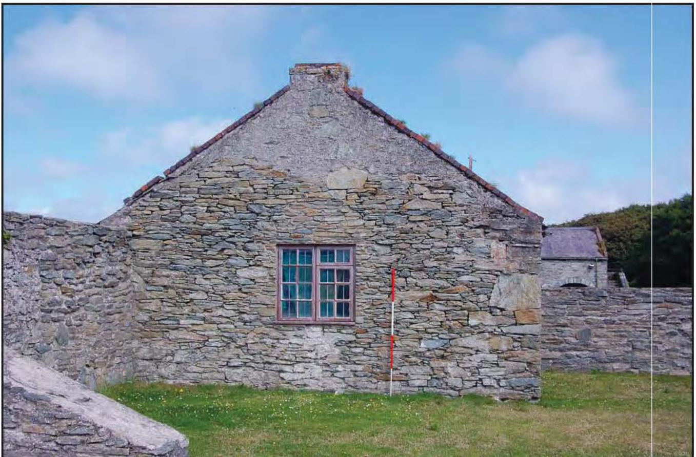
Plate 04: Penrhos Home Farm out building (15). Photograph taken from the west
