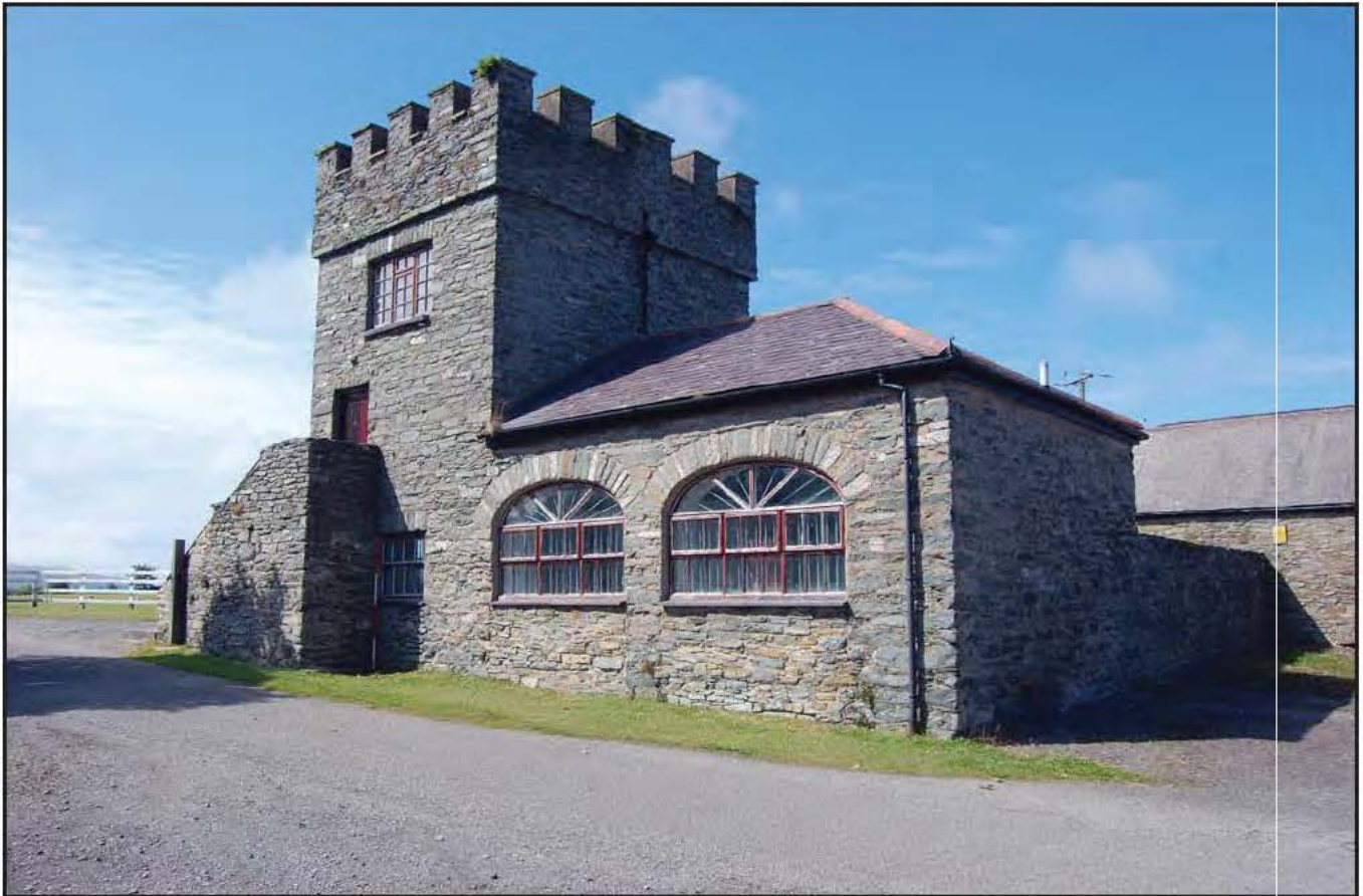
Plate 03: Bailiffs Tower Penrhos Home Farm (15). Photograph taken from the south east
