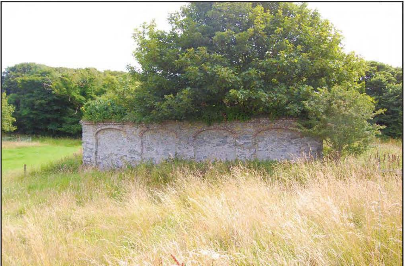
Plate 02: A Tre-gôf farm out building (13). Photograph taken from the north west
