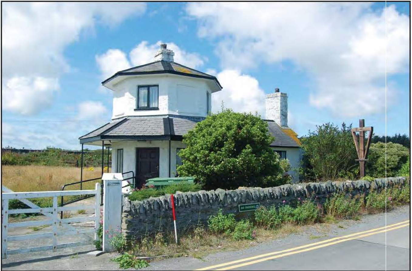
Plate 19: Penrhos Toll House (06). Photograph taken from the east
