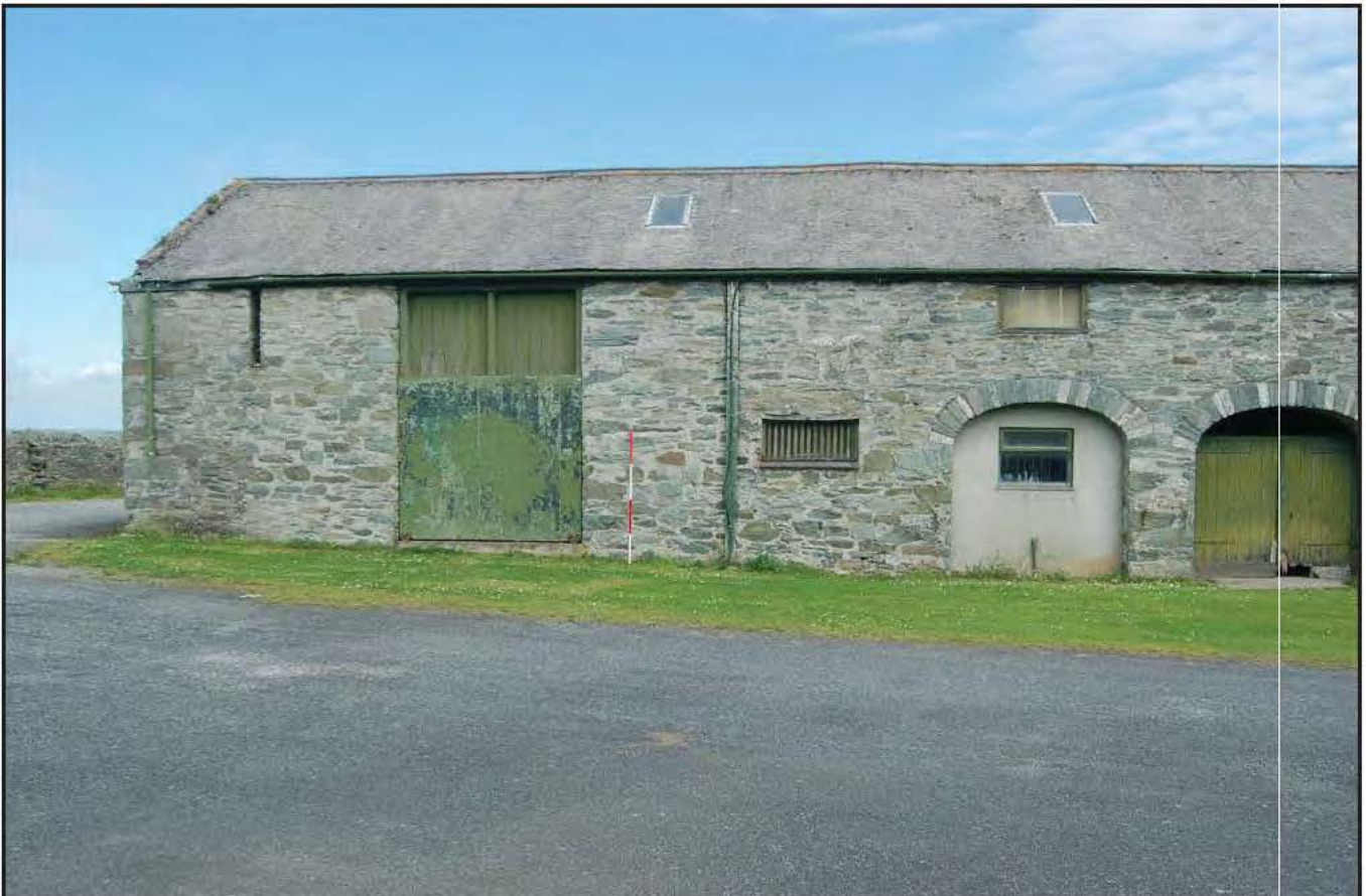
Plate 08: Penrhos Home Farm out building (15). Photograph taken from the south east
