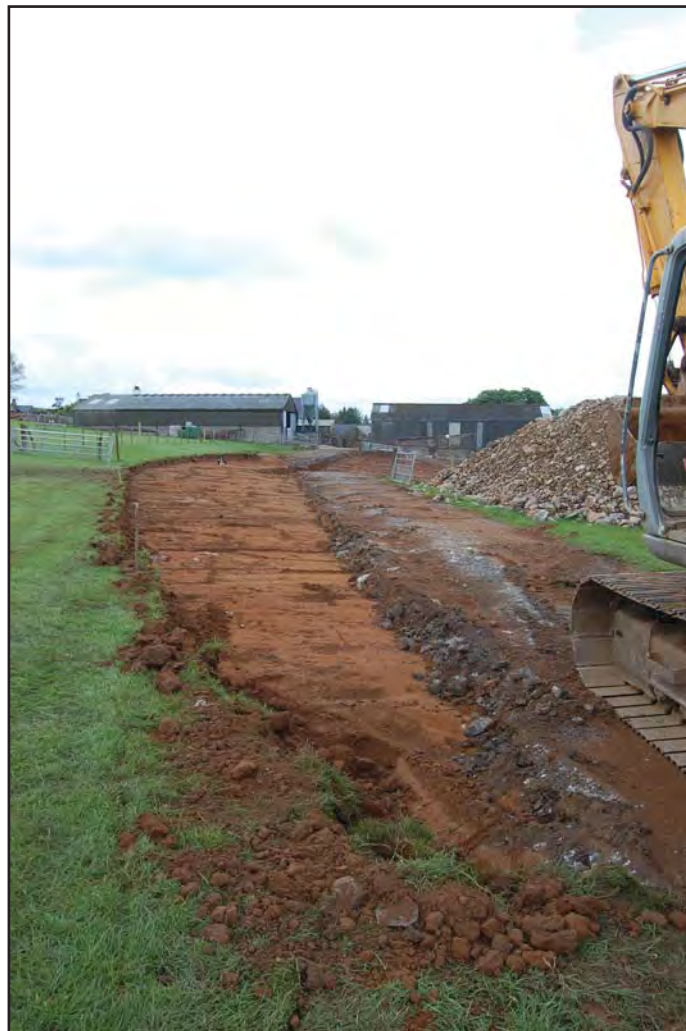
Plate 9: Post-excitation shot of the foundation trench for the replacement track (view from the south-west).
