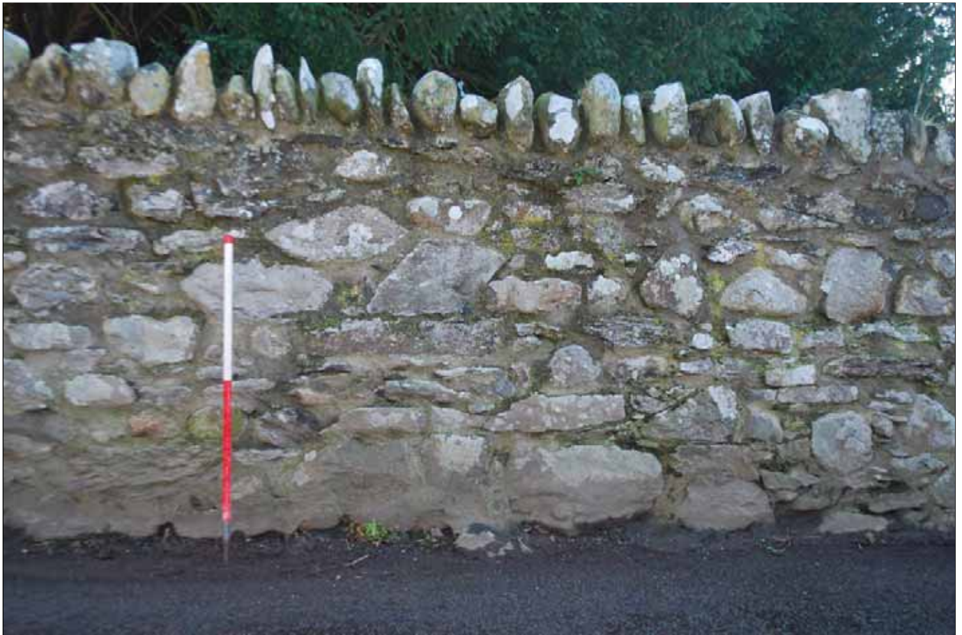
Plate 15 The churchyard wall from the west, showing building style with larger field stones at the base and cock and hen capping. Scale 1m with 50cm divisions
