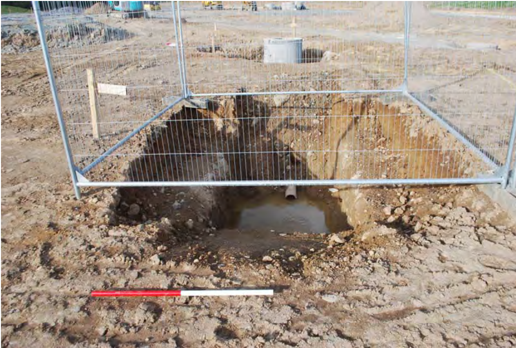
Plate 9 Excavation for service manhole during construction phase
