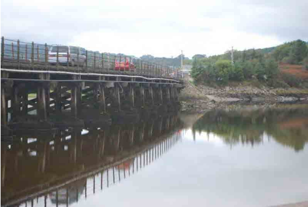
Plate 9 Pont Briwet at Traeth Bach level from the south south east showing wooden piers
