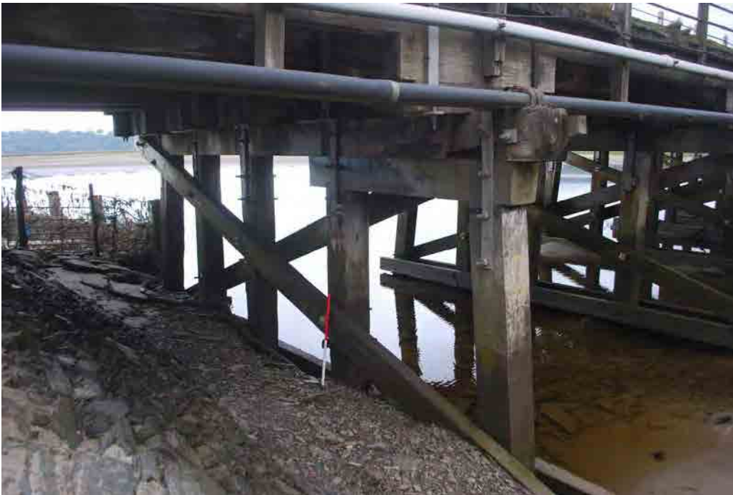
Plate 8 Detail of Braced timber piles and supports on Pont Briwet. View from east south east. Scale 1m
