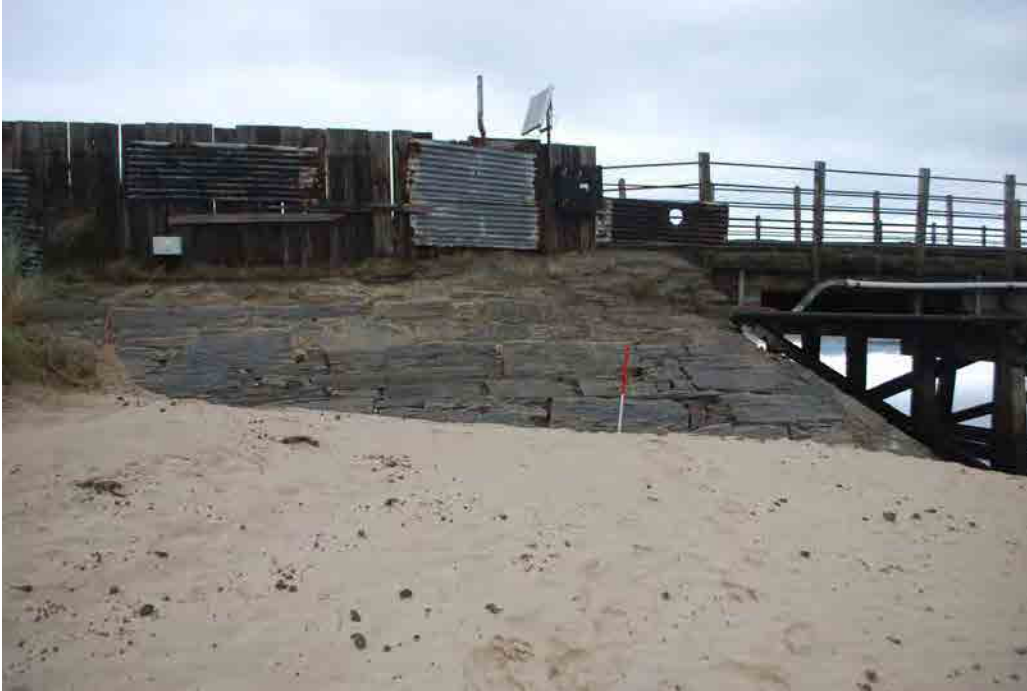
Plate 7 Slate abutment at the southern end of Pont Briwet, from the south east. Scale 1m
