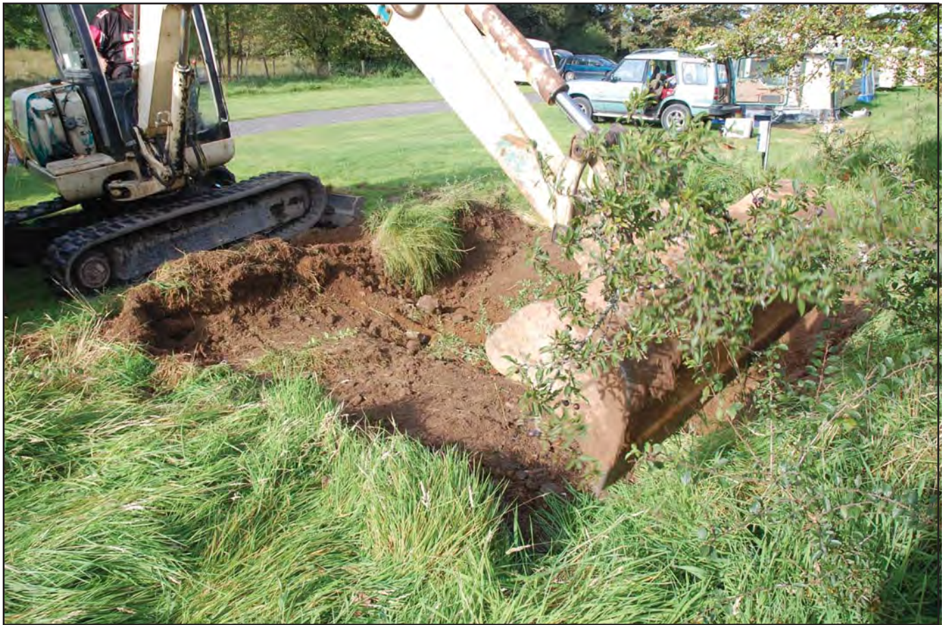
Plate 03 - Excavation of trench 1. View from the north-east.
