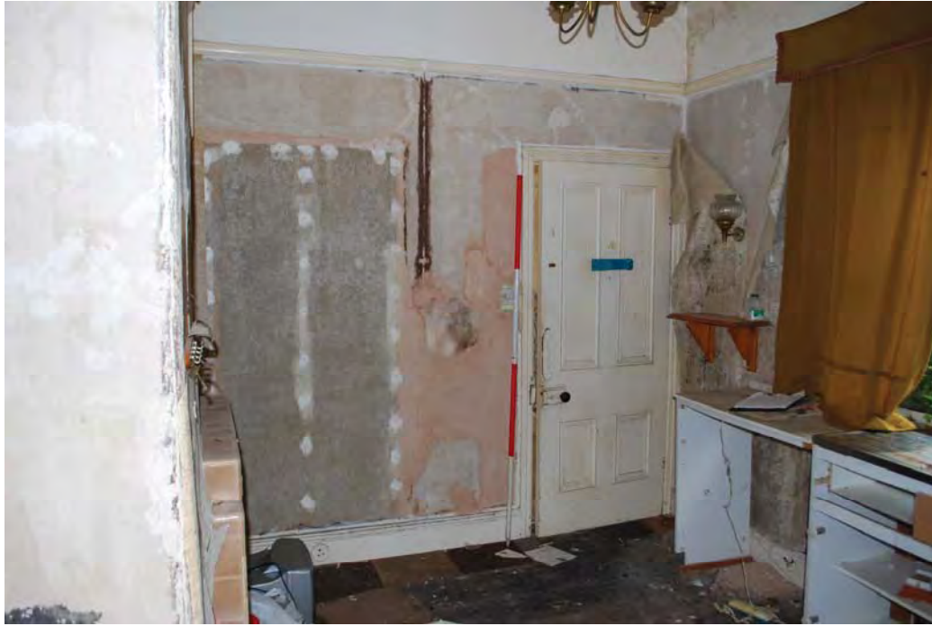
Plate 17 Room 1, showing panelled door to room 4. Scale 2m
