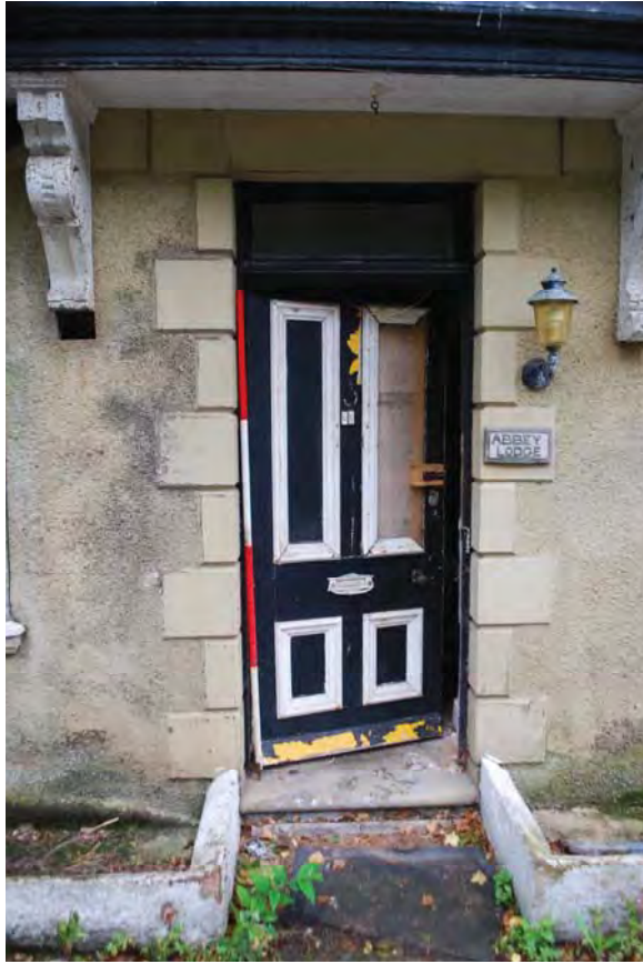
Plate 15 Abbey Lodge front door. Scale 2m
