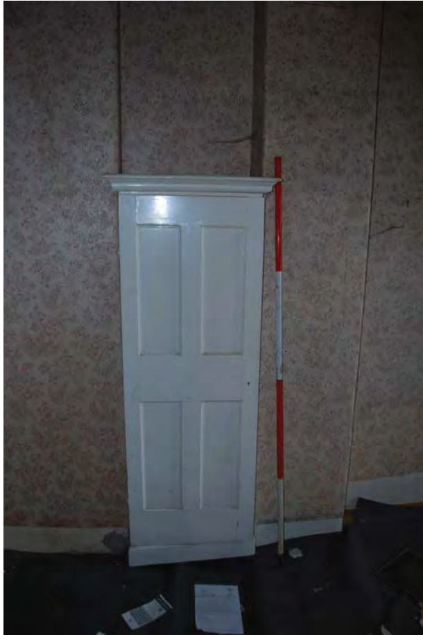
Plate 23 Cupboard in room 5. Scale 2m
