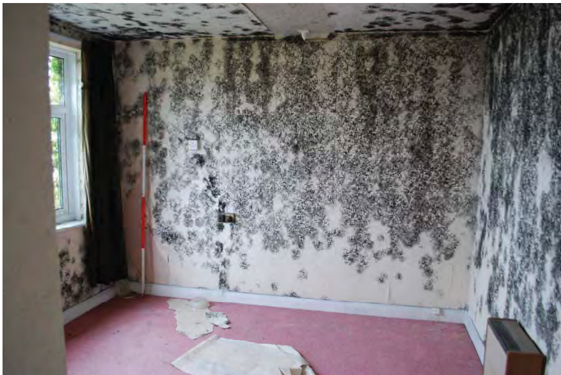
Plate 28 Room 9. Scale 2m
