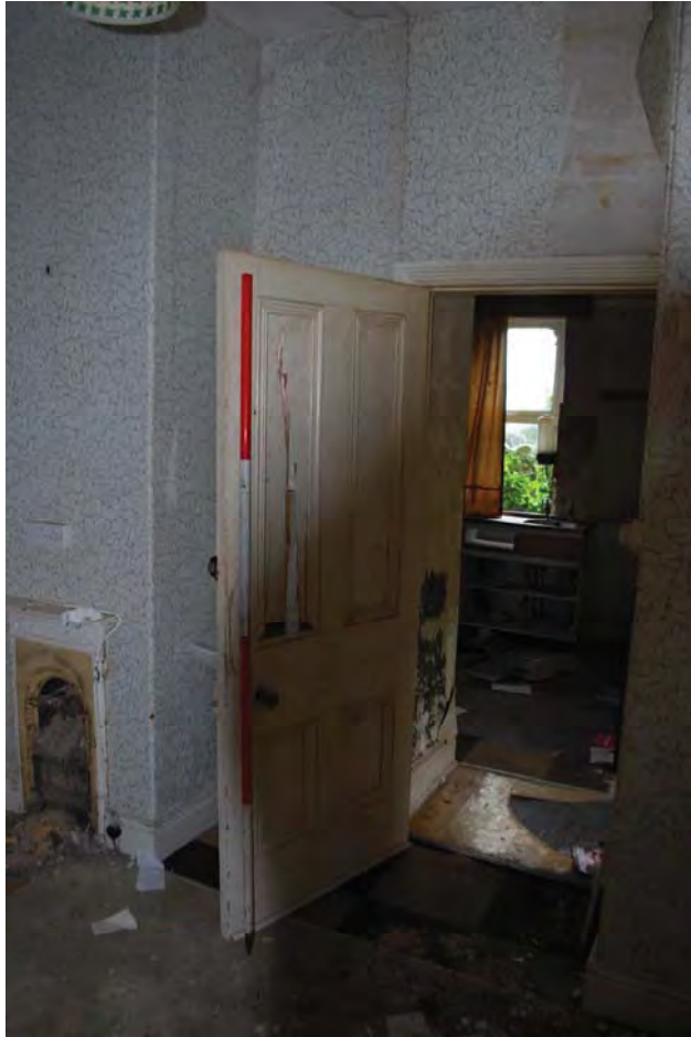
Plate 19 Panelled door between rooms 1 and 2. Scale 2m
