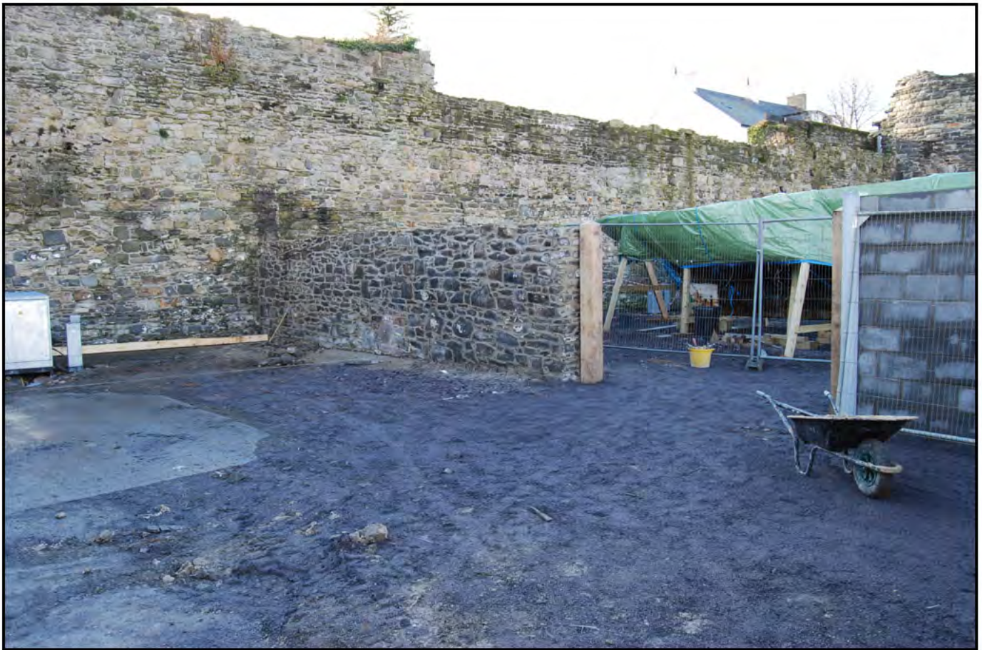
Plate 01: Zone 1/Yard 1 (PRN 30451): view west of Zone 01 during repointing of former Cross Wall A (cf. Fig. 02) and construction of a block wall joining Cross Wall A to Enclosure Wall A (not visible). A new entrance linking Zones 01 and 02 is also visible. The Nobby boat is also visible in the background (Zone 02), supported on wooden posts and covered with tarpaulin. Zone 01 was the former location of Buildings 01 and 18 (see appendix I for PRN numbers).
