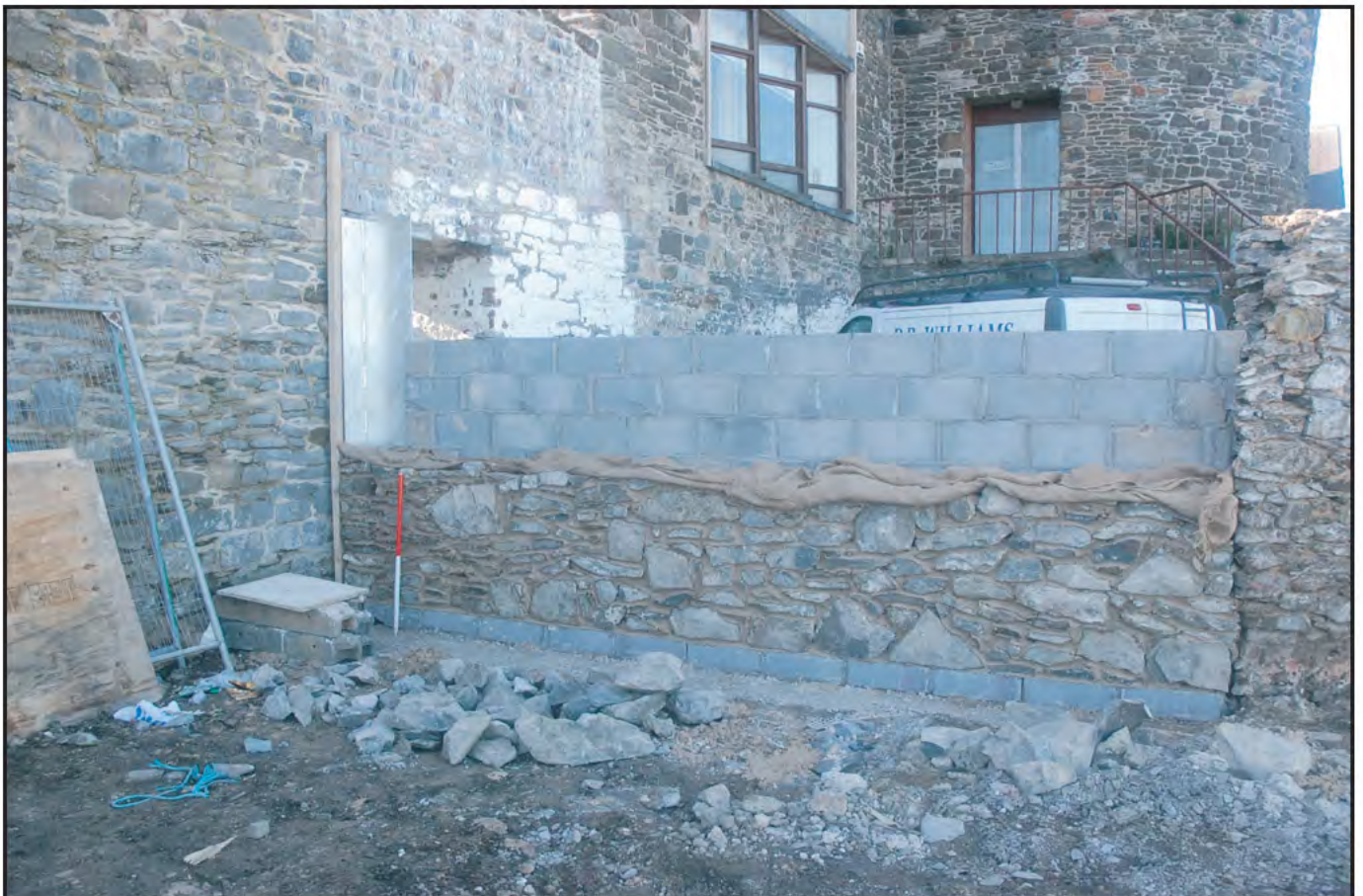
Plate 12: Zone 3/Yards 5 (PRN 30469) & 6 (PRN 30474): view northwest of salvaged stone wall during construction, designed to replace the timber screen visible in Plate 11. Scale: 1 x 1.0m.
