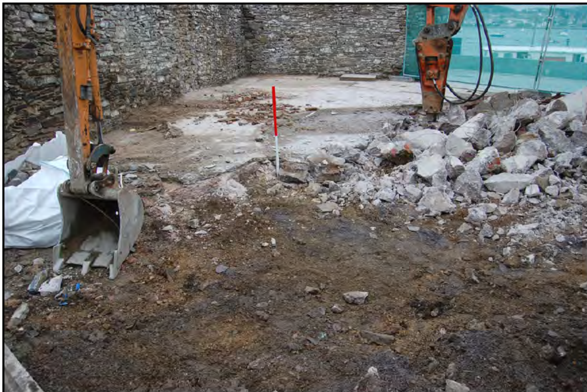
Plate 07: Zone 3/Yards 5 (PRN 30469) & 6 (PRN 30474): excavation of the former ground levels of Buildings 7 (PRN 30475) and 8 (PRN 30476): both floors were built from concrete atop redundant (brick) building material sub-base. Beneath the sub-base was the construction layer for the quayside previously identified during the service trench installation. Zone 03 became the location for the new interpretation area. Scale: 1 x 1.0m
