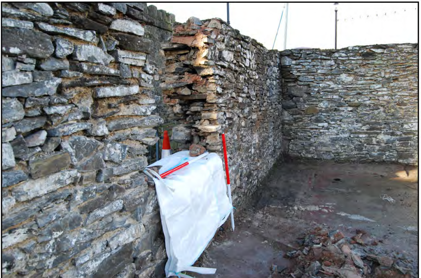
Plate 10: Zone 3/Yards 5 (PRN 30469) & 6 (PRN 30474): Enclosure Wall A repair; former aperture for Building 07 (PRN 30475), detailing wall thickness and construction (0.40m thick). Scale (2 x 1.0m)
