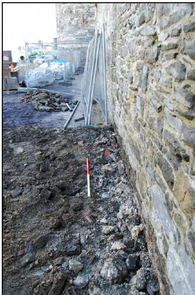
Plate 08: Zone 3/Yards 5 (PRN 30469) & 6 (PRN 30474): View southeast of after removal of Building 08 (PRN 30476) floor surface. The foundation footing for Building 08 can be seen running parallel to the town wall. This footing had originally been identified during the initial watching brief (GAT Report 815). Scale: 1 x 1.0m
