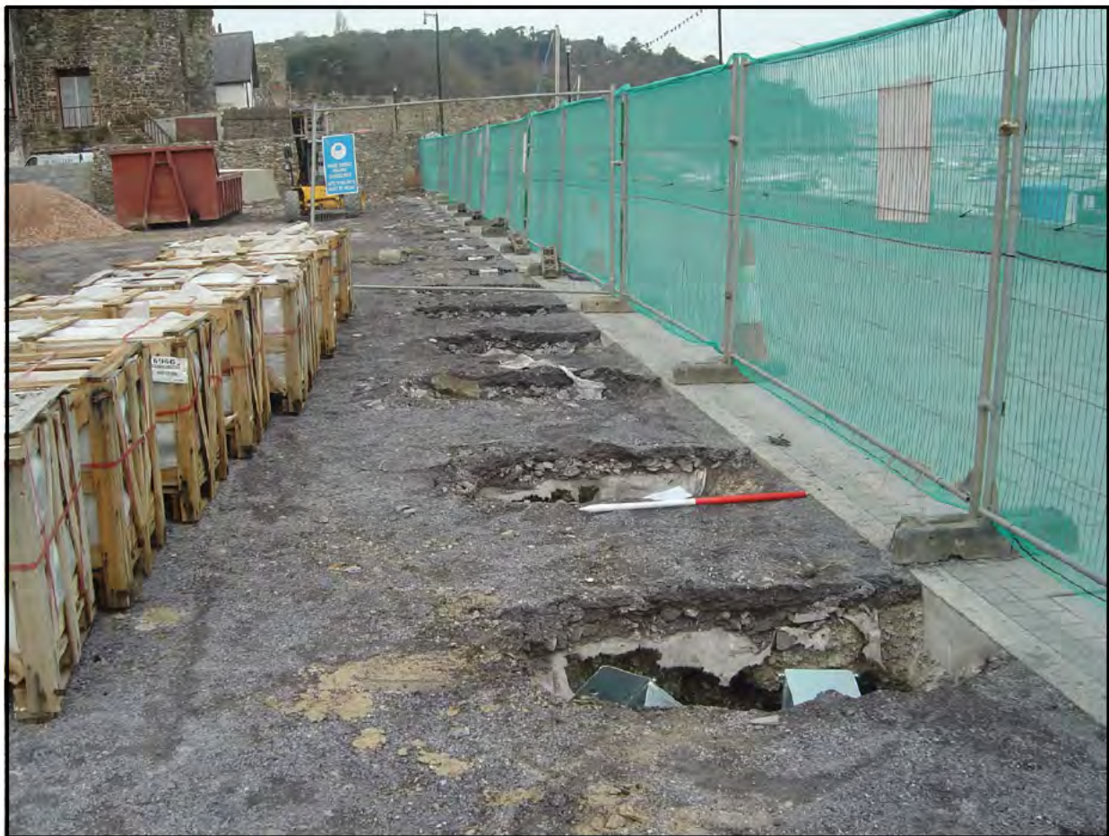
Plate 03: Zone 2/Yards 2 (PRN 30454), 3 (PRN 30457) & 4 (PRN 30463): view northwest of oak bollard foundation cuts (depth 0.75m). The oak bollards were set 2.0m apart and to be connected by chain links that segregate the paved road and the eventspace in Zone 02. A total of 31 foundation cuts were made. (Scale 1 x 1.0m)
