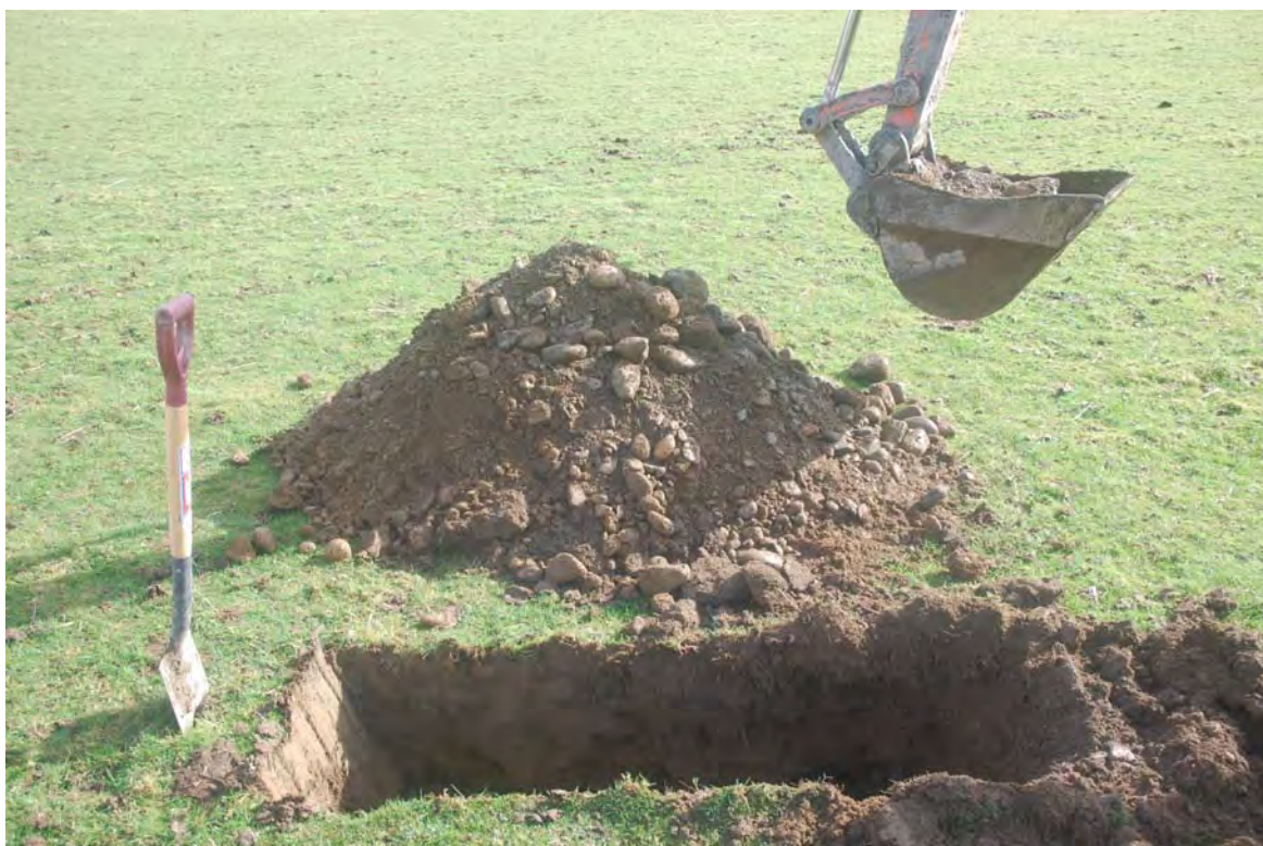
Plate 2 Test Pit 11 under excavation
