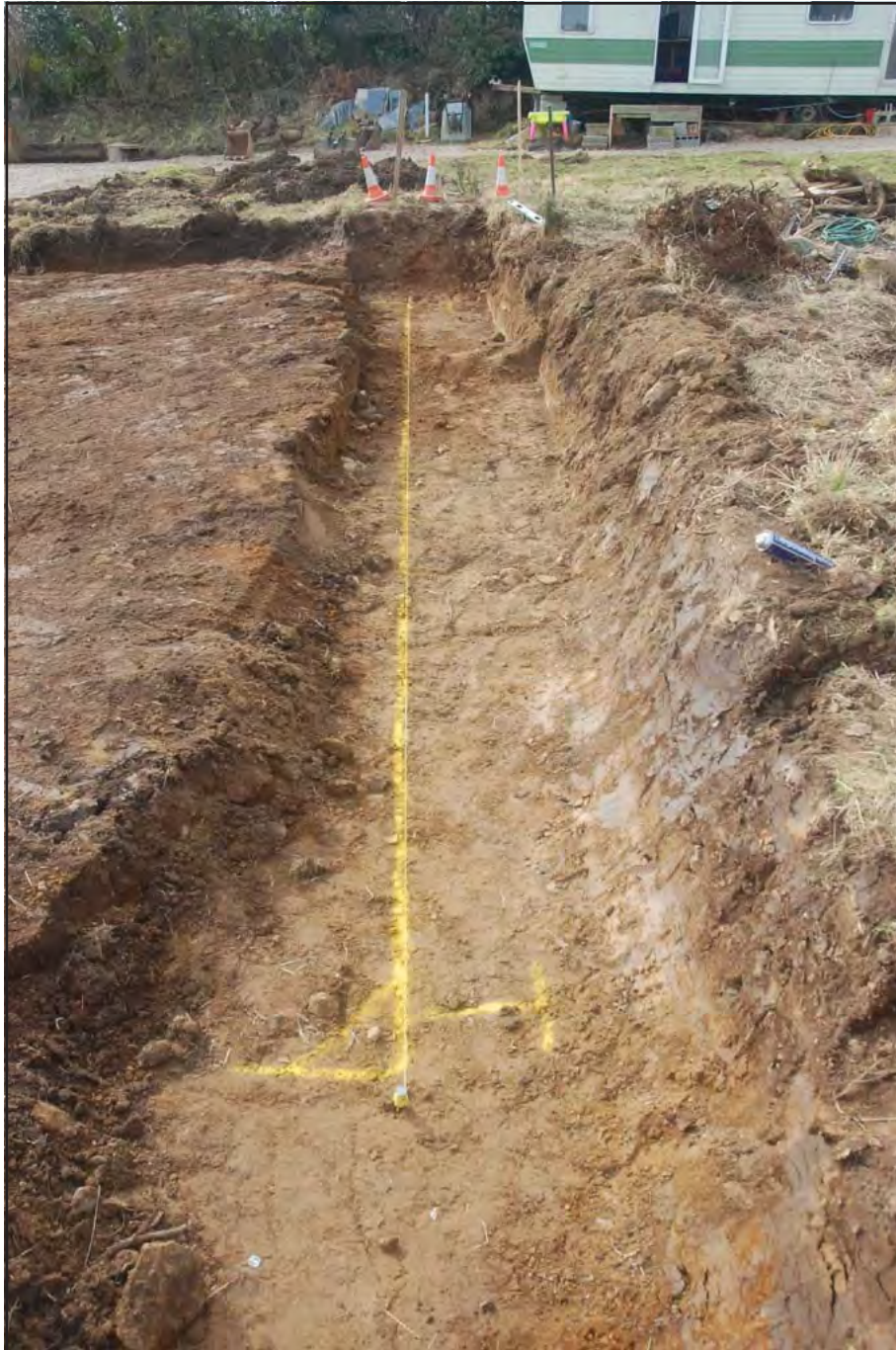
Plate 05: view south of groundworks area detailing limit of excavation (0.75m below ground level) and orientation of footings for the new development. The topsoil was removed with the JCB and had a depth of between 0.30m and 0.40m. The natural deposits lay directly below the topsoil and was excavated to a maximum depth of 0.28m over the total extent of the trench
