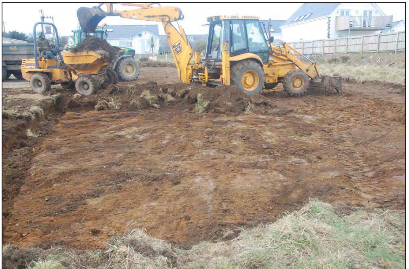
Plate 02: view northwest of groundworks during removal of topsoil and exposure of glacial deposits. The topsoil was removed with the JCB and had a depth of between 0.30m and 0.40m. The glacial deposits lay directly below the topsoil and was excavated to a maximum depth of 0.28m over the total extent of the trench. The surface geology was visible as a light orange-yellow sand-clay containing a moderate amount of cobble sized stone.
