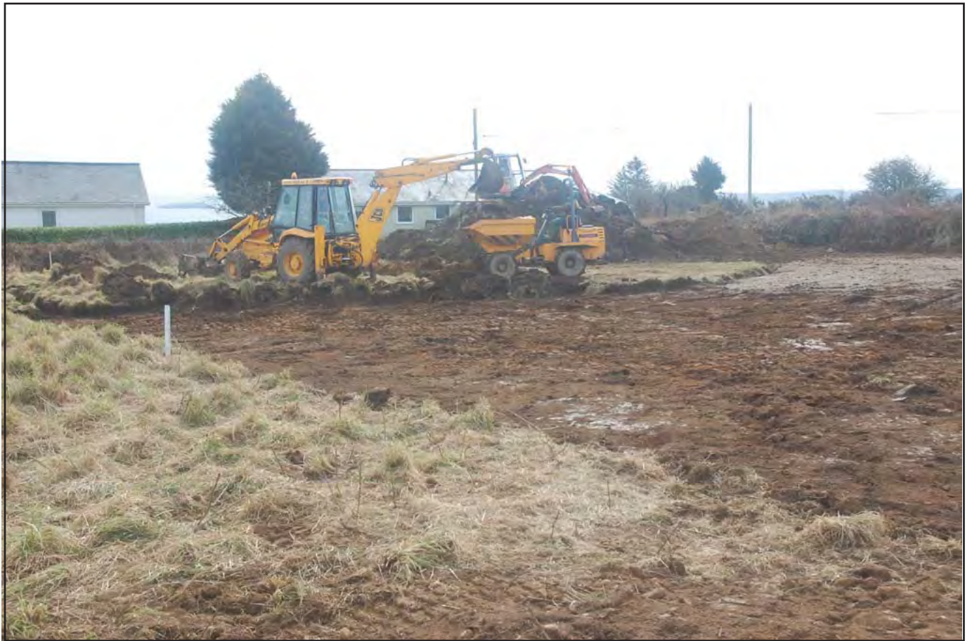
Plate 01: view north of groundworks area during initial strip. Total area groundworks area measured 372m 2 . The topsoil was removed with the JCB and had a depth of between 0.30m and 0.40m. The glacial deposits lay directly below the topsoil and was excavated to a maximum depth of 0.28m over the total extent of the trench, in the presence of the GAT archaeologist.
