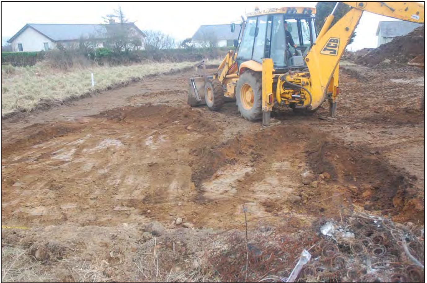
Plate 03: view northeast of the site during initial groundworks. The topsoil was removed with the JCB and had a depth of between 0.30m and 0.40m. The glacial deposits lay directly below the topsoil and was excavated to a maximum depth of 0.28m over the total extent of the trench. The surface geology was visible as a light orange-yellow sand-clay containing a moderate amount of cobble sized stone.
